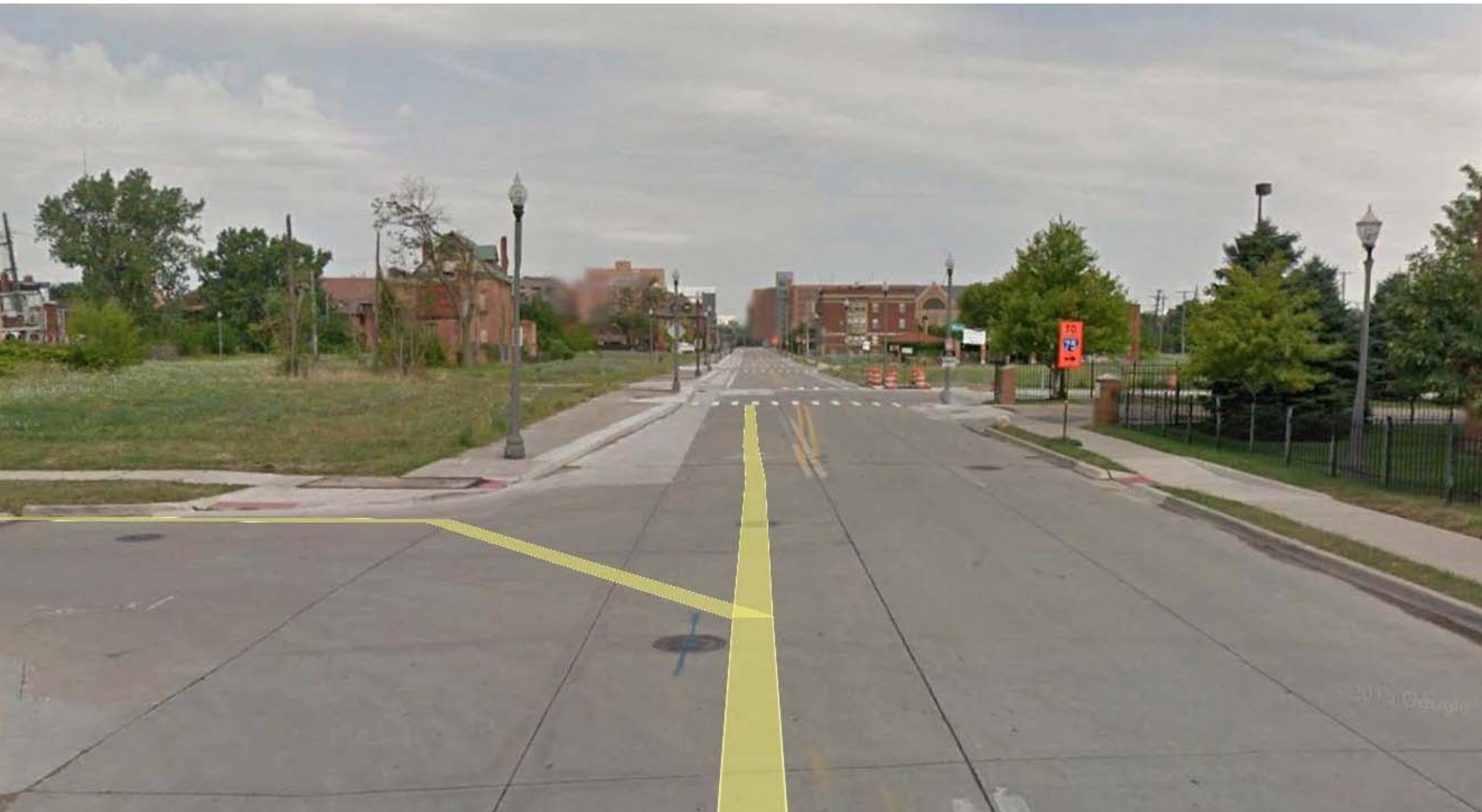
Looking northwest on Brush Street from Edmund Place.
