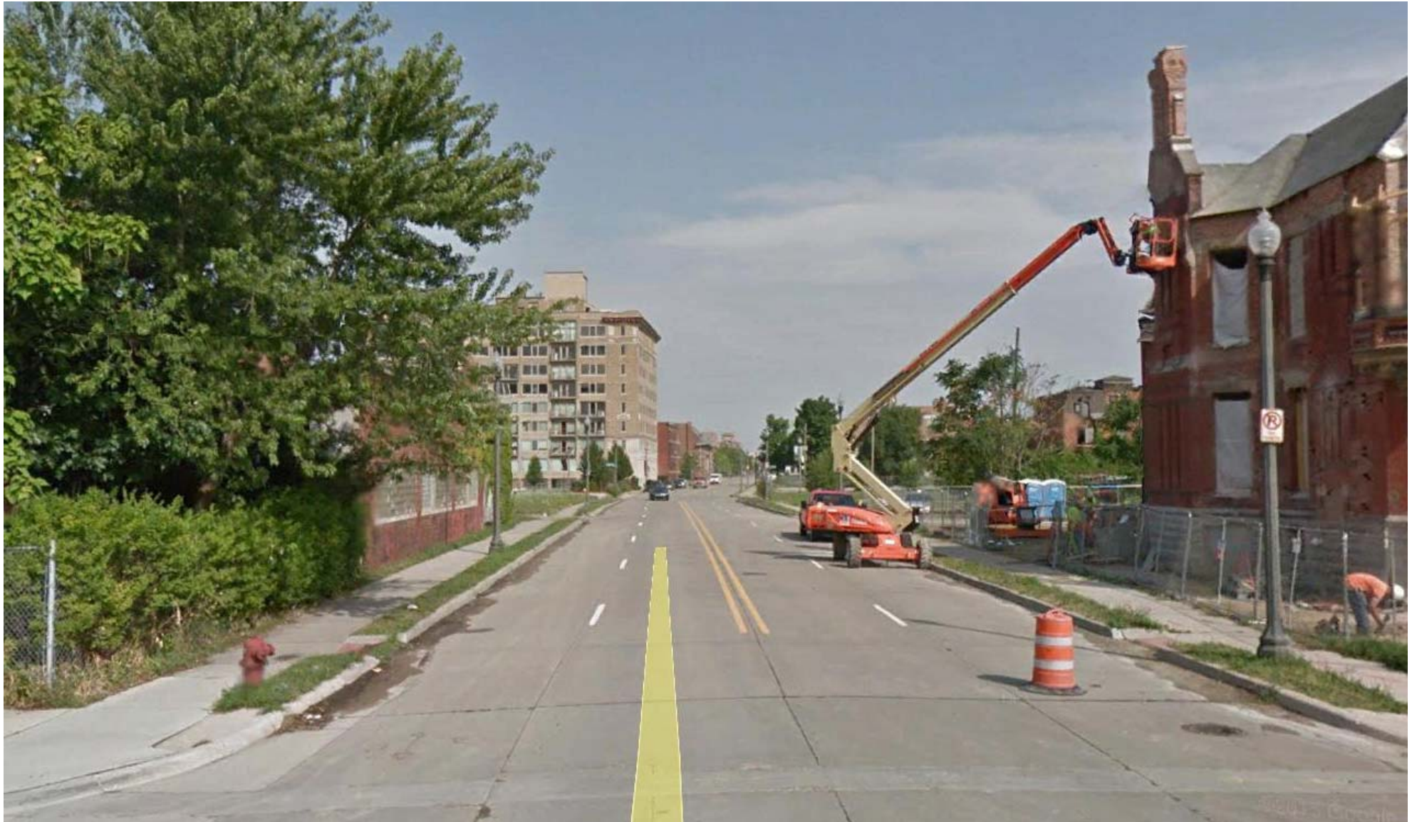
Looking northwest on John R Street from Alfred Street.
