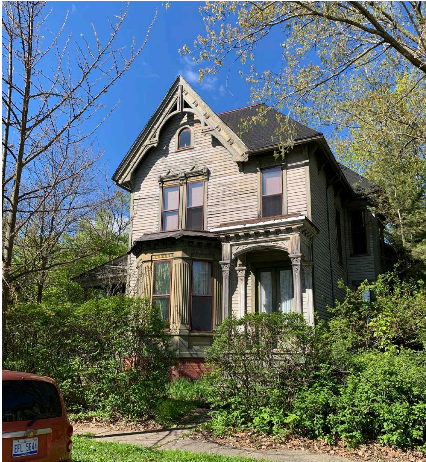
4147 LINCOLN STREET - IN HISTORIC DISTRICT
