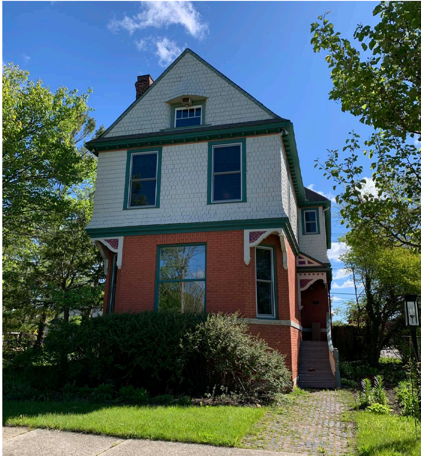
4104 LINCOLN STREET - IN HISTORIC DISTRICT
