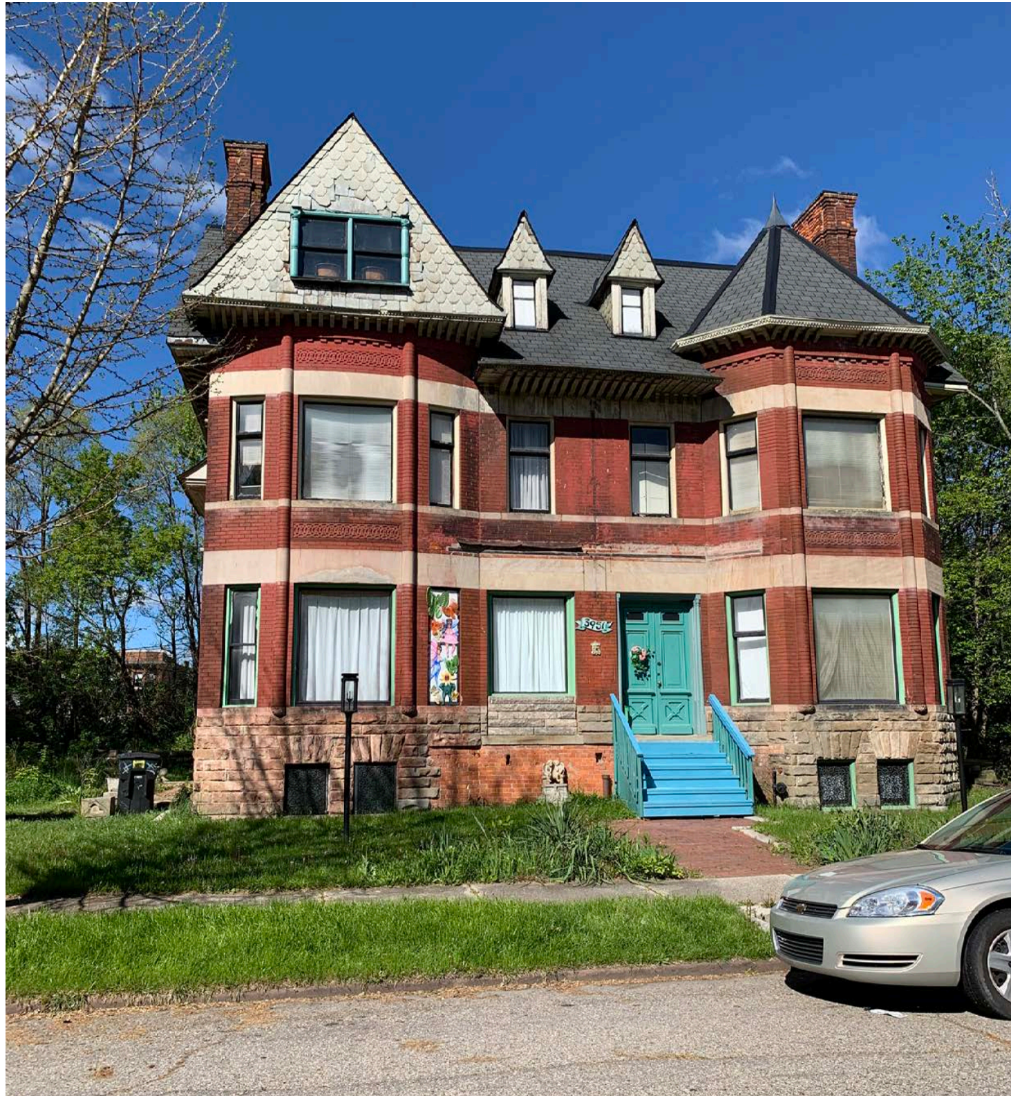
3962 LINCOLN STREET - IN HISTORIC DISTRICT
