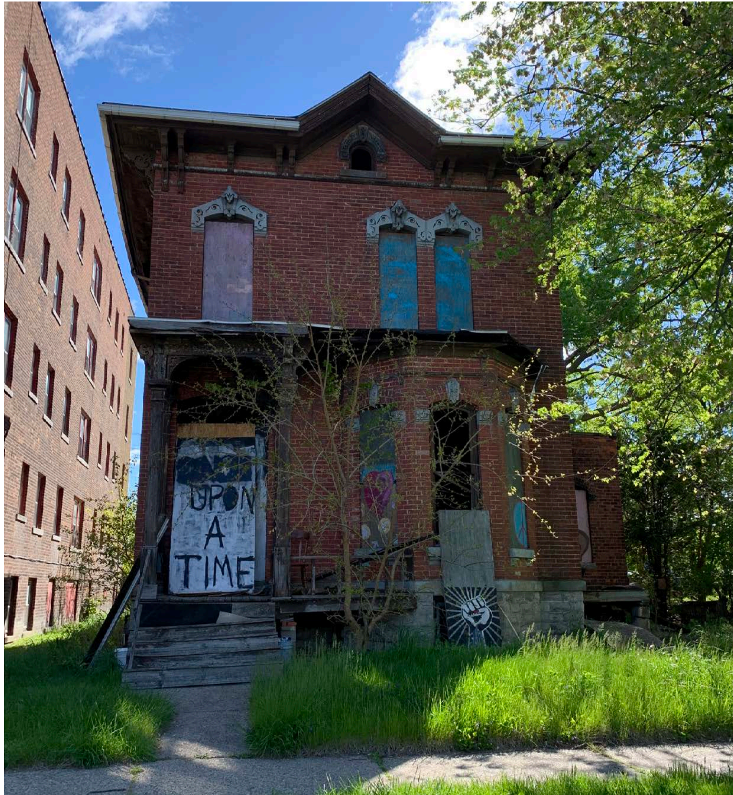
3644 LINCOLN STREET - IN HISTORIC DISTRICT
