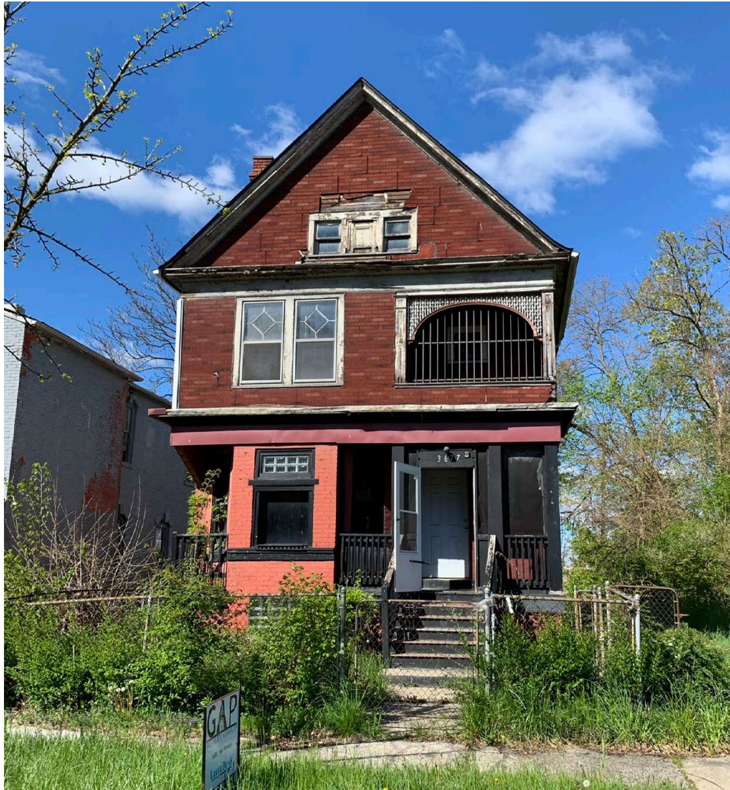
3677 LINCOLN STREET - IN HISTORIC DISTRICT
