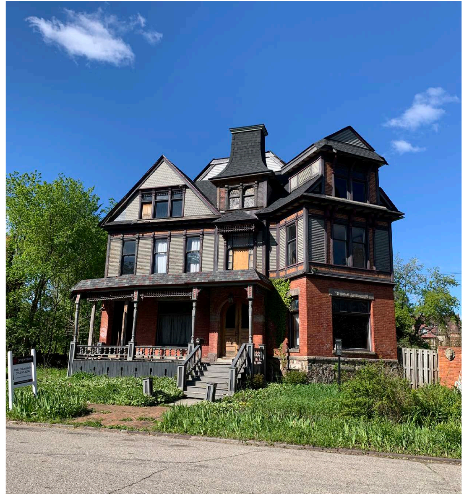
3971 LINCOLN STREET - IN HISTORIC DISTRICT
