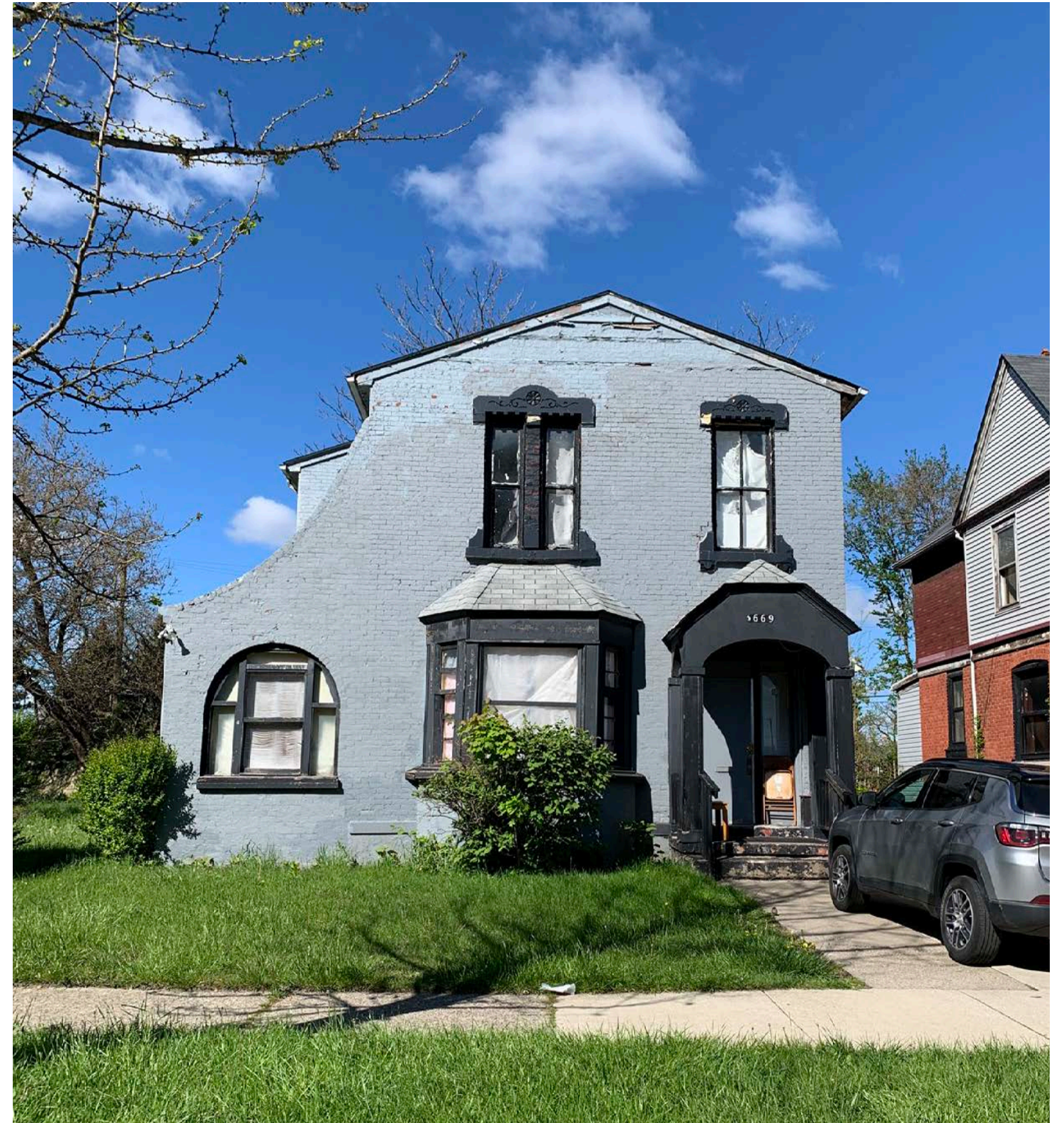
3669 LINCOLN STREET - IN HISTORIC DISTRICT
