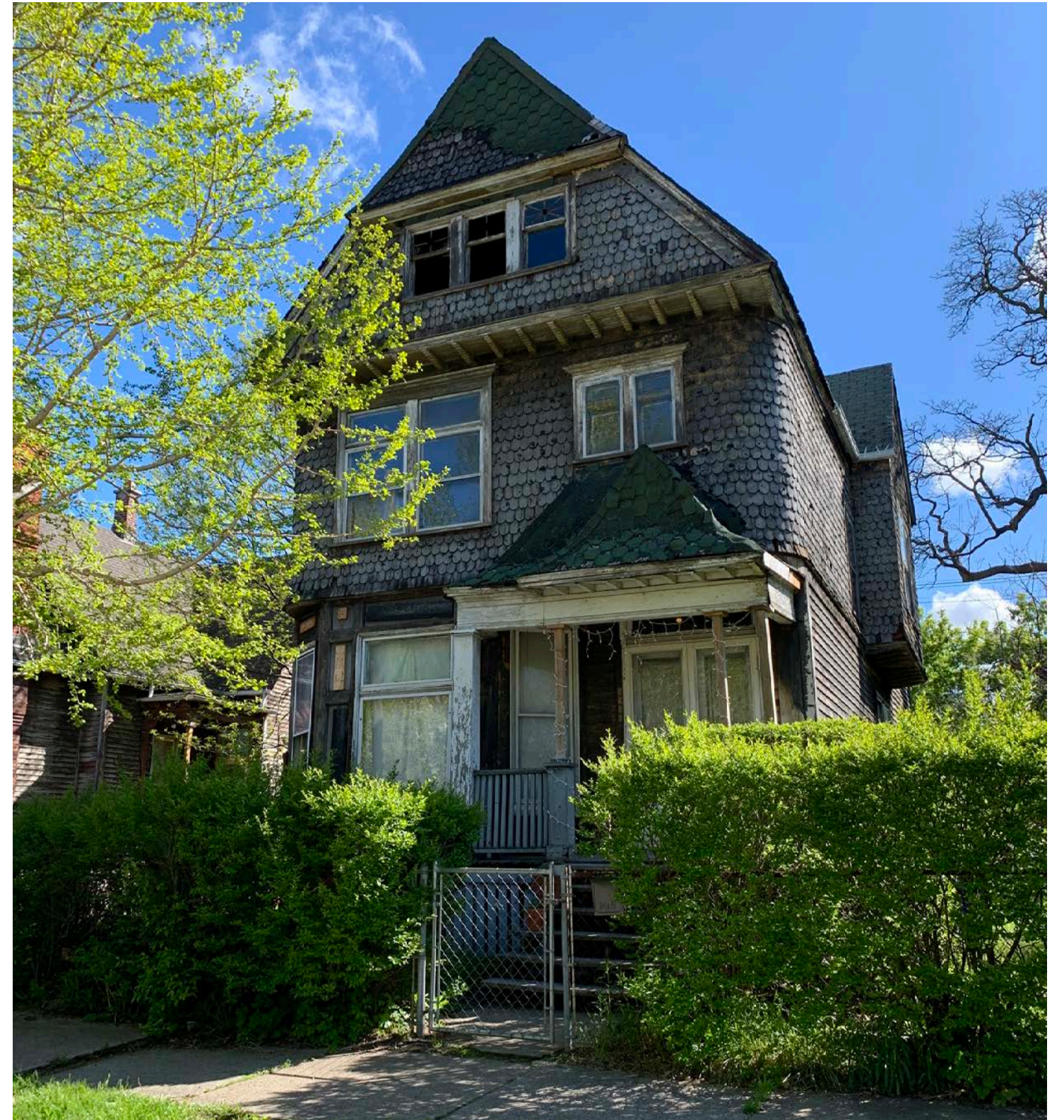
4138 LINCOLN STREET - IN HISTORIC DISTRICT
