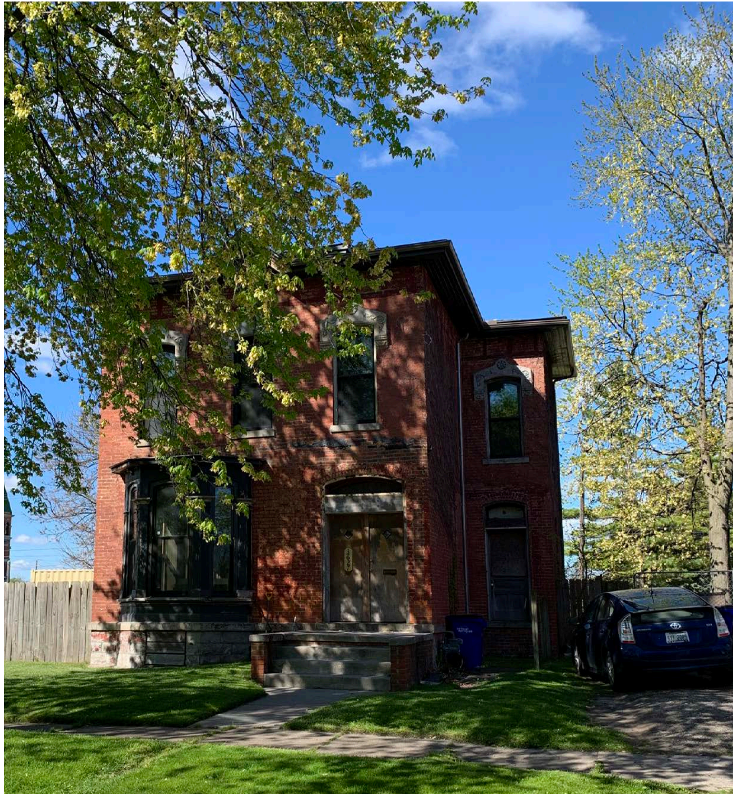
3627 LINCOLN STREET - IN HISTORIC DISTRICT
