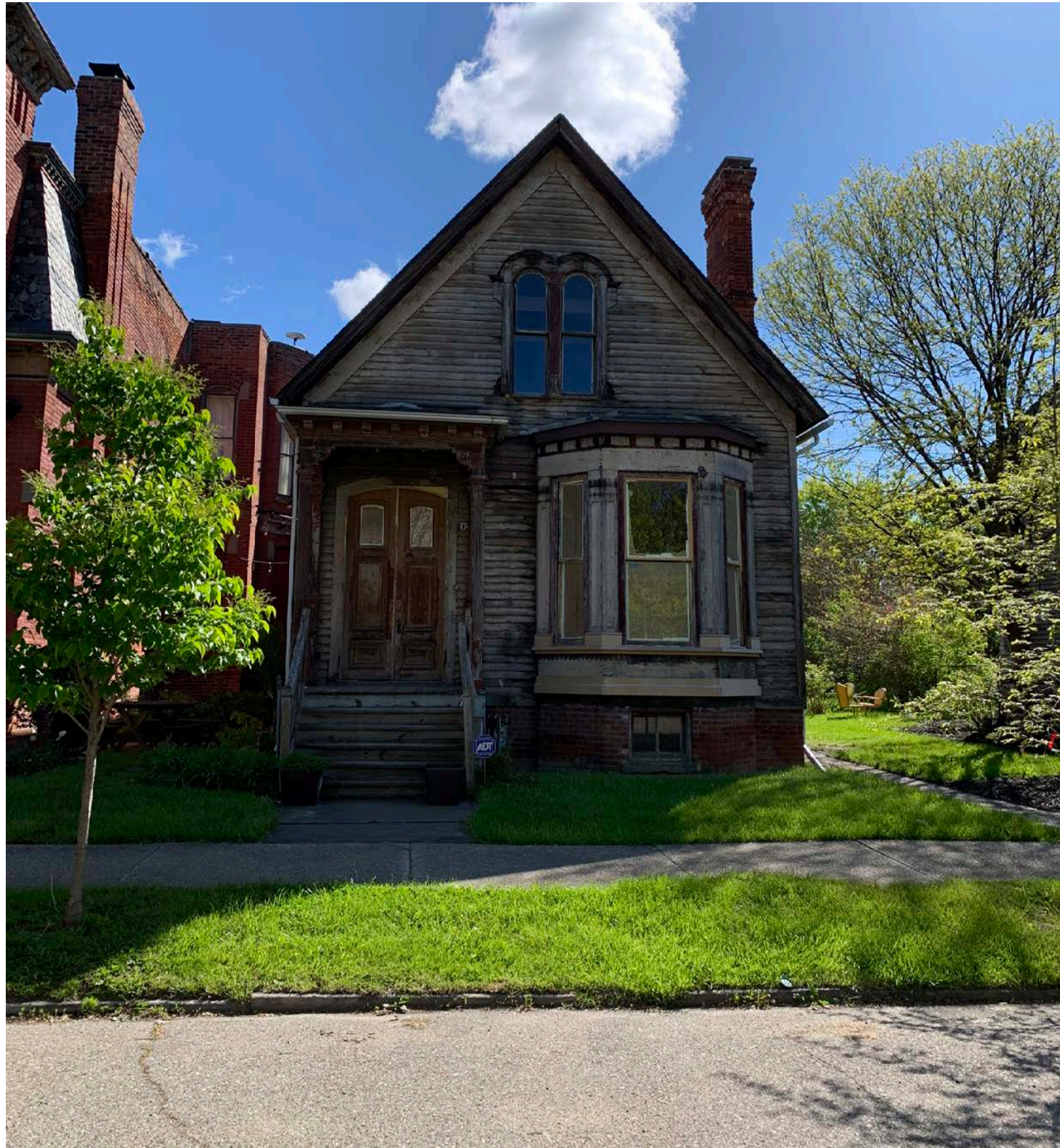
4144 LINCOLN STREET - IN HISTORIC DISTRICT
