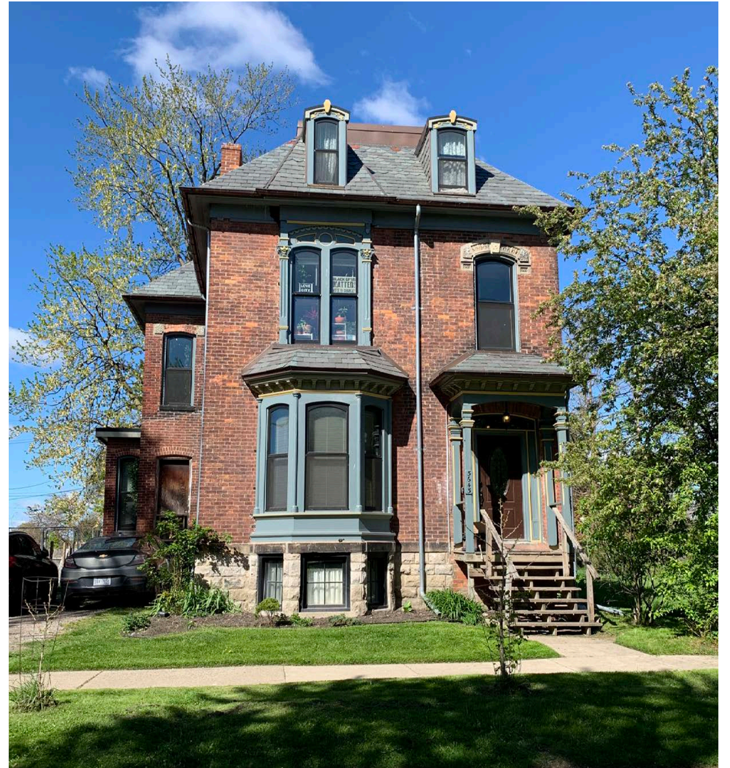
3643 LINCOLN STREET - IN HISTORIC DISTRICT
