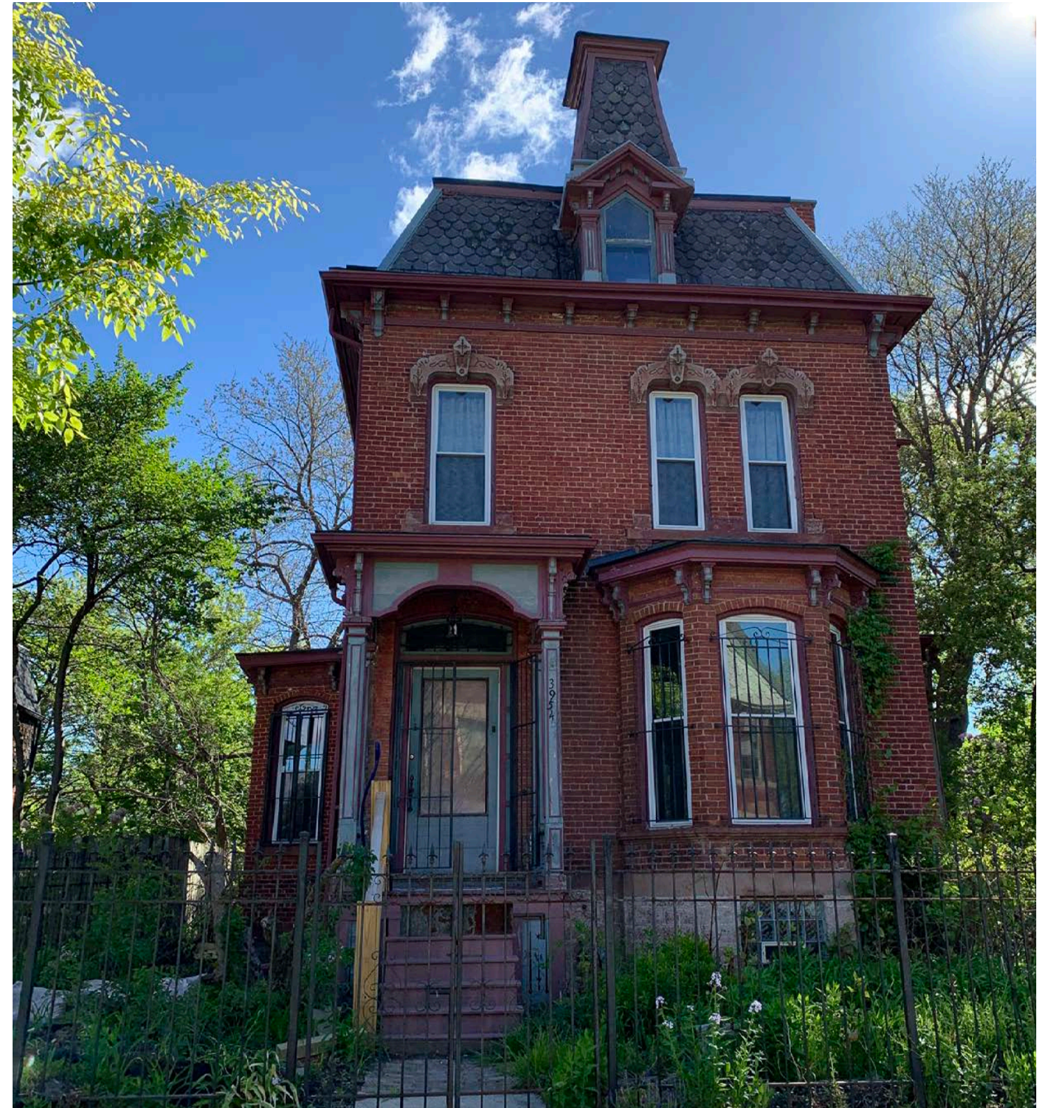
3954 LINCOLN STREET - IN HISTORIC DISTRICT
