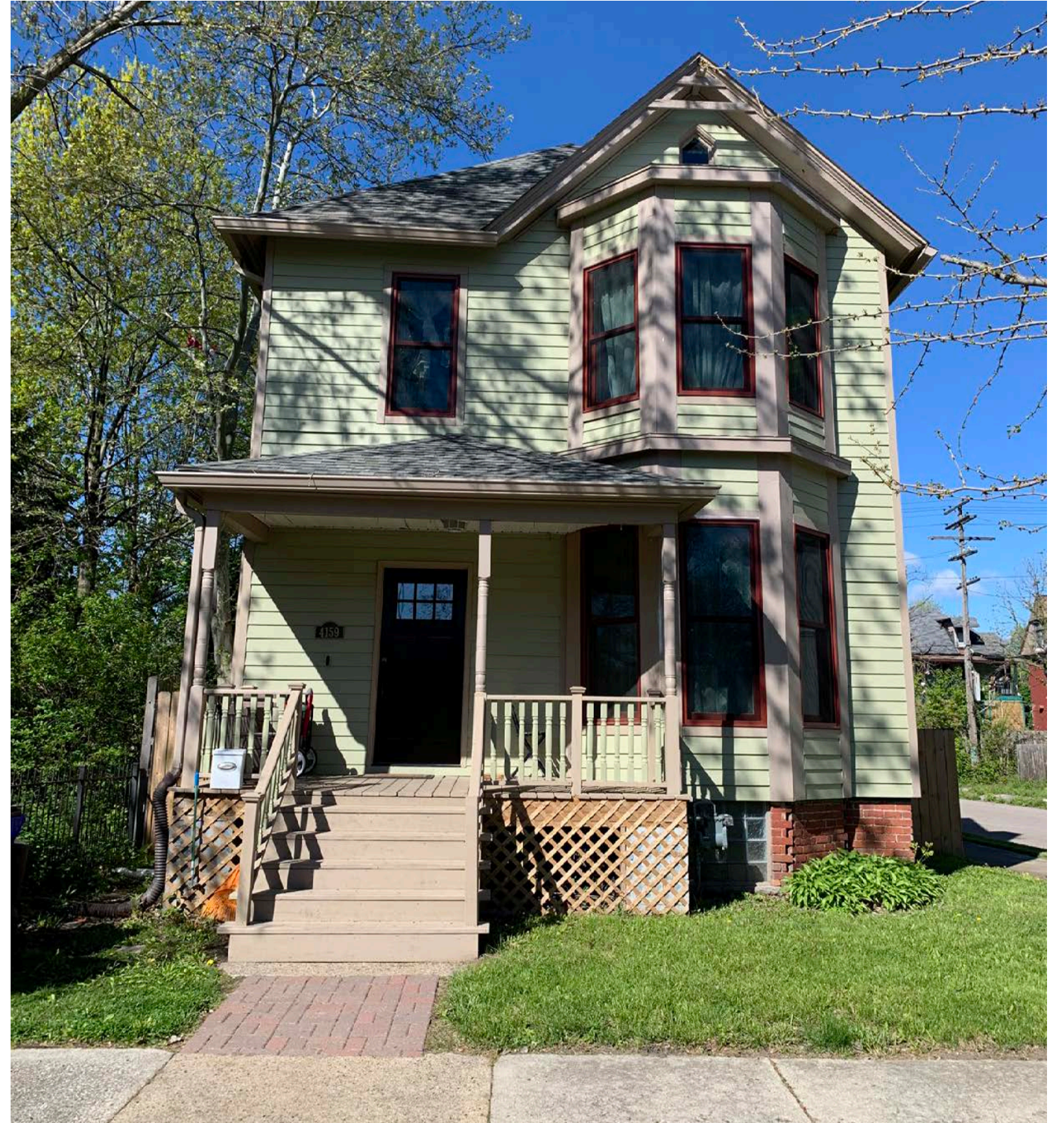
4159 LINCOLN STREET - IN HISTORIC DISTRICT
