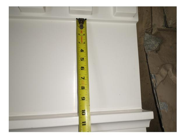
New decorative leaf location (proposed height of new applied piece (8)" to be centered in the offsets between the dentals & lower offset.
