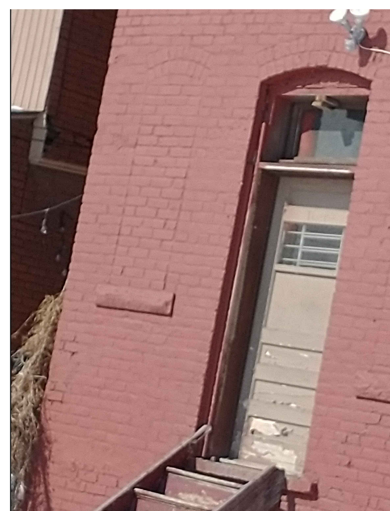
Existing Unit Rear Door (CURRENT)
