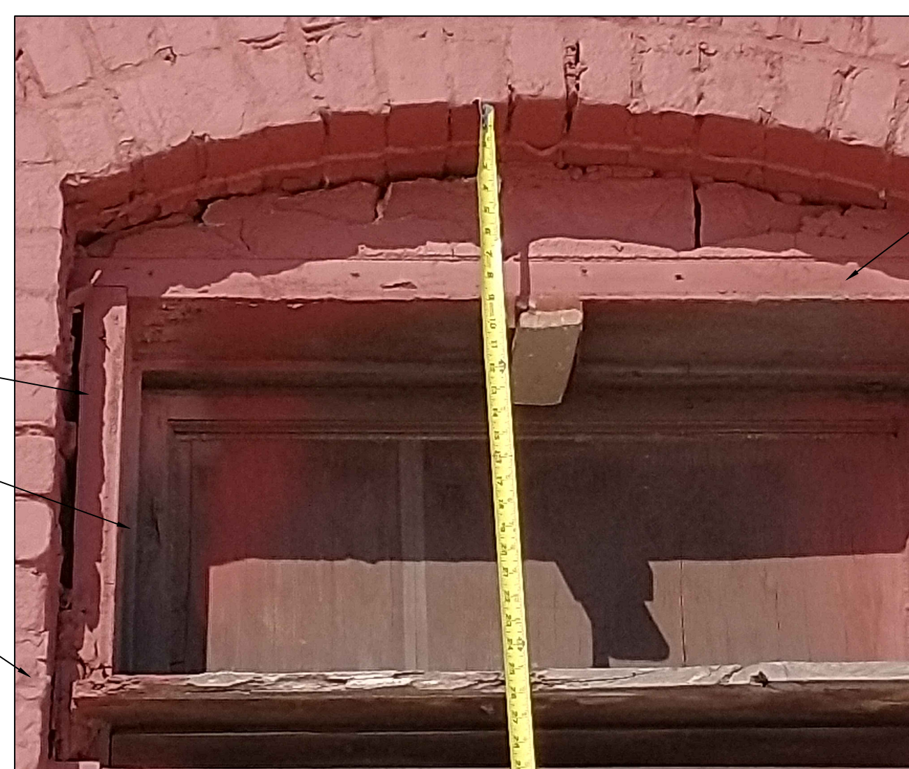
Enlarged View of Existing Door Transom Opening
