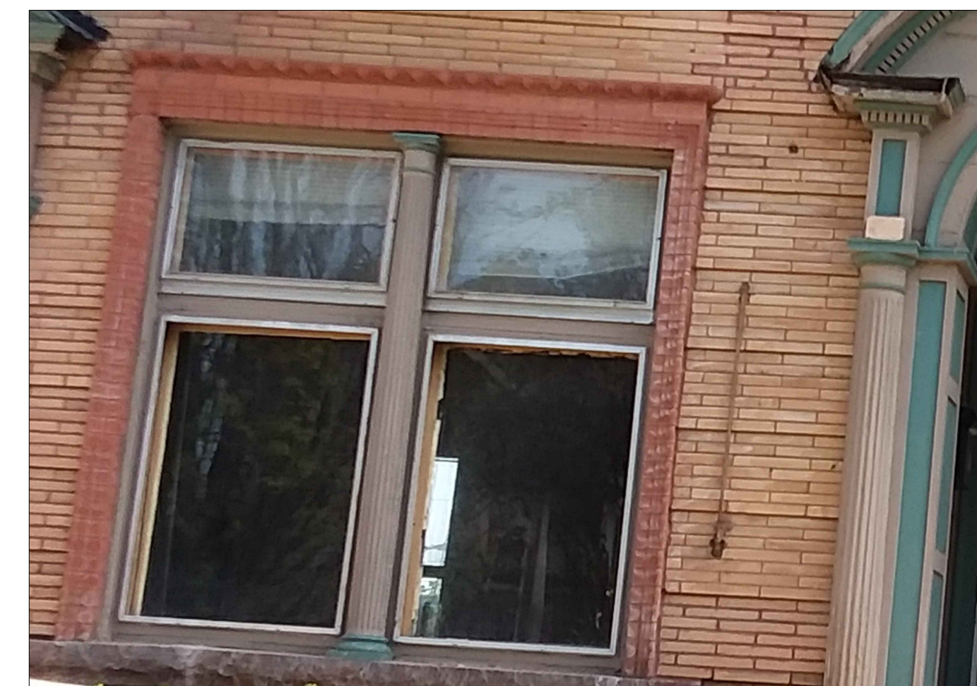
Window Before Replacement
