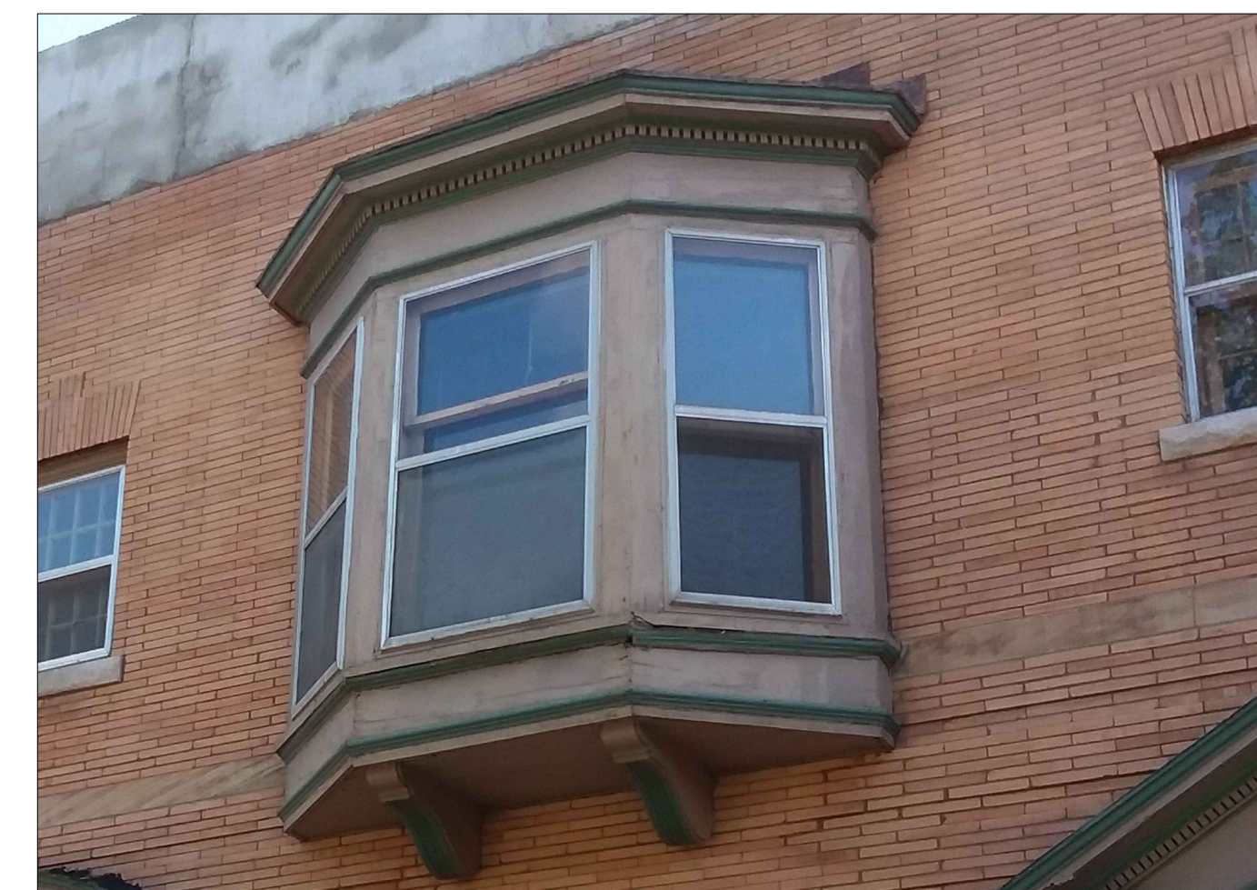
Bay Window Before Replacement
