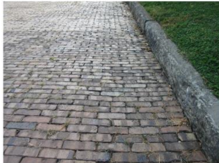
Embry Ave. brick pavers and limestone curb
