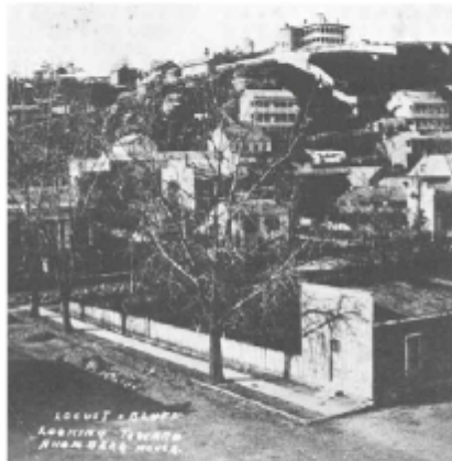
6.62 Seventh Street left from 5th and Locust, possibly in the late 1880's. The upper slopes are planted to plantings.
