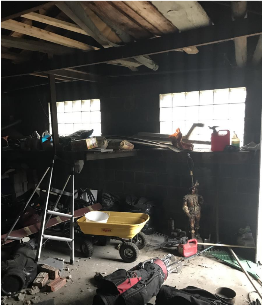
Interior of front/west elevation
