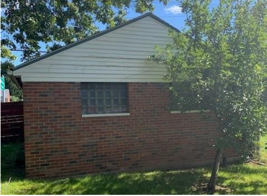
Front/west elevation - Garage
