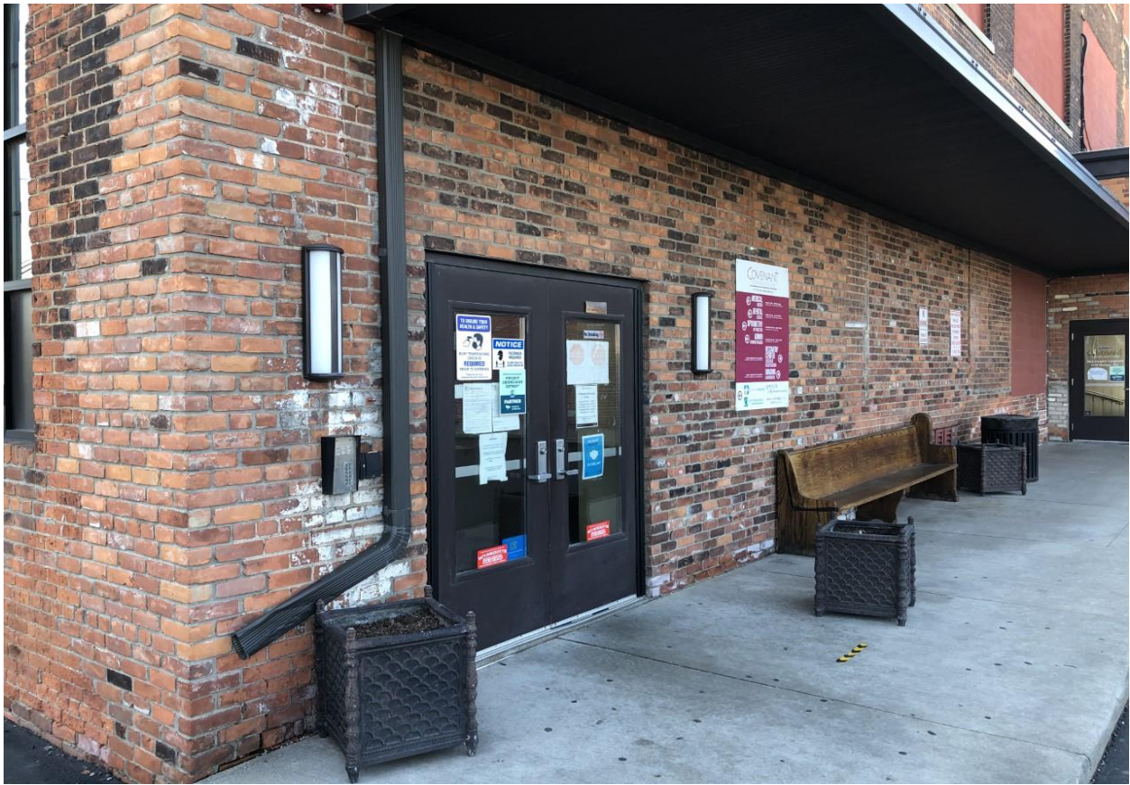
5716 MI AVE, West Elevation Entrance-Close UP
