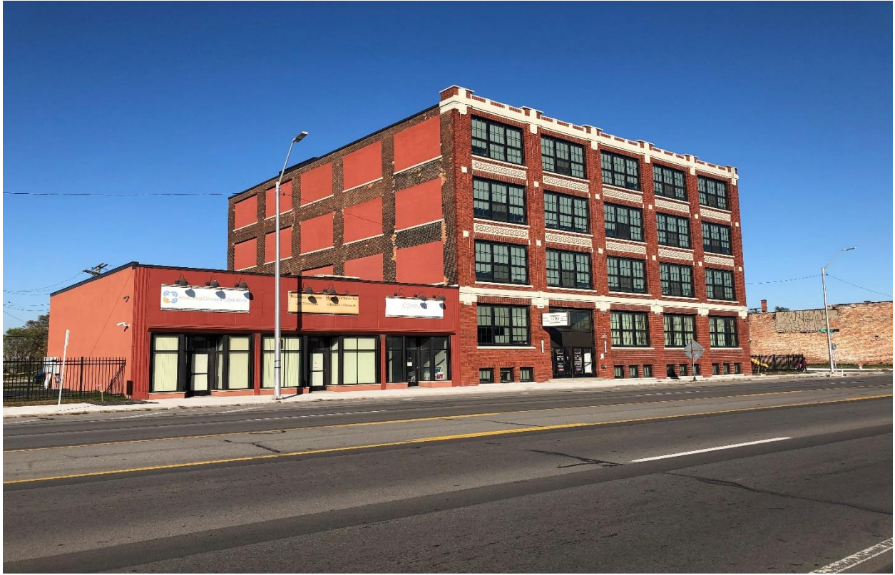
5716 MI AVE, South Elevation
