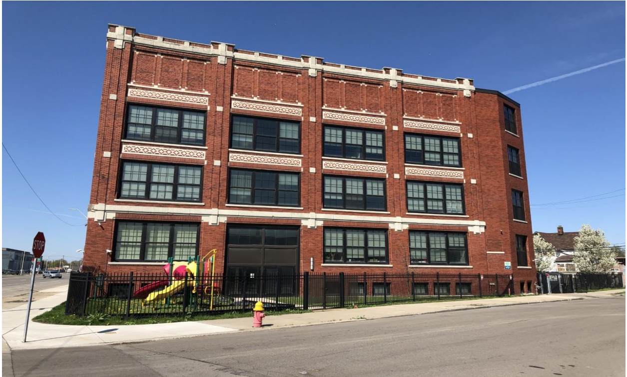
5716 MI AVE, East Elevation
