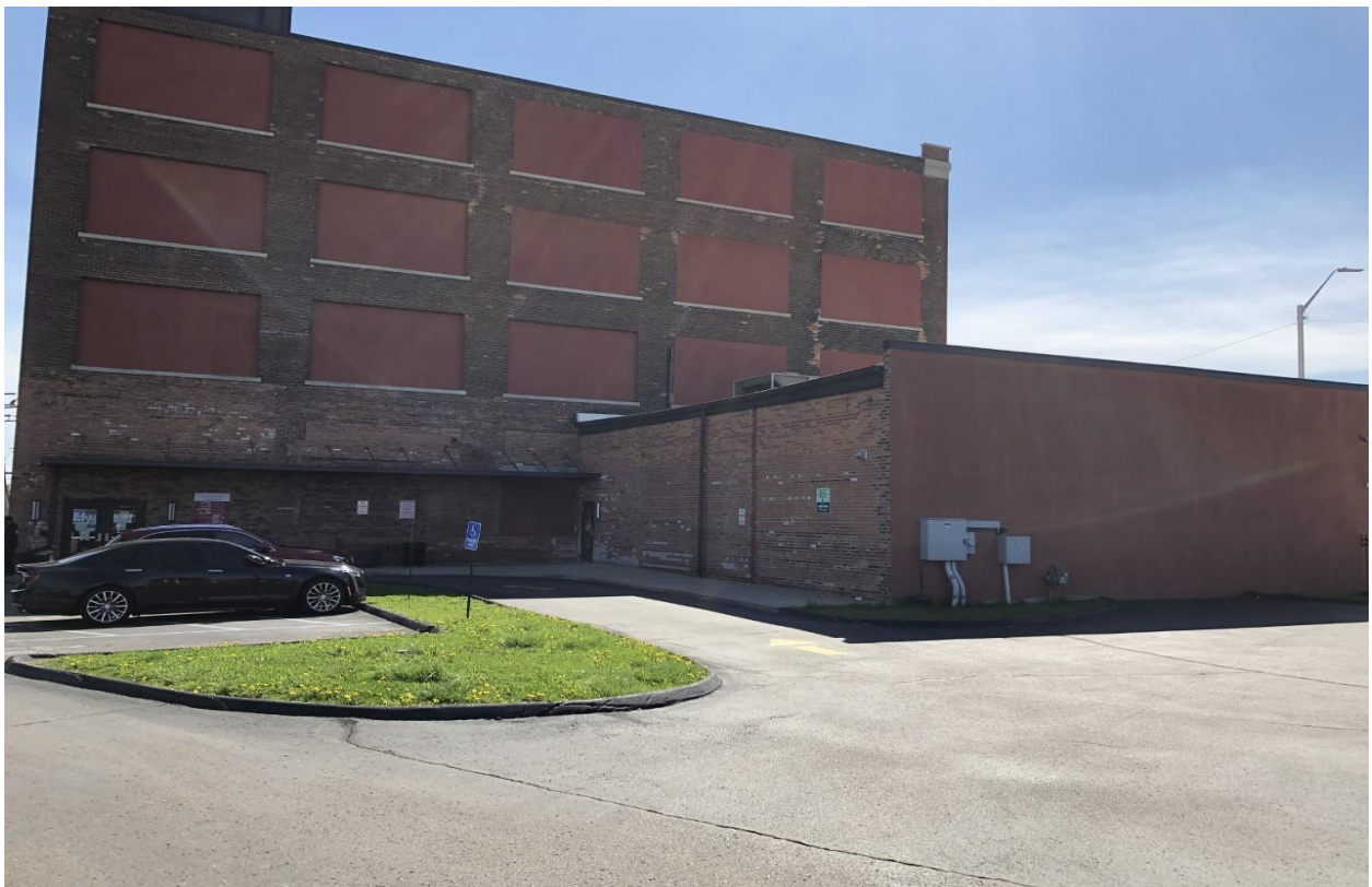
5716 MI AVE, West Elevation
