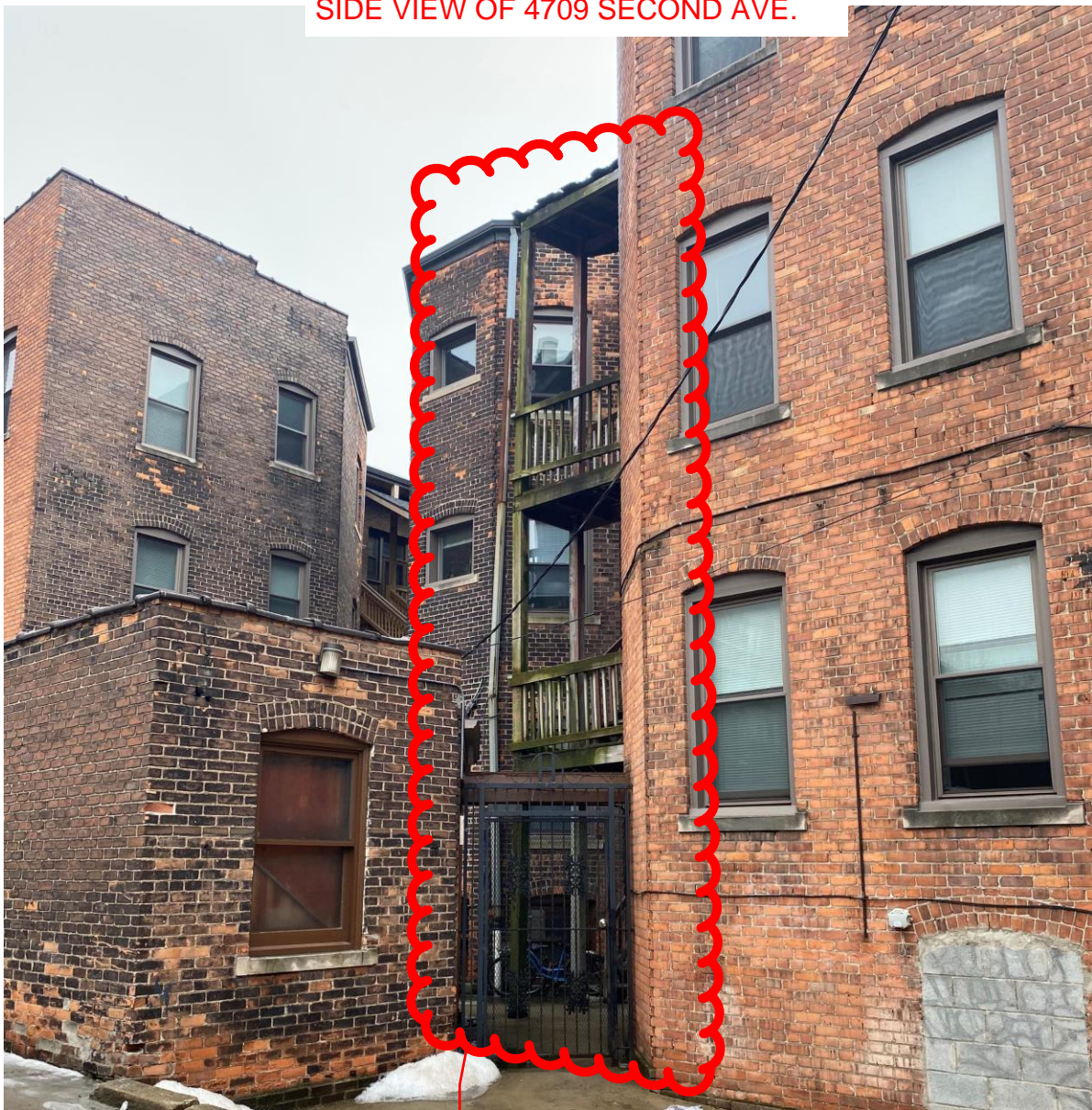
DEMO EXISTING STAIR CASE AND REBUILD NEW
