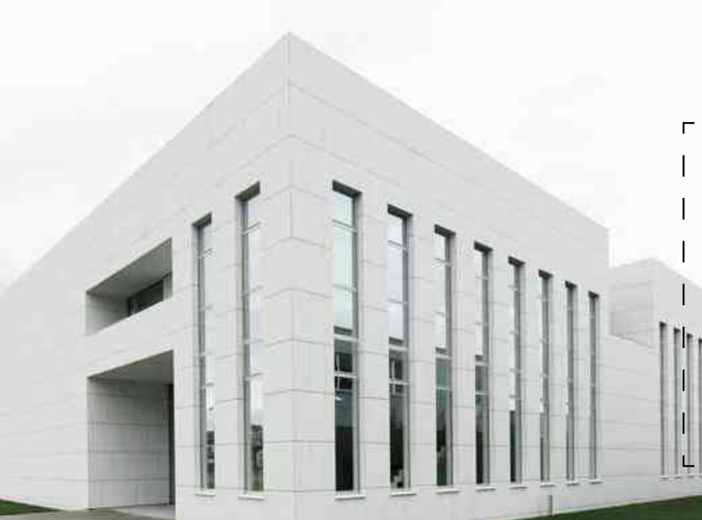
Office & production building | Spießberger Bau concrete skin in polar white with ferro
