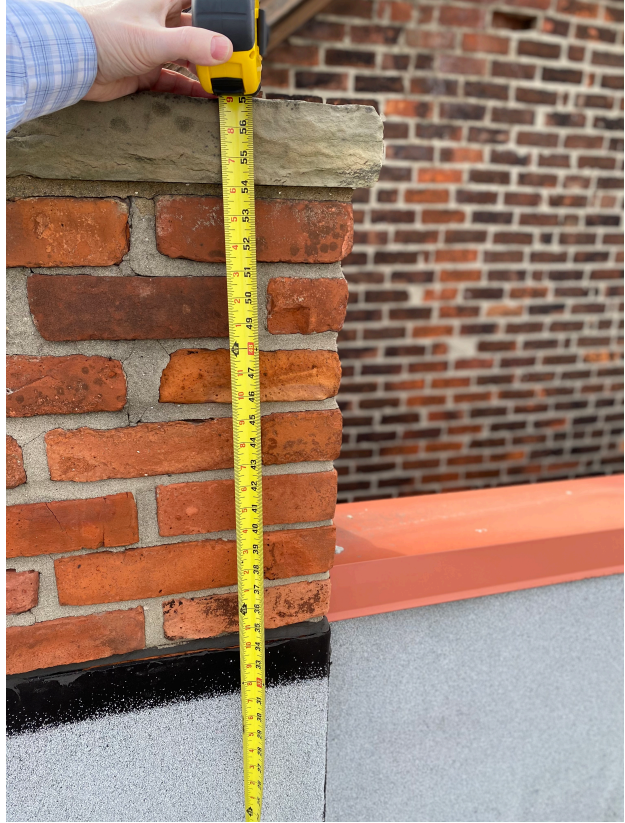
Existing chimney height of +/- 4'-9"
