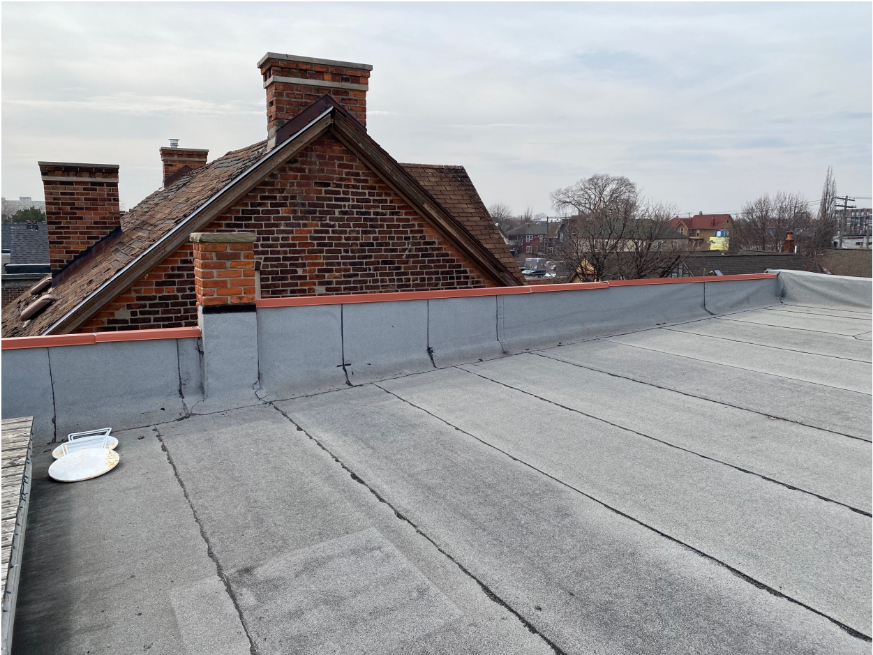
Area of roof where new HVAC Unit will be placed.
