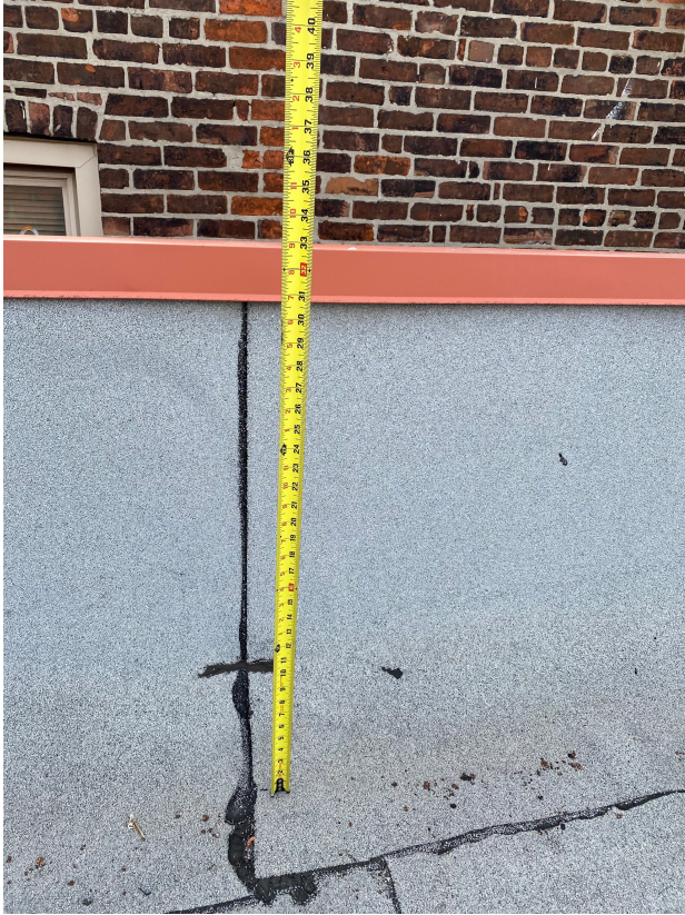
Existing parapet height at +/- 2'-9"
