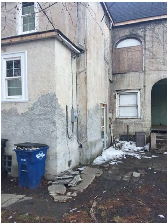
STUCCO DETERIORATION AT SW CORNER OF BUILDING
