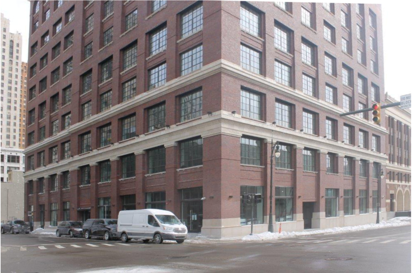
North and West Storefront Elevations after rehabilitation looking se.
