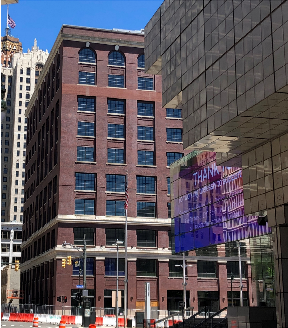
West Elevation looking east during construction.
