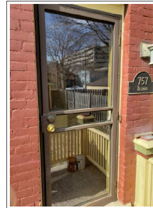
EXTERIOR STORM DOOR CONDITION
