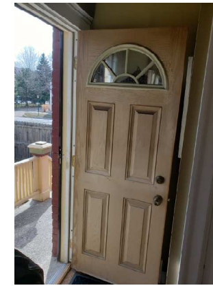
EXTERIOR DOOR CONDITION
