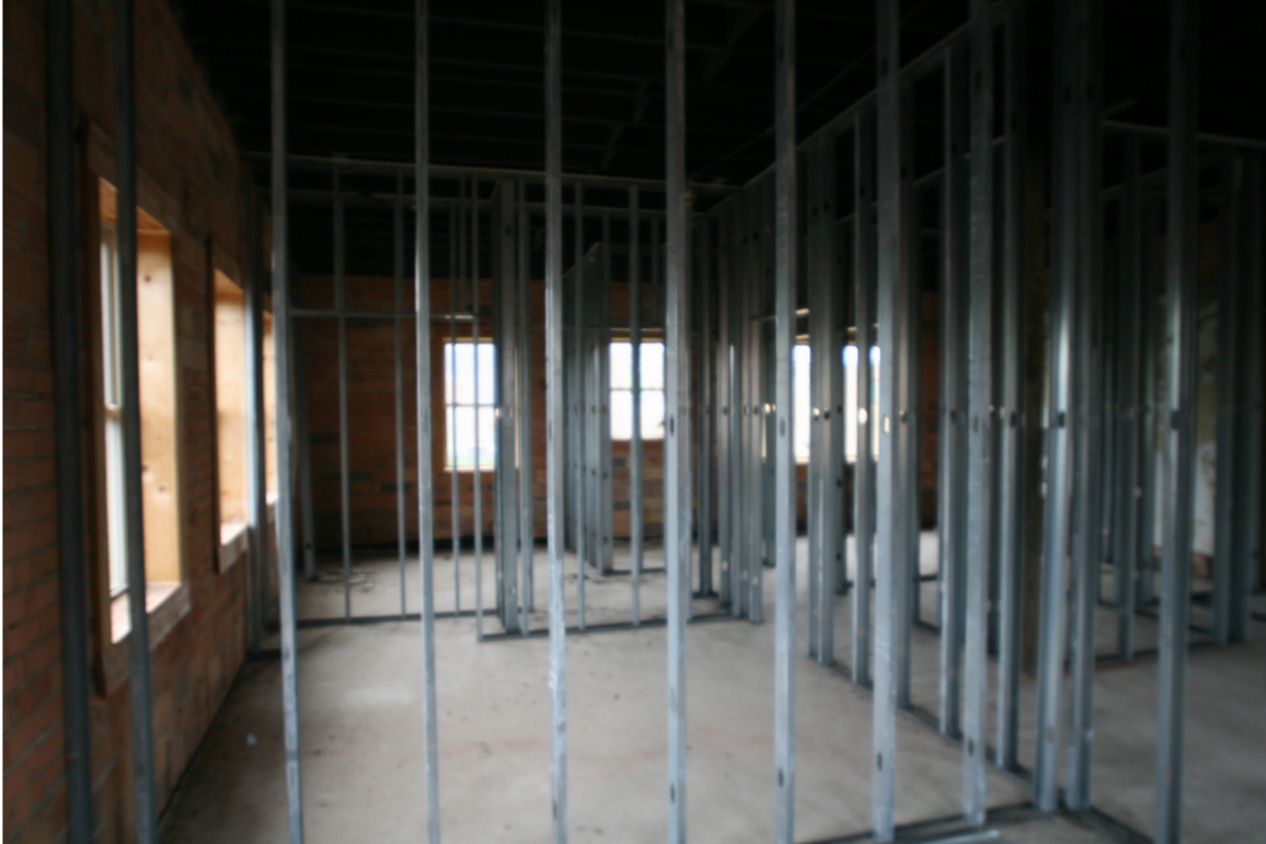
21. Interior View, Third Floor at Northwest, Looking E
