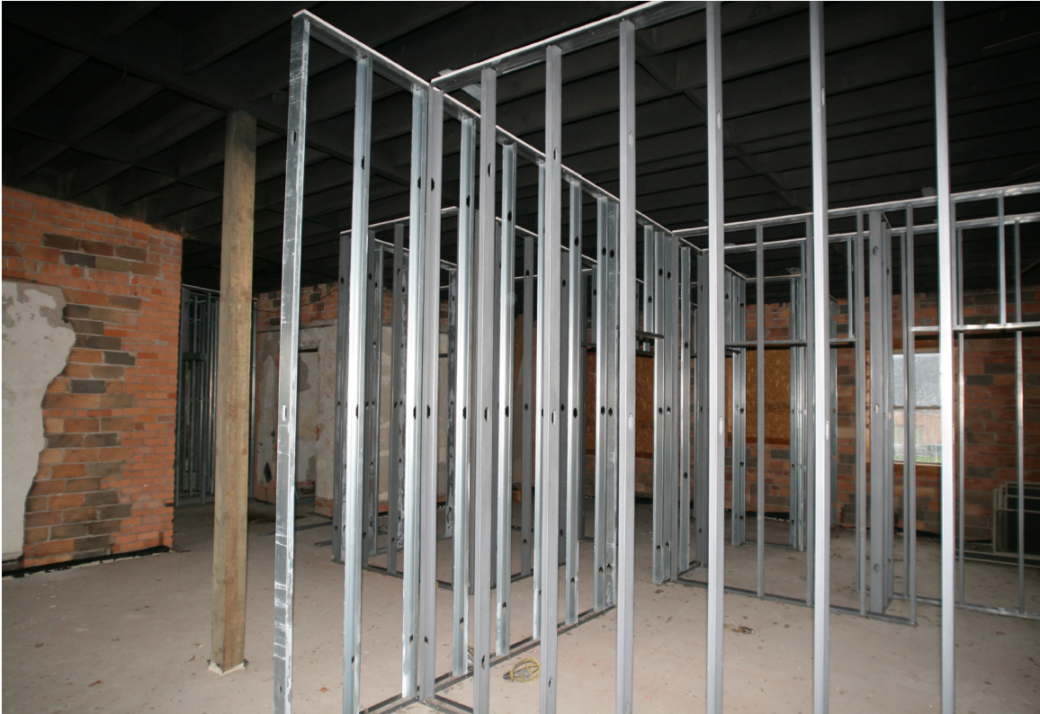
22. Interior View, Third Floor at Southwest, Looking NE
