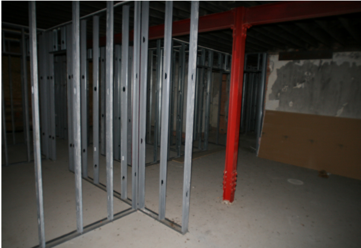
12. Interior View, First Floor at Northwest, Looking SE
