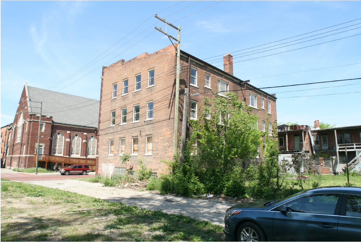
7. Exterior View, South and East Elevations, Looking NW
