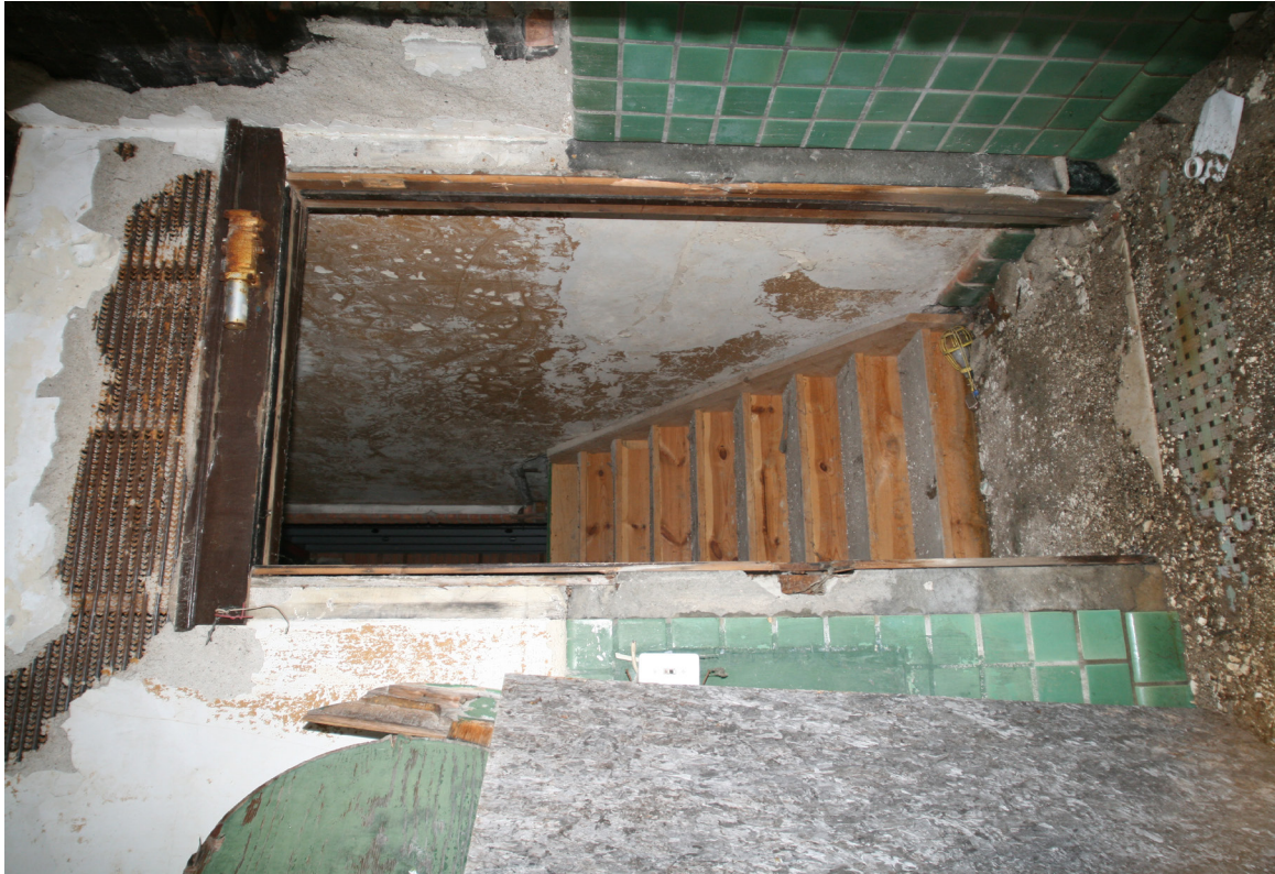
10. Interior View, First Floor, Entry, Looking W
