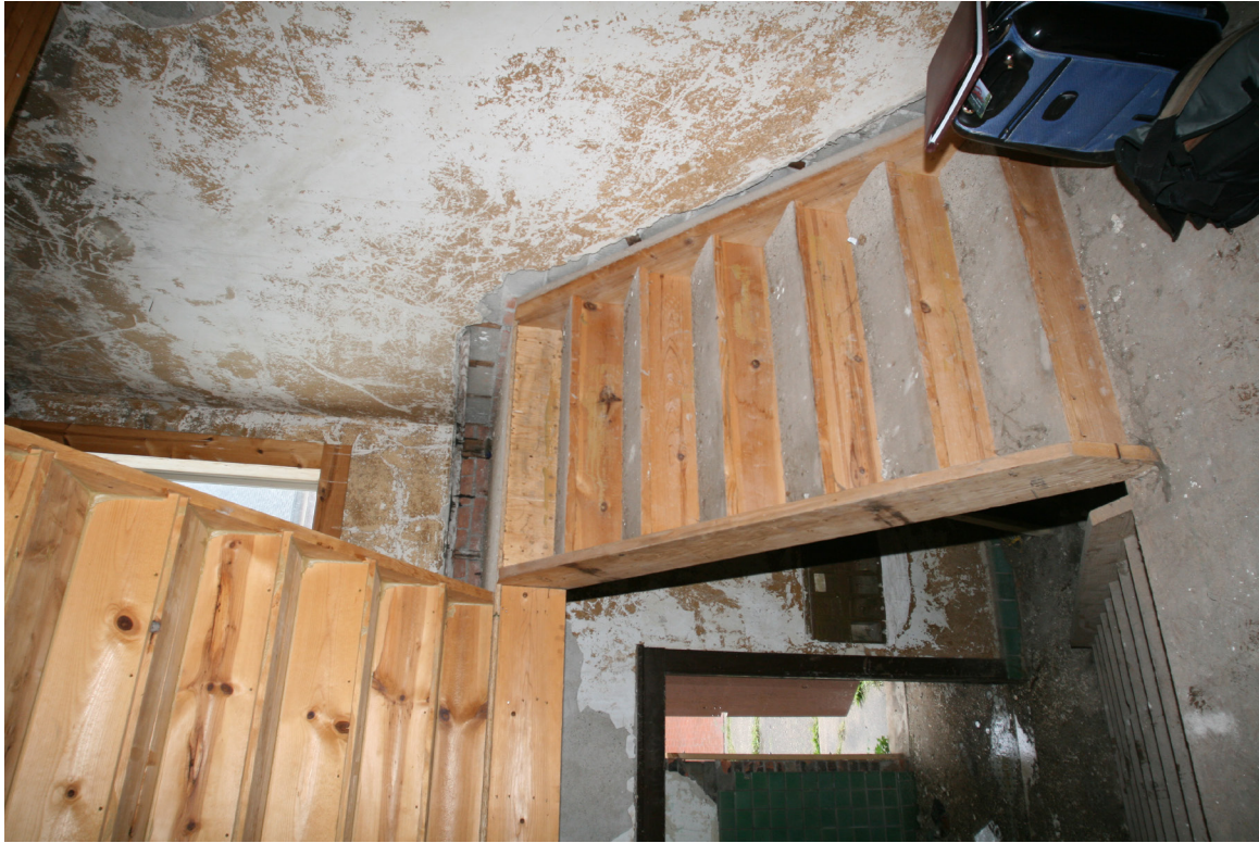
11. Interior View, First Floor, Stair at Center-West, Looking W
