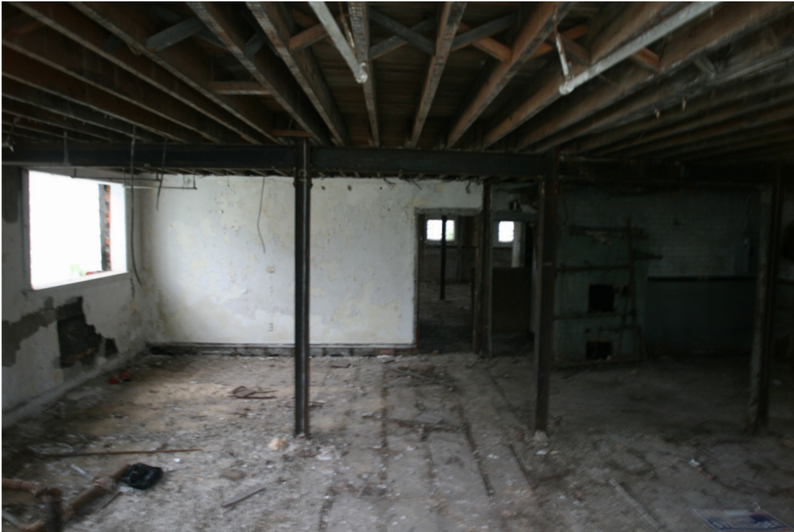
25. Interior View, Basement at Center-South, Looking N
