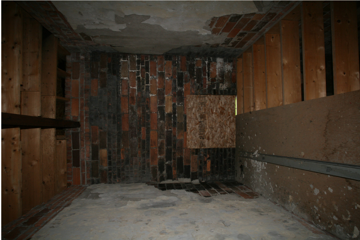
19. Interior View, Third Floor at Center-East, Looking E
