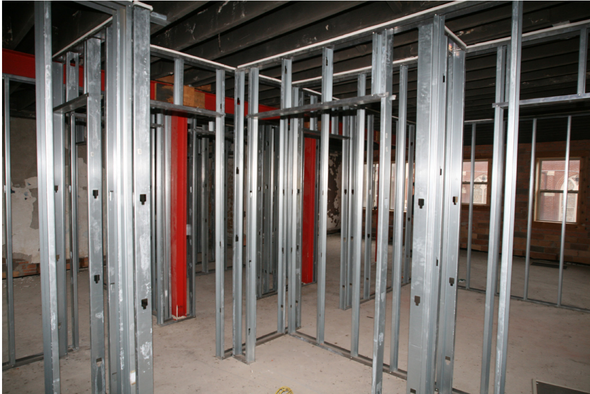
17. Interior View, Second Floor at Northeast, Looking SW
