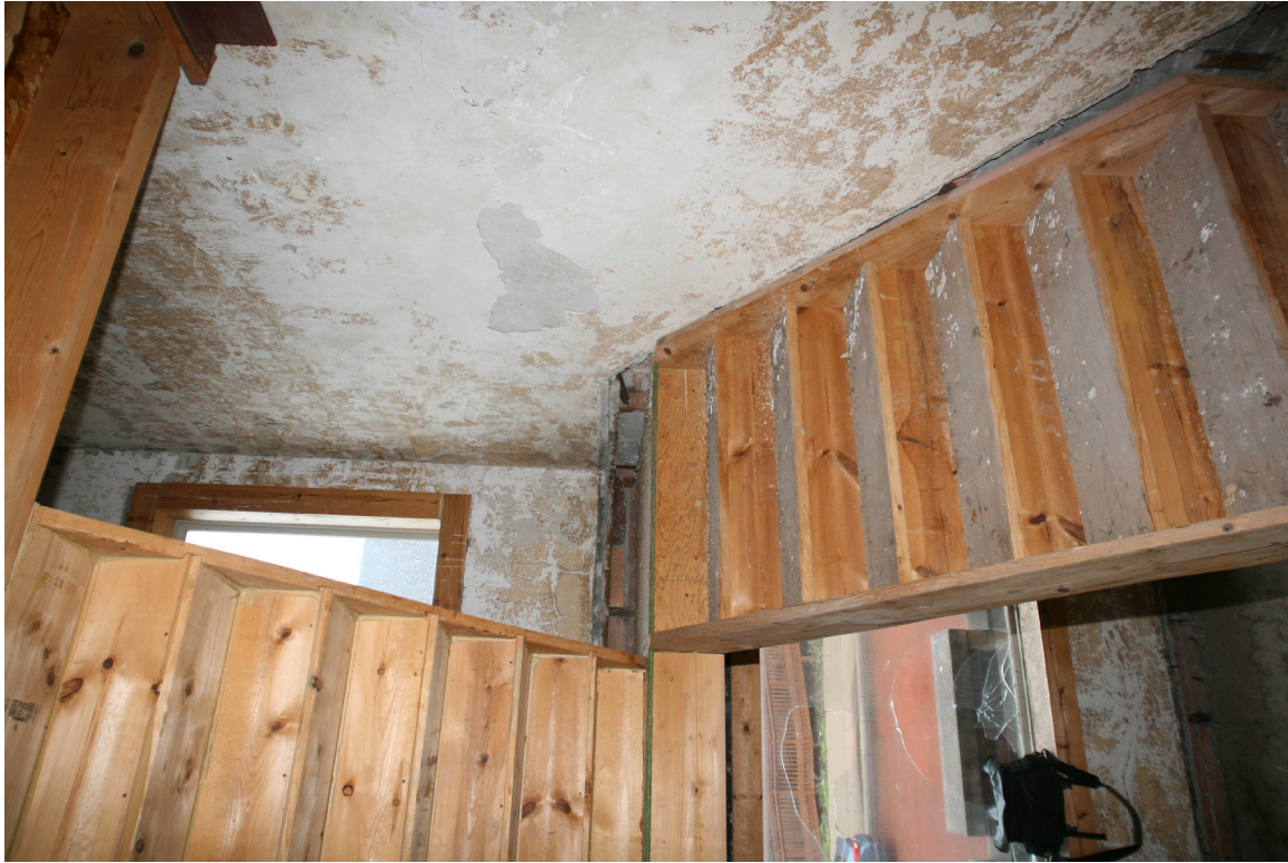
15. Interior View, Second Floor, Stair at Center-West, Looking W
