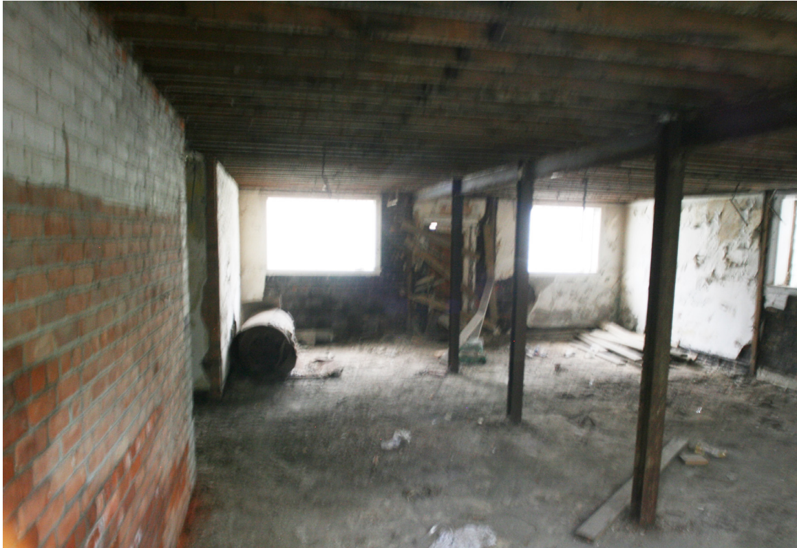
24. Interior View, Basement at Center-East, Looking NW
