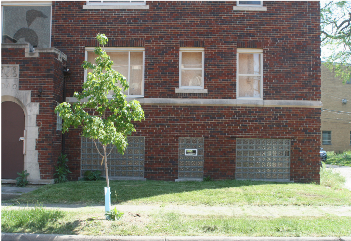
4. Exterior Detail, West Elevation at South, Lower Floors, Looking W
