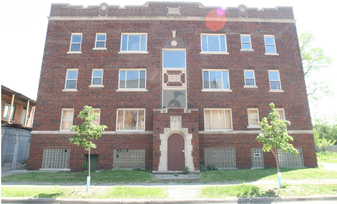
1. Exterior View, West Elevation, Looking E
