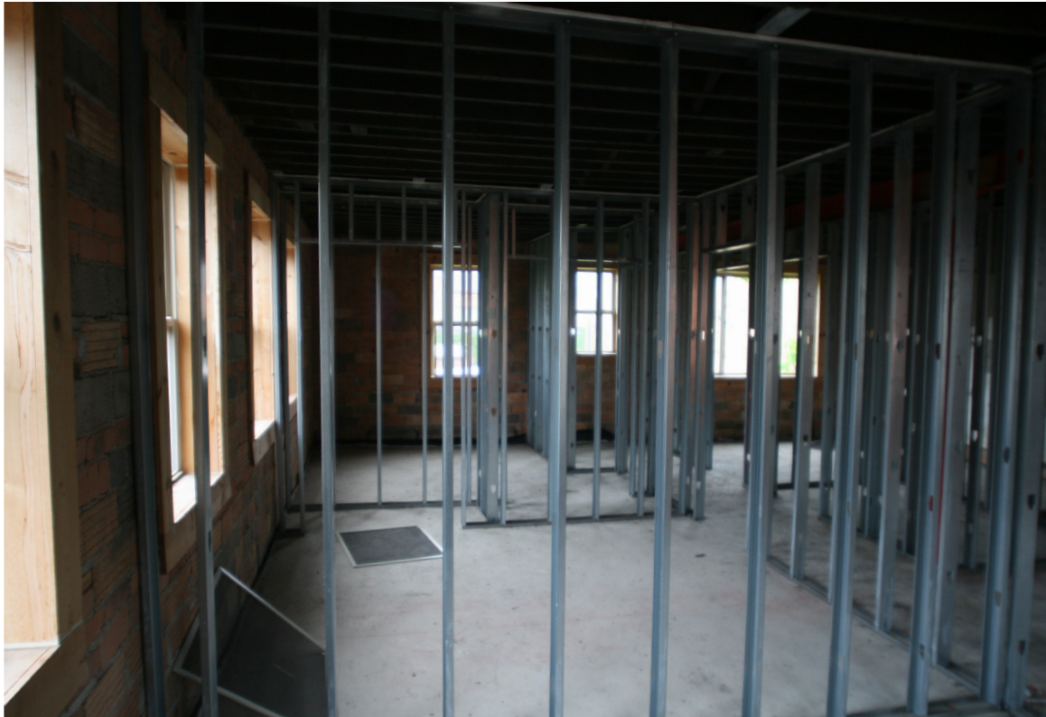
16. Interior View, Second Floor at Center-West, Looking N
