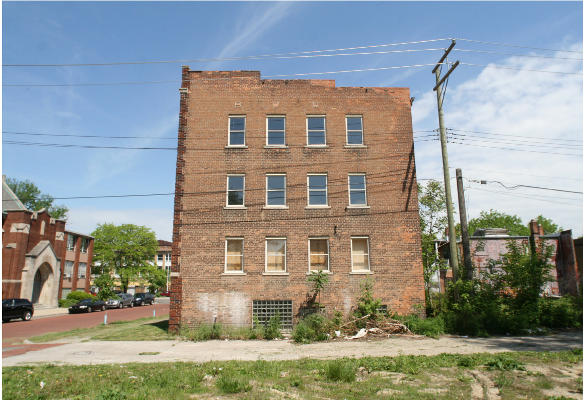
6. Exterior View, South Elevation, Looking N
