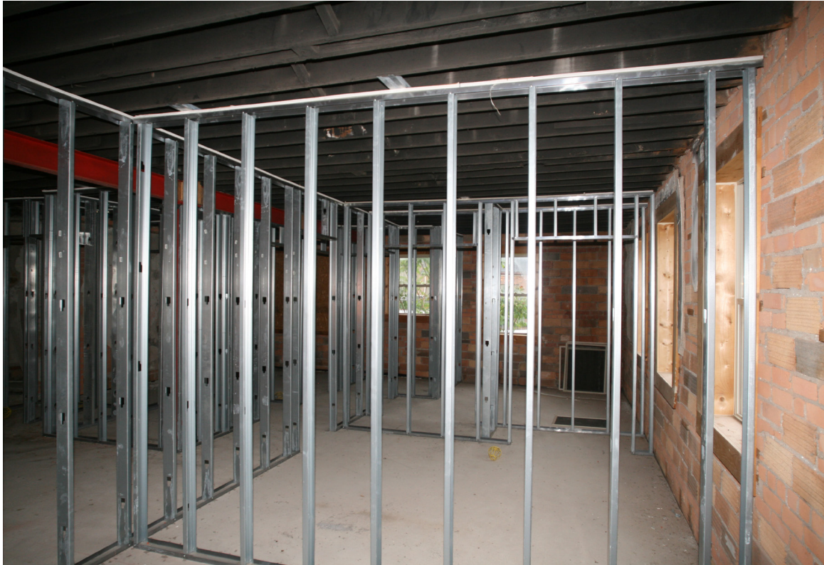
18. Interior View, Second Floor at Southwest, Looking E
