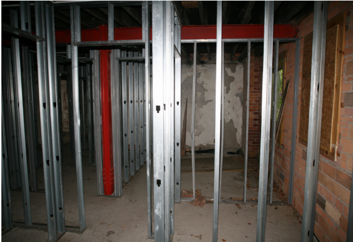
14. Interior View, First Floor at Southeast, Looking N
