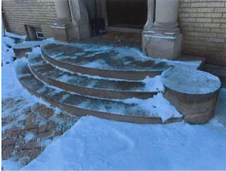
5- West/Front Entry Stoop , detail
