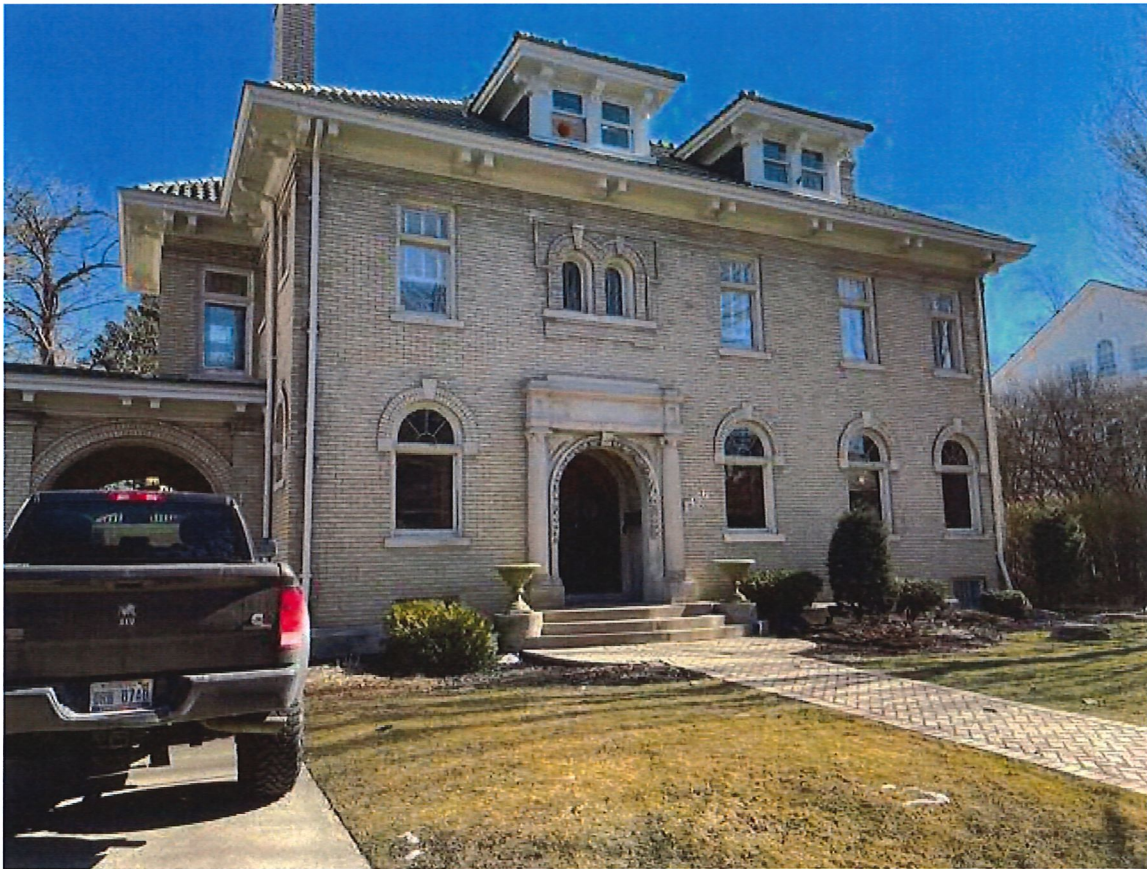
6- Front Walk Existing , detail
