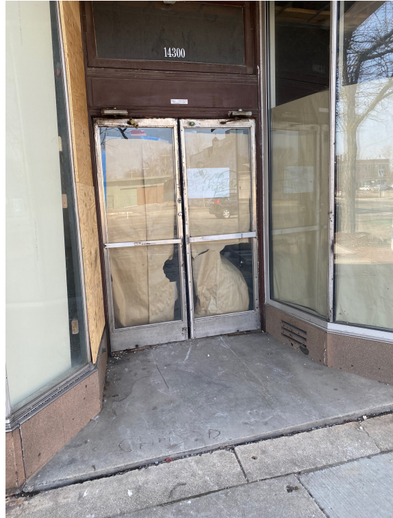
Existing Exterior of doors
