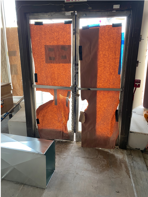
Existing Interior of doors
