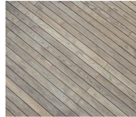
THERMALLY MODIFIED WOOD (THERMORY - WHITE ASH) REAR DECK
