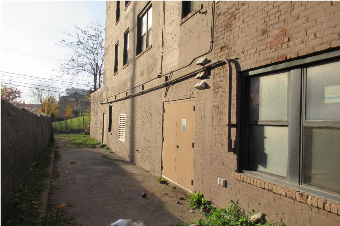
Figure #24: Exterior, looking South. 11/6/20
