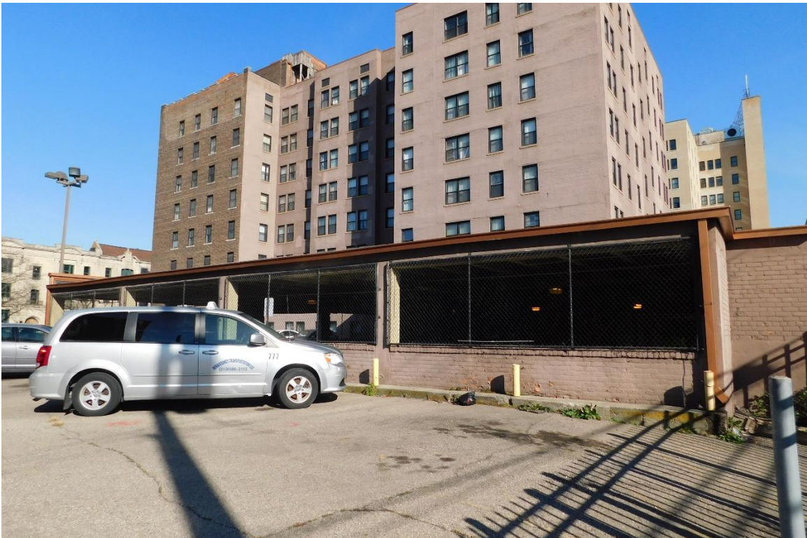
Figure #12: Exterior, Garage, Looking Northeast. 11/18/20
