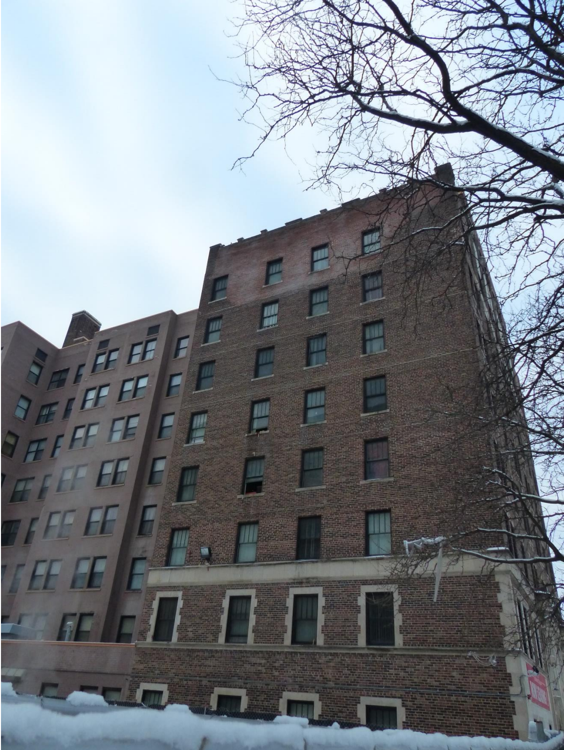
Figure #19: Exterior, Looking West. 12/18/20
