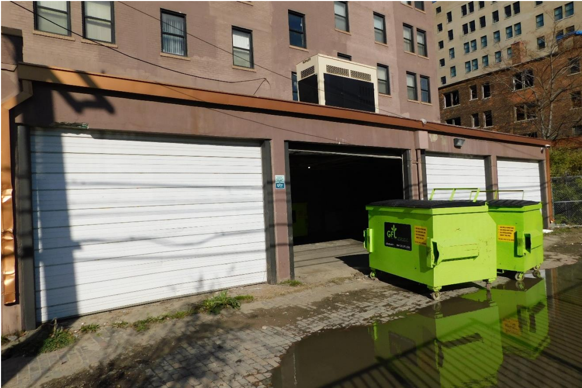
Figure #30: Exterior, Looking North. 11/18/20
