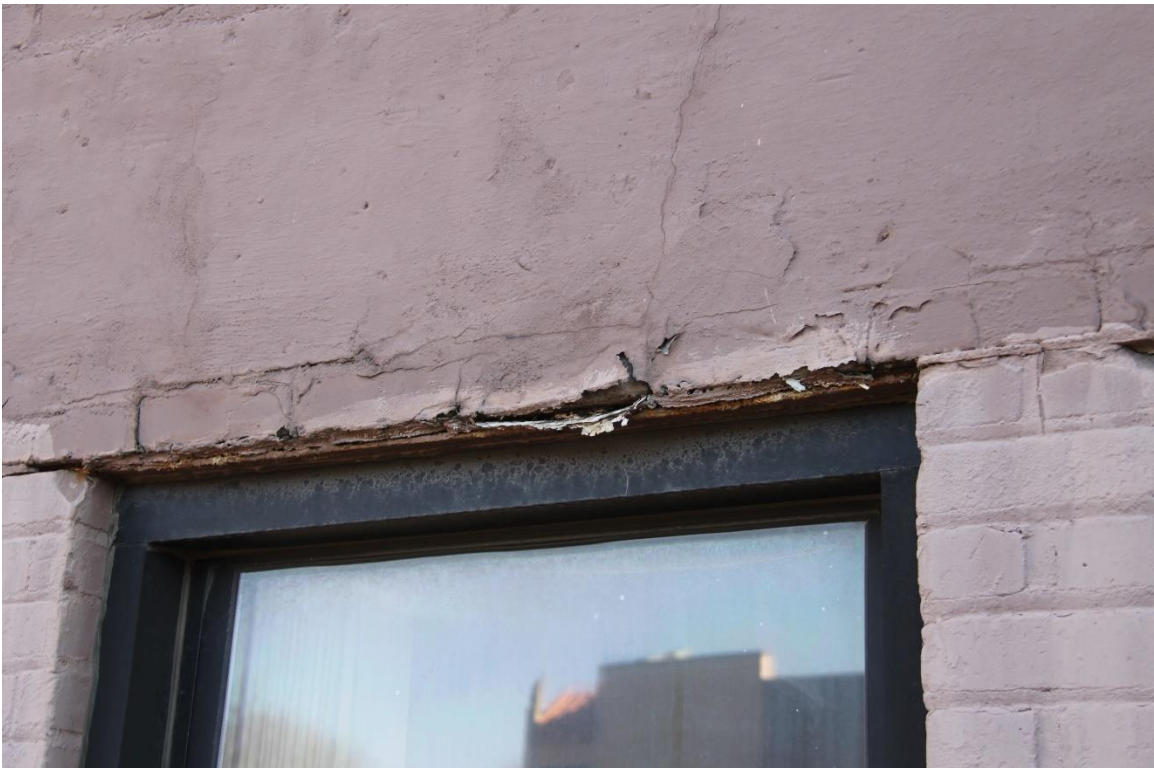
Figure #40: Exterior, Window, Looking Up. 11/18/20
