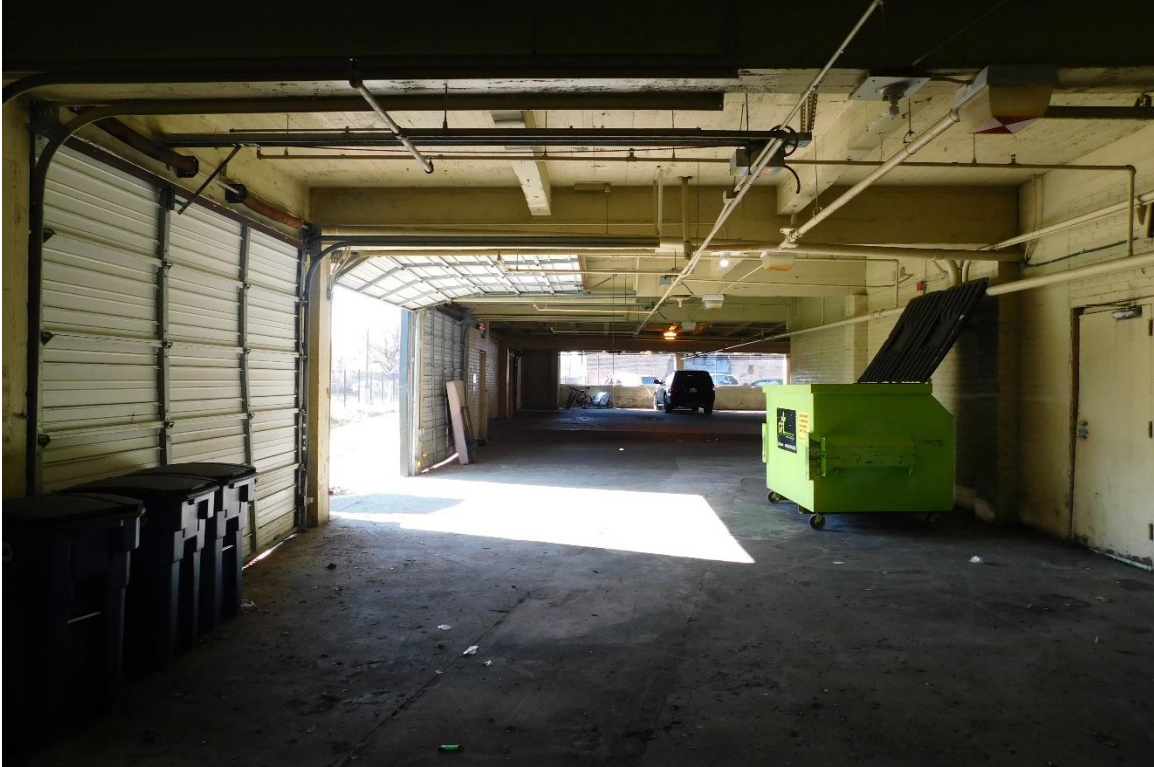
Figure #17: Garage, Looking West. 11/18/20
