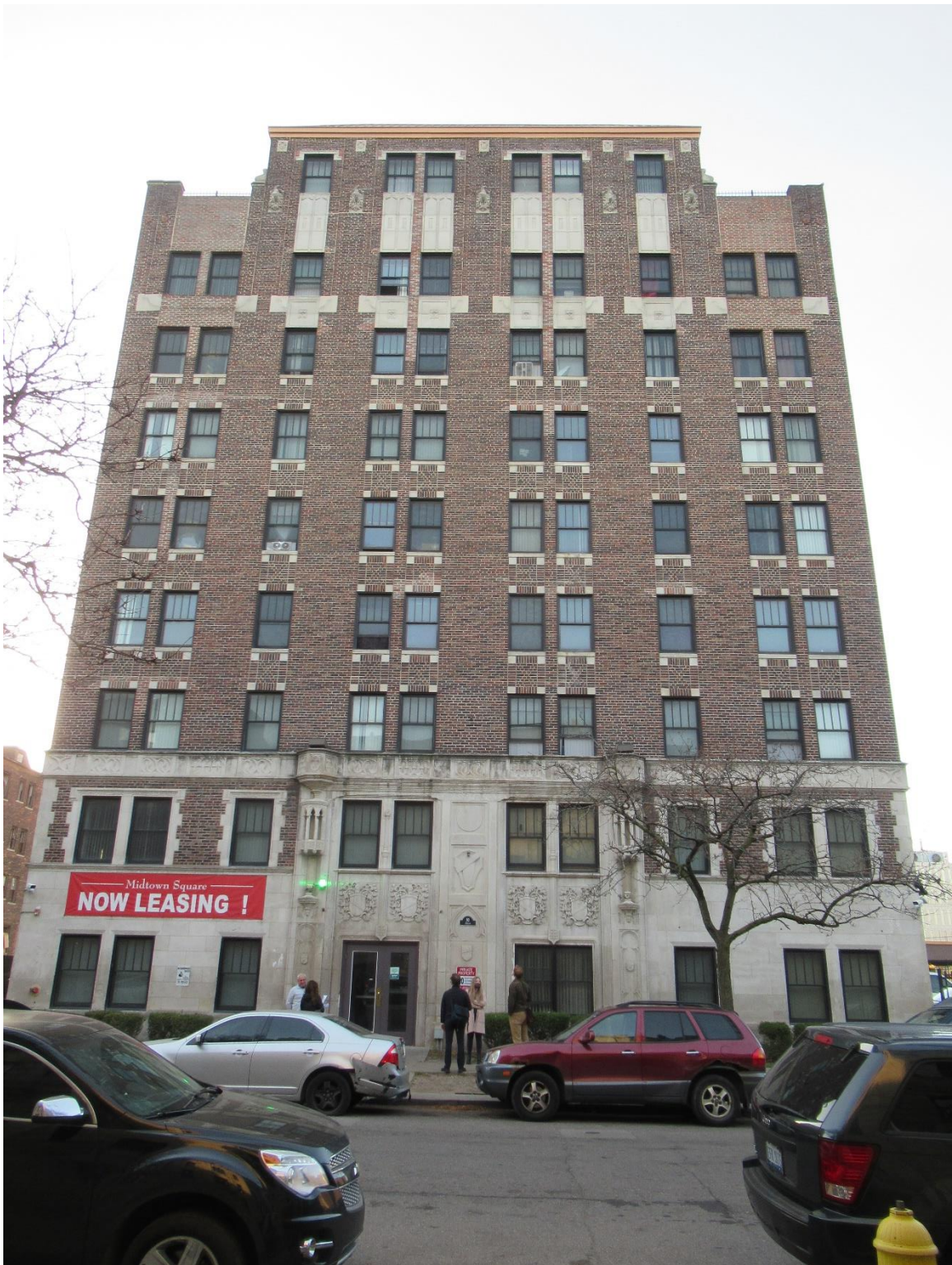
Figure #1: Exterior, Looking South. 11/6/20
