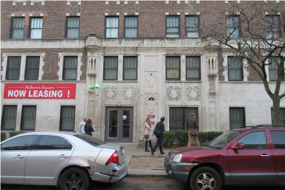
Figure #2: Exterior, Looking South. 11/6/20
