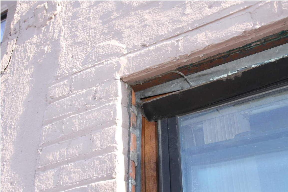
Figure #39: Exterior, Window, Looking Up. 11/18/20
