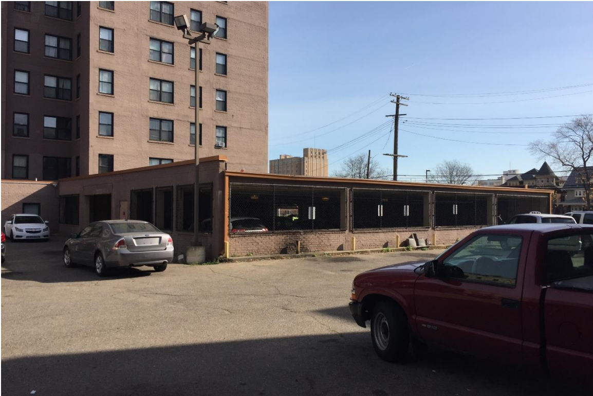
Figure #11: Exterior, Garage, Looking East. 11/6/20
