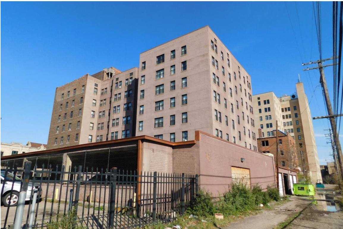
Figure #31: Exterior, Looking Northeast. 11/18/20
