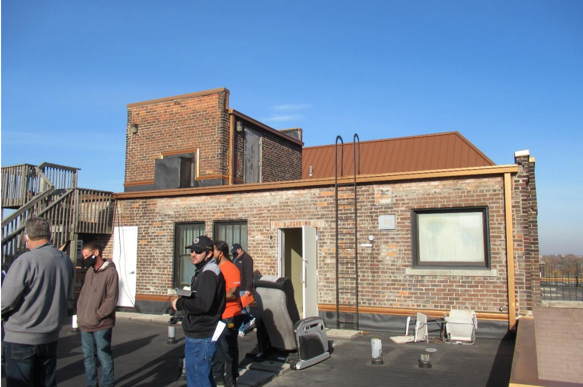
Figure #43: Exterior, Roof, Looking North. 11/6/20
