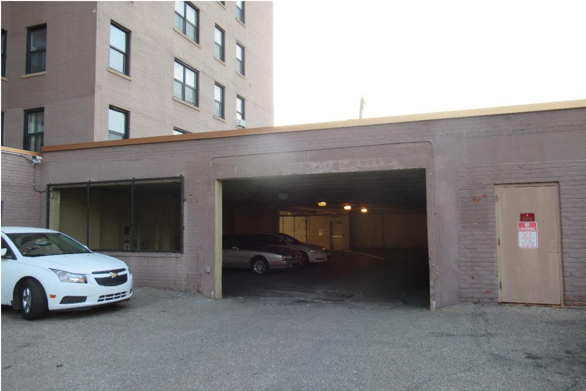
Figure #13: Exterior, Garage, Looking South. 11/6/20
