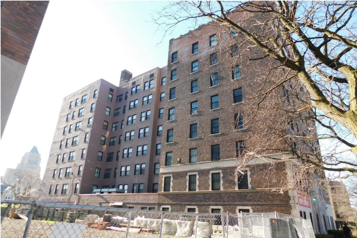
Figure #20: Exterior, Looking West. 11/18/20
