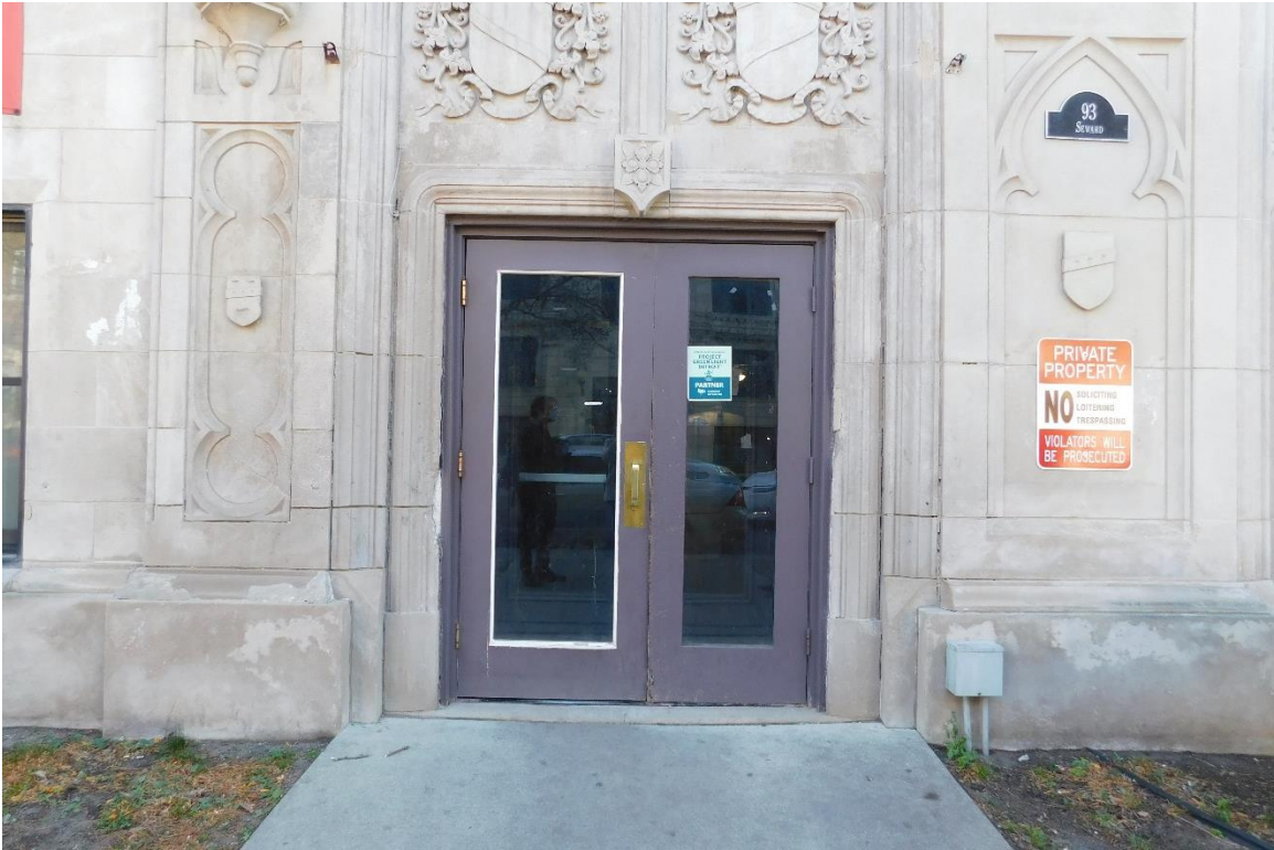
Figure #4: Exterior, Main Doors, Looking South. 11/18/20
