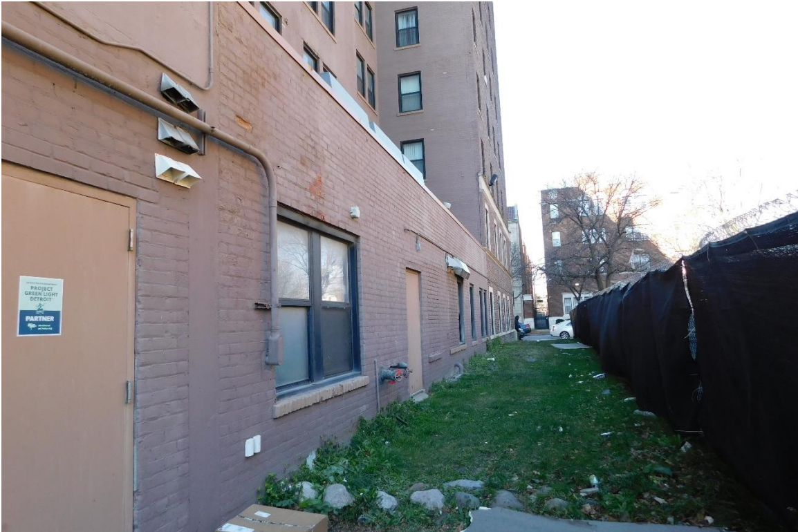
Figure #26: Exterior, looking North. 11/18/20
