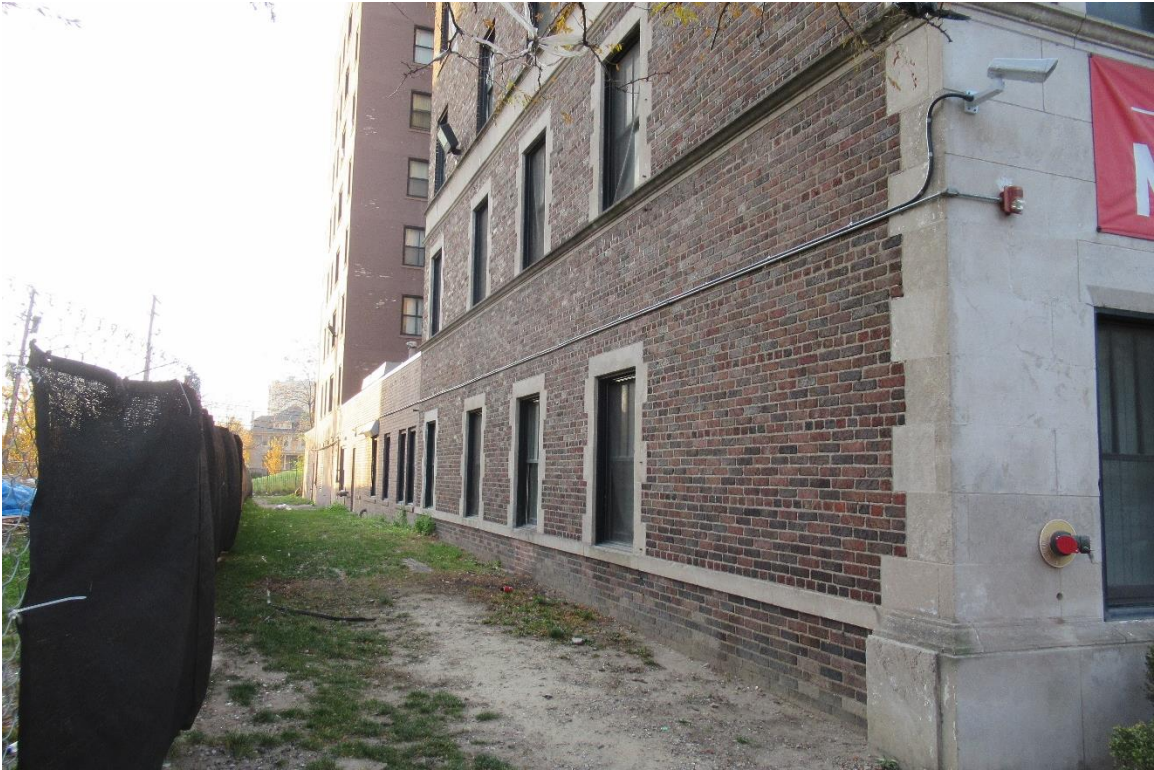
Figure #22: Exterior, Looking South. 11/18/20
