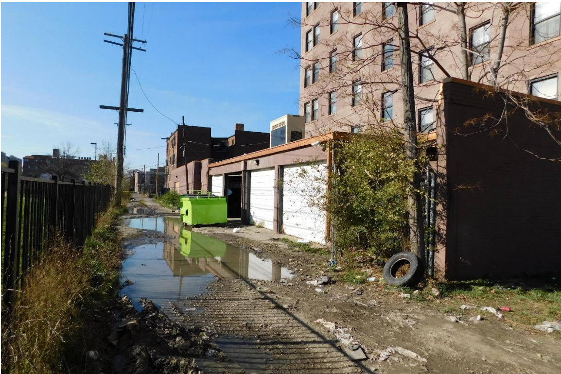
Figure #29: Exterior, Looking West. 11/20/18
