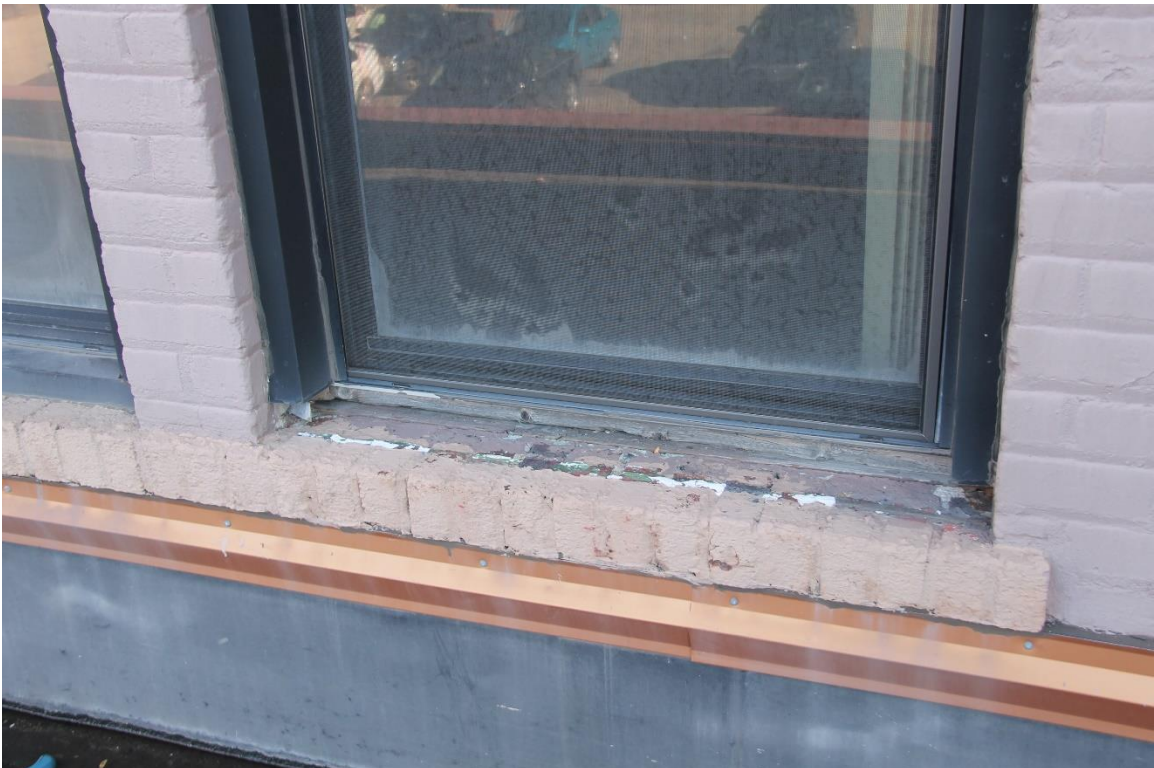
Figure #38: Exterior, Window, Looking Down. 11/18/20
