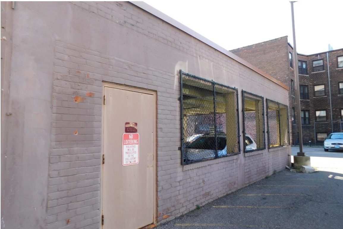
Figure #14: Exterior, Garage, Looking Southwest. 11/18/20
