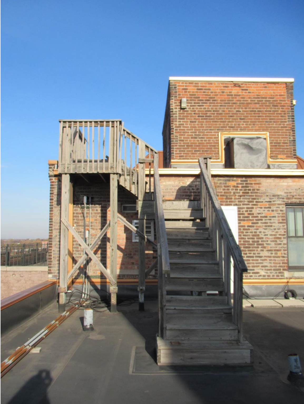
Figure #49: Exterior, Roof, Looking North. 11/6/20
