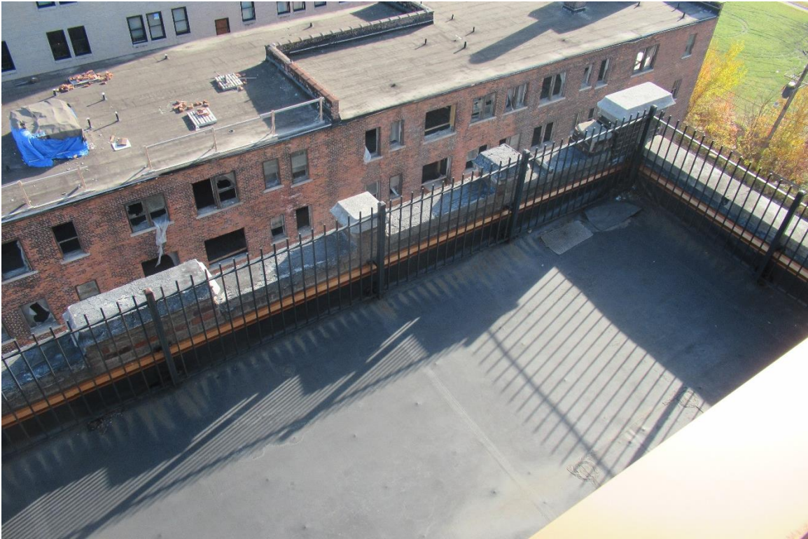
Figure #52: Exterior, Penthouse Patio (East), Looking Down. 11/6/20
