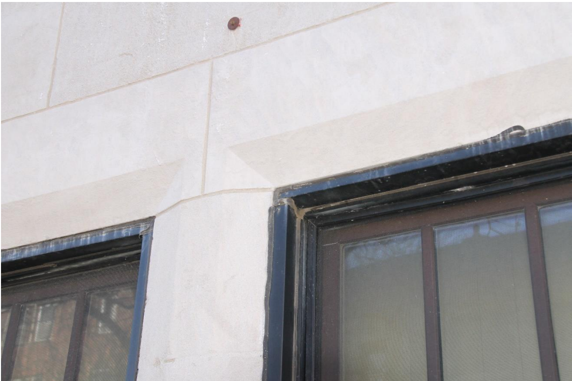
Figure #36: Exterior, Window, Looking Up. 11/18/20
