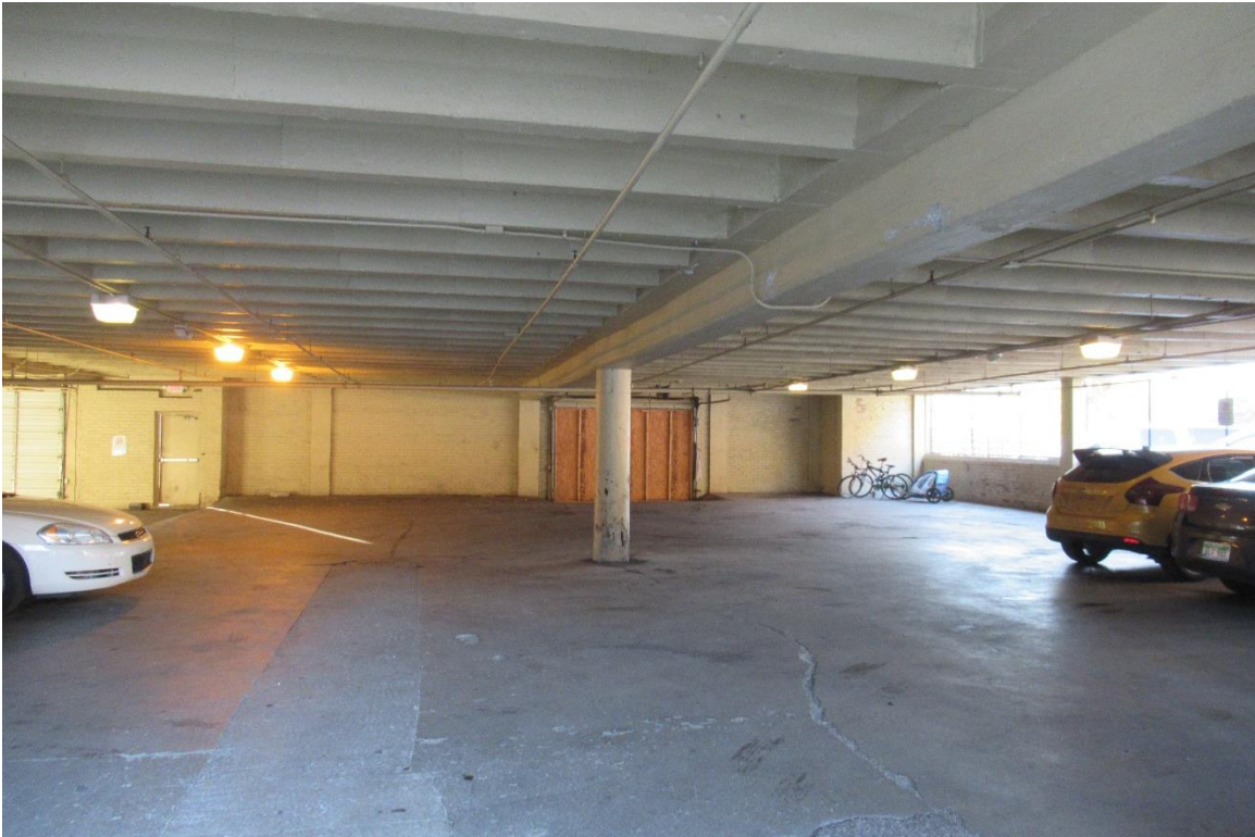
Figure #15: Garage, Looking South. 11/6/20
