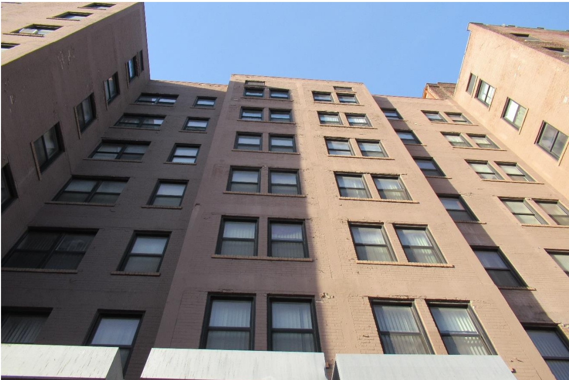
Figure #21: Exterior, East façade, Looking up. 11/6/20
