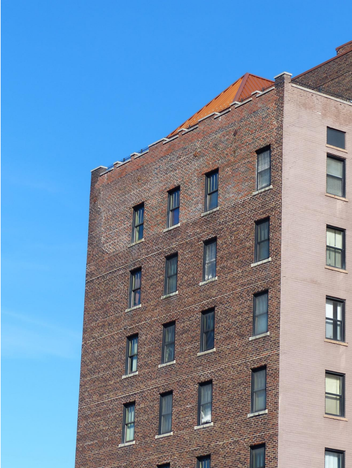
Figure #10: Exterior, Looking North. 11/18/20
