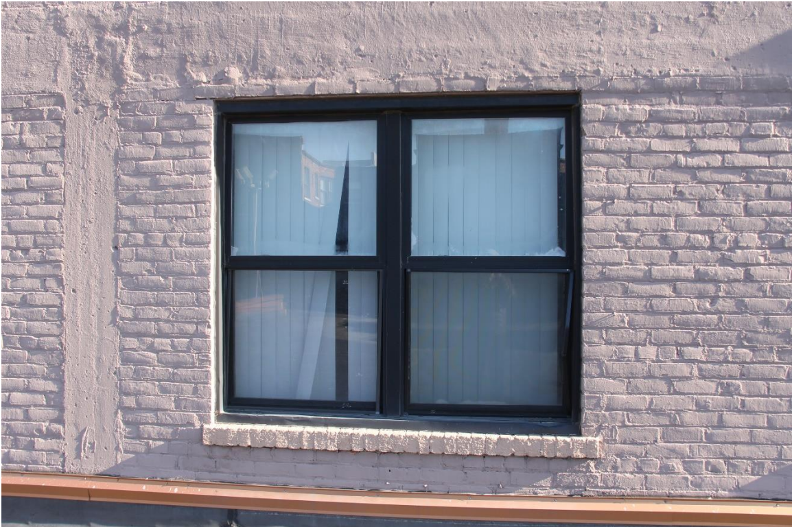
Figure #37: Exterior, Window, Looking East, 11/18/20
