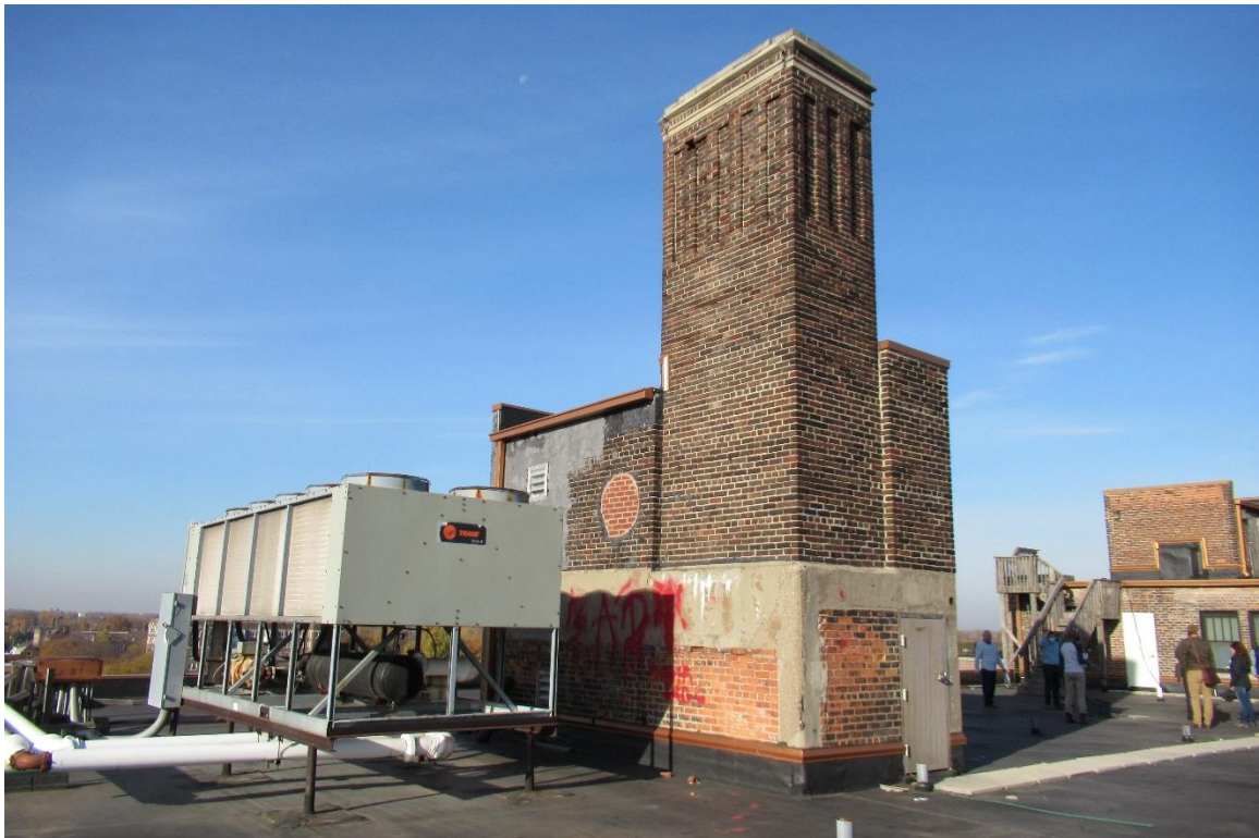
Figure #42: Exterior, Roof, Looking Northwest. 11/6/20
