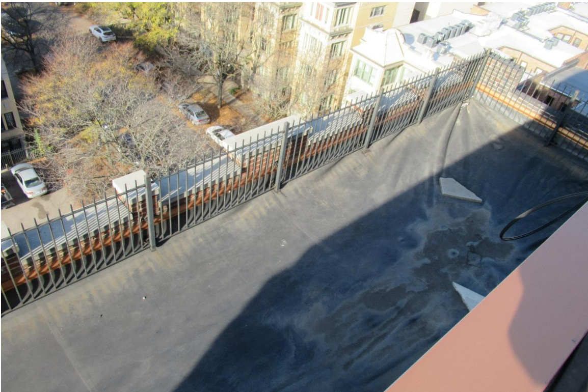
Figure #51: Exterior, Penthouse Patio (West), Looking Down. 11/6/20
