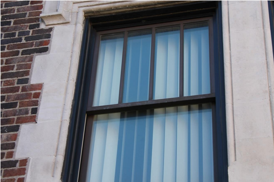
Figure #35: Exterior, Window, Looking Up. 11/18/20
