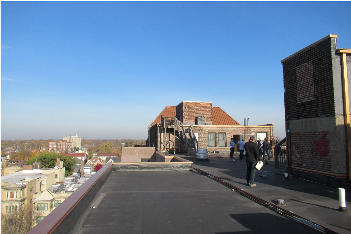
Figure #44: Exterior, Roof, Looking North. 11/6/20
