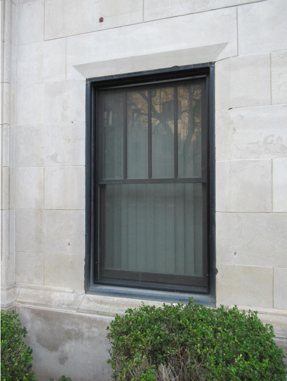
Figure #34: Exterior, Window, Looking South. 11/6/20
