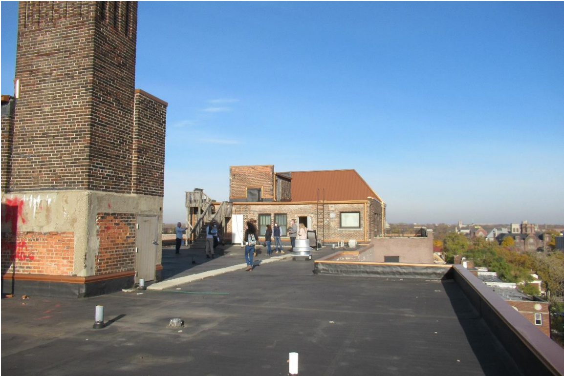
Figure #45: Exterior, Roof, Looking North. 11/6/20
