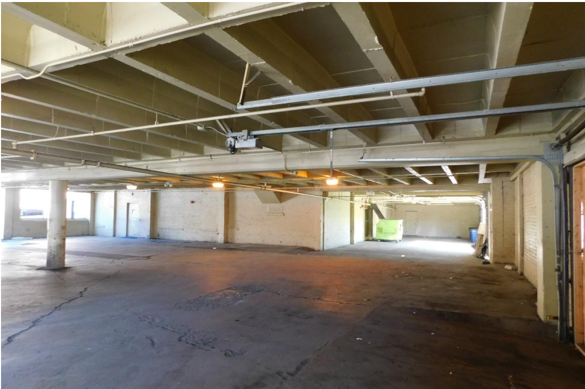
Figure #18: Garage, Looking East. 11/18/20
