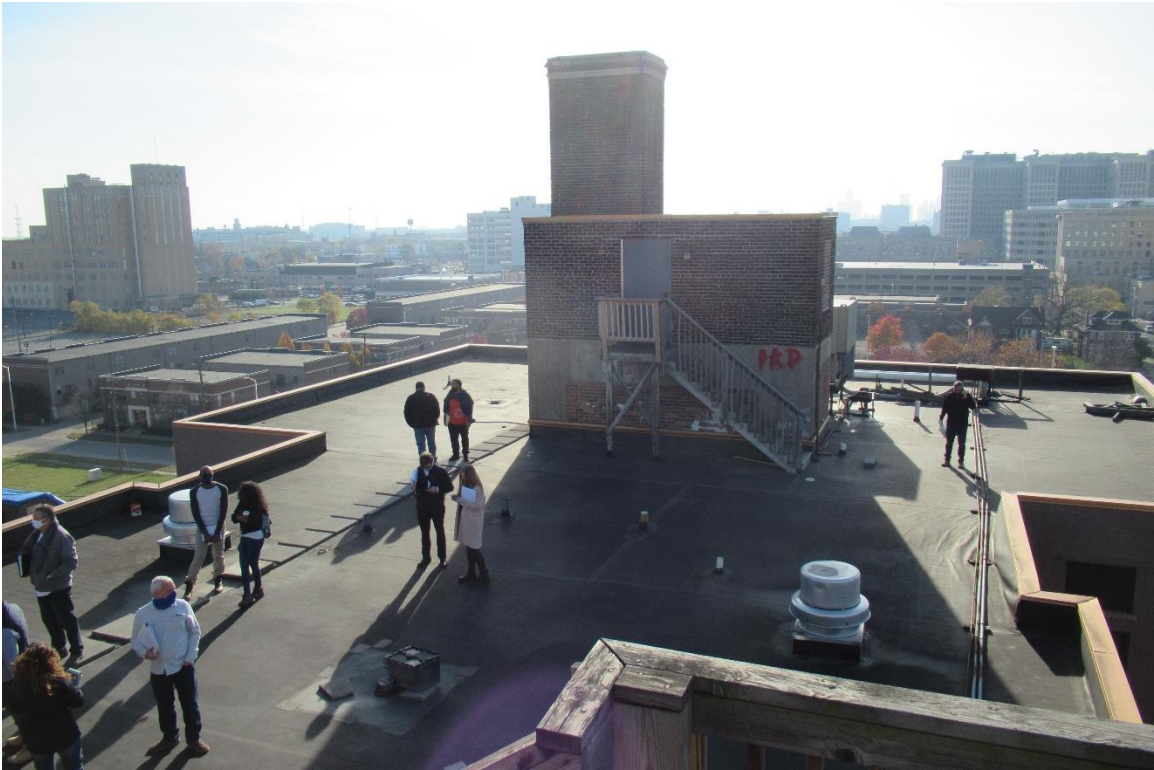
Figure #47: Exterior, Roof, Looking South. 11/6/20
