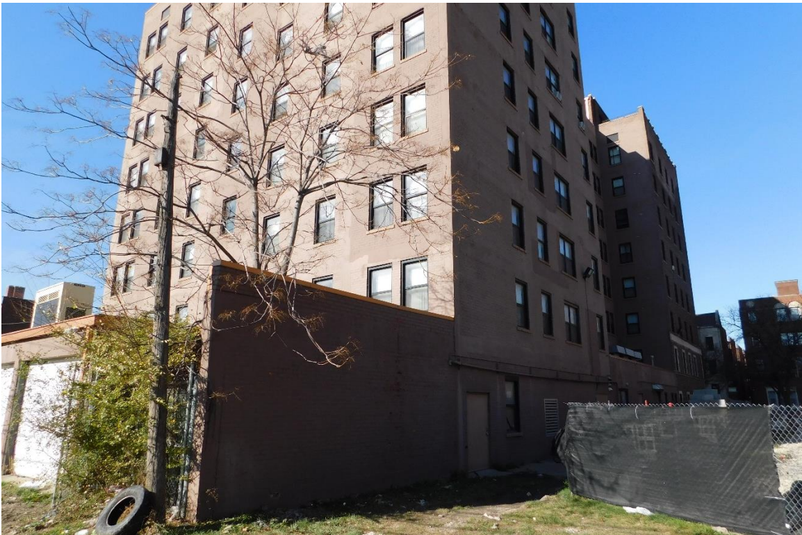
Figure #27: Exterior, looking Northwest. 11/18/20
