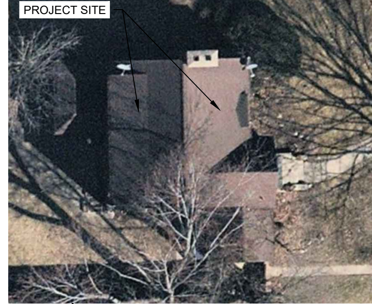
2 HOUSE PHOTO PV-1 | SCALE: NTS
