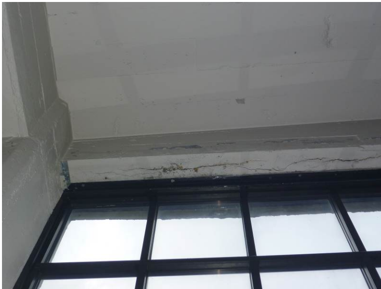
Photo No. 7 – Unit 400
