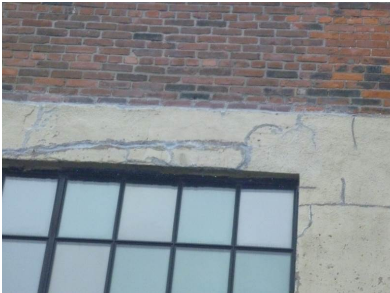
Photo No. 9 – Exterior above Unit 400
