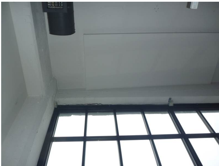
Photo No. 2 – Unit 300
