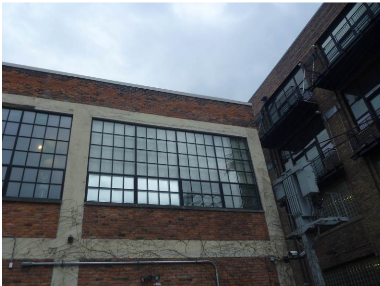
Photo No. 12 – Exterior Unit 700
