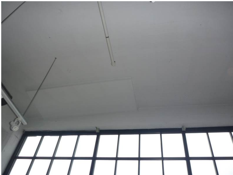
Photo No. 1 – Unit 300
