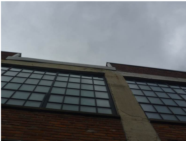
Photo No. 4 – Exterior above Unit 300
