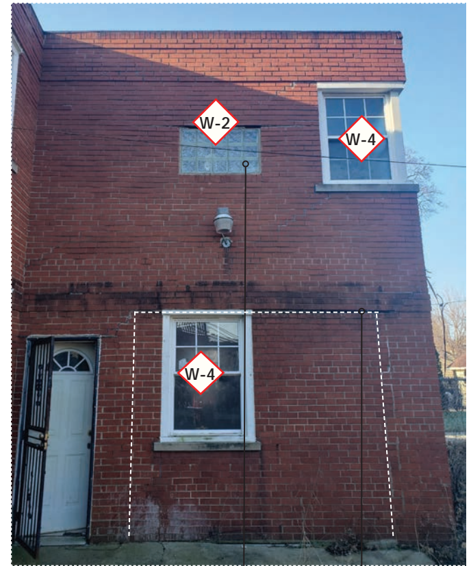
Fig. 1 | East Facade (Former Garage)
