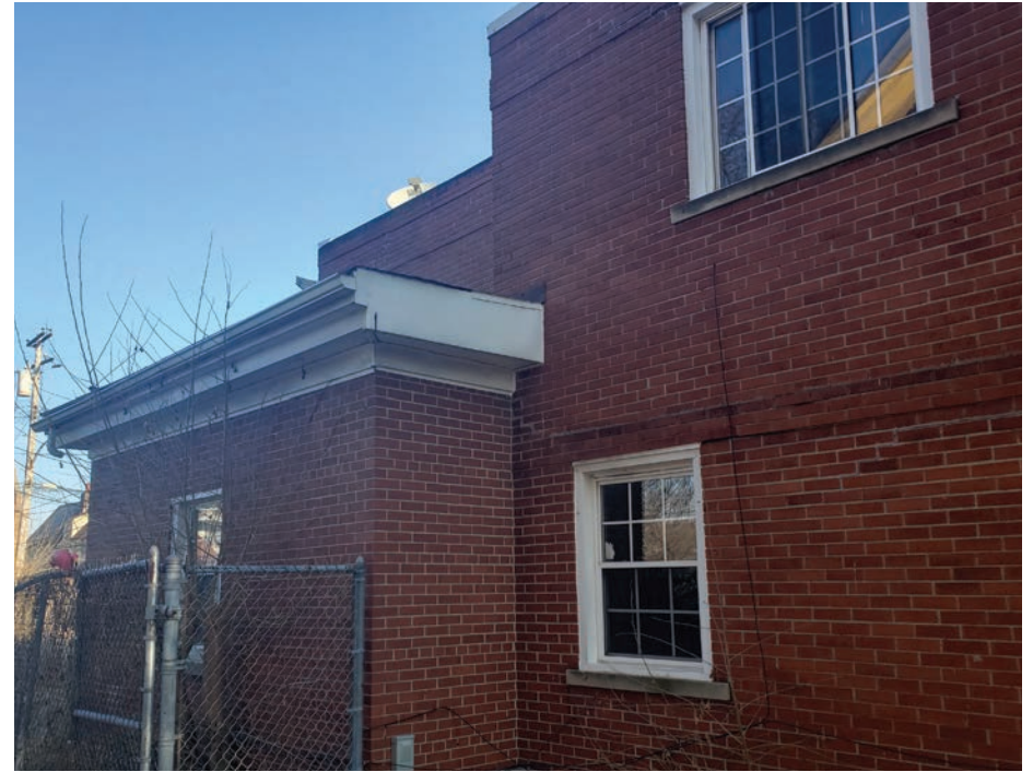
Fig. 14 | The sideyard of 1948 Chicago Blvd. -West Elevation
