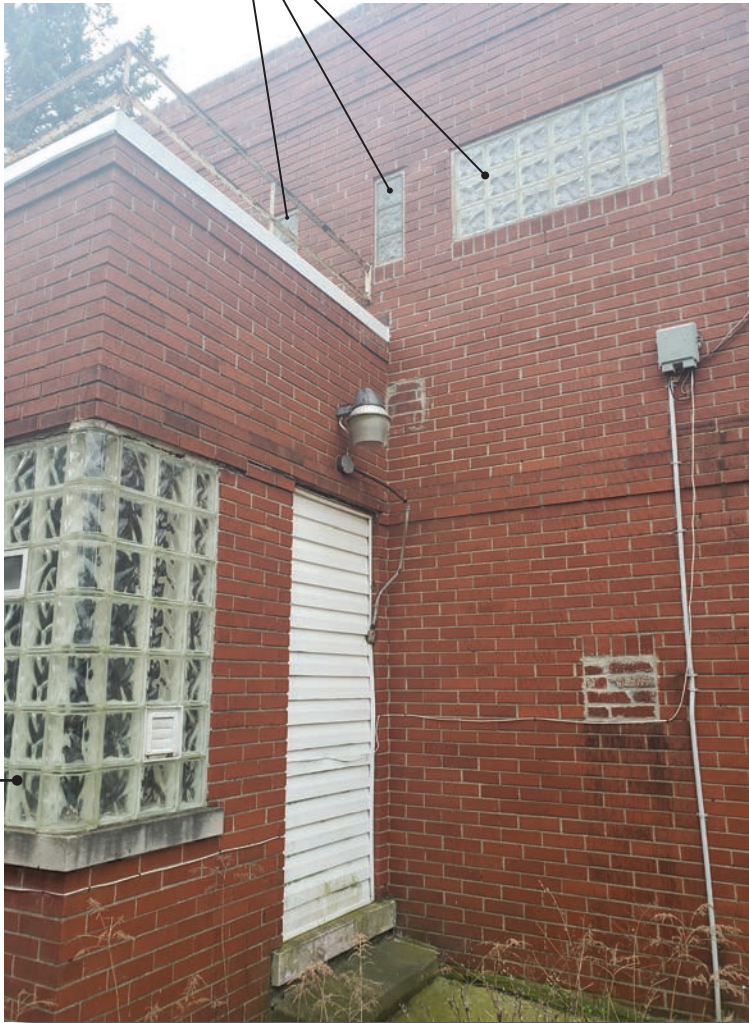
Fig. 2 | Looking SW at East Facade (Former Rear Entry)
