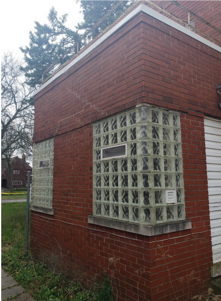
Fig. 3A | Today, the windows have been replaced with glass block. See window type (W-3) for more informaton
