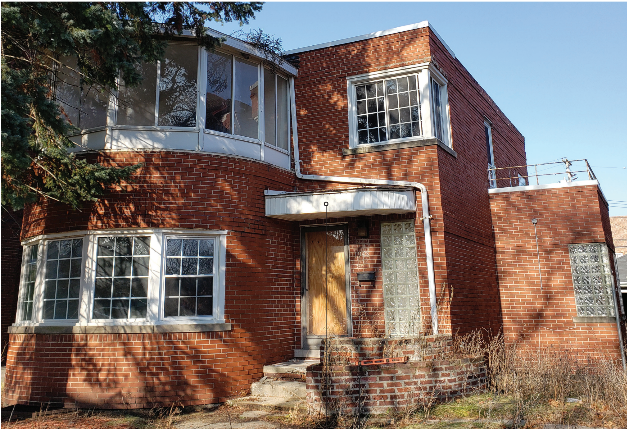
Fig. 6 / South Facade (Street View). See 1974 and 1980 Historic Photos
