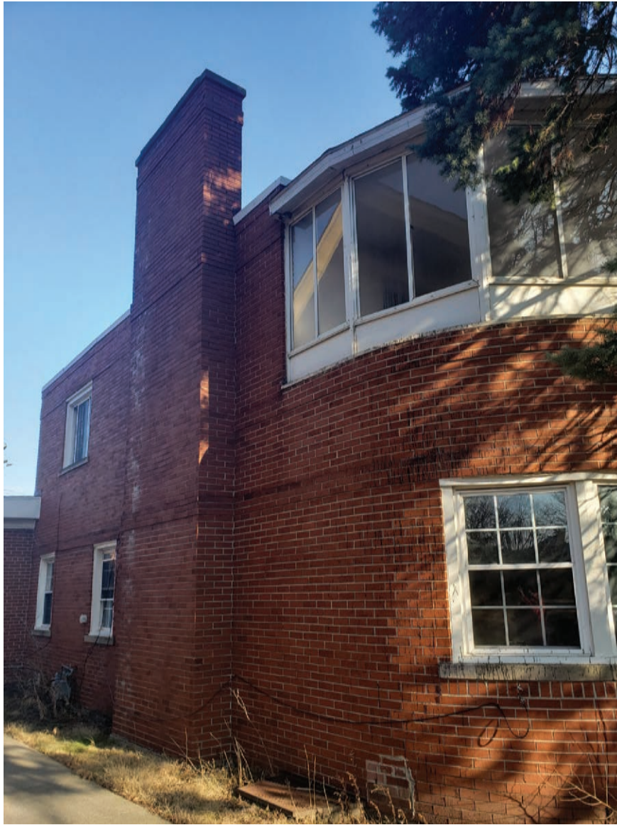
Fig. 13 | The sideyard of 1948 Chicago Blvd. -West Elevation
