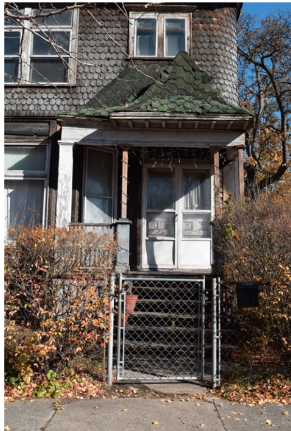
Front Porch (Southwest)
