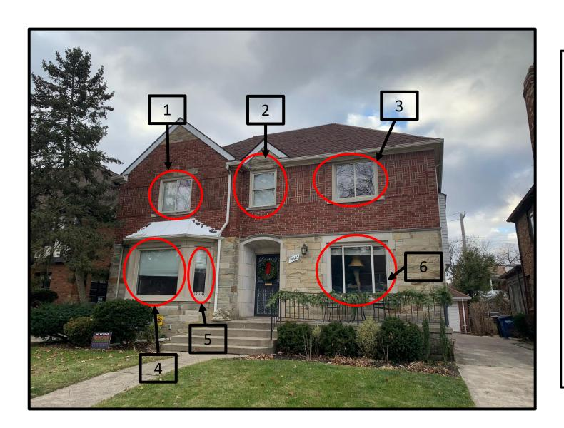
1 – Master Bedroom: Currently sliding without grid, putty color; caulked shut to prevent draft, seal broken causing condensation between panes
