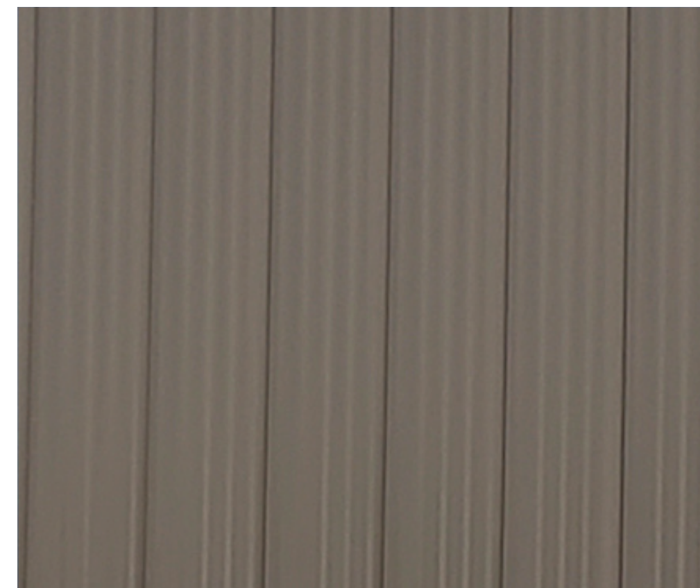
PAC CLAD STANDING SEAM SIDING R-36 PANEL, 24 GA STEEL COLOR: BURNISHED STEEL
