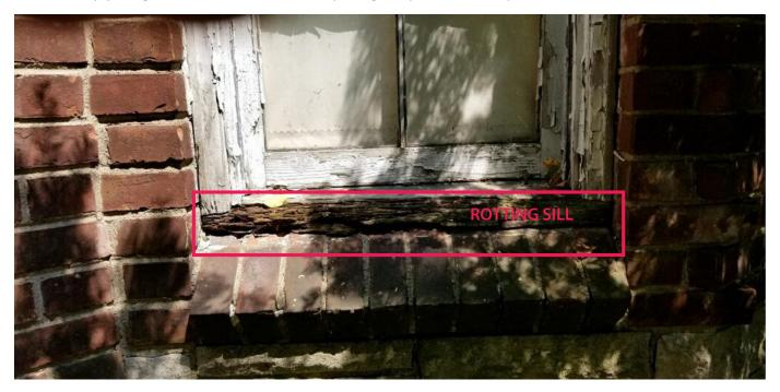
Window 3 is also suffering from the same things as the previous two windows. The sill is discolored from rot and there are cracks starting to form in it. A small section of the sash has broken off, which as we've seen in Window 1, can become a huge problem
