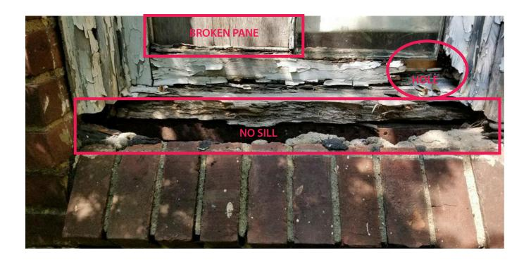
In Window 2, we can already see signs of the sill rotting away in the bottom left. The rot damage has already been so deeply integrated in to this wood that repairing this piece isn't an option.
