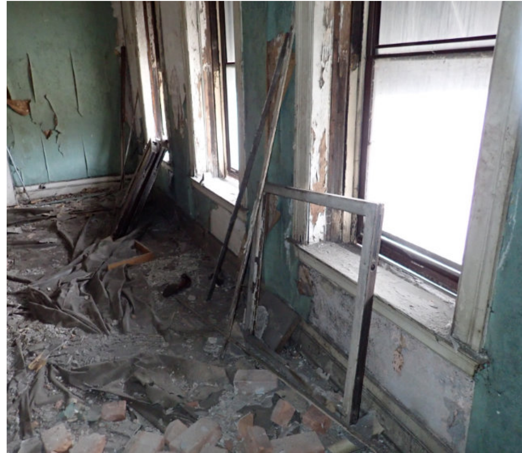
UNIT 203: REMOVED FRAMES AND STOPS
