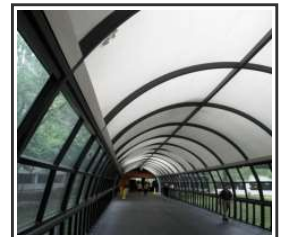
WEATHER PROTECTION ENCLOSURE
