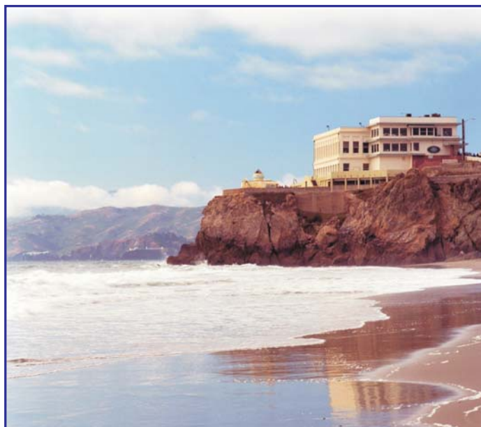
PHOTO: EverKote 300 was applied to this Historic Landmark building as part of the building's restoration program.
