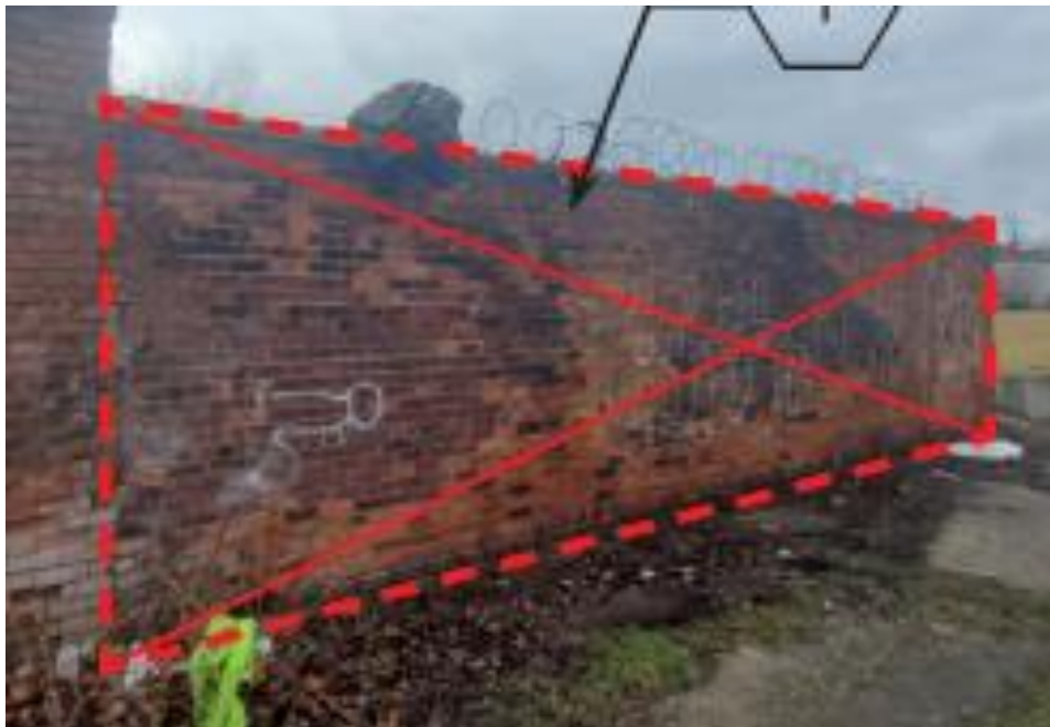
Photograph 3: East Masonry Wing Wall - North
