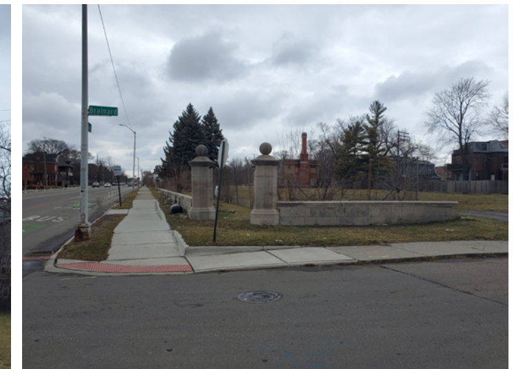
EXISTING STONE WALL AND DECORATIVE COLUMNS
