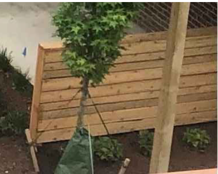
4' ht. Screen Fence - Alternate Natural Finish (For use between select buildings and as AC Unit screens)
