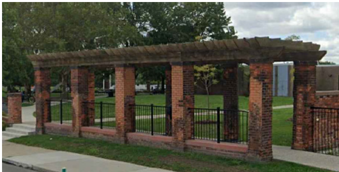
Decorative Trellis Structure (Potentially matching Scripps Park, or similar)
