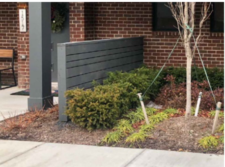
4' ht. Screen Fence - Color to match Architecture (For use between select buildings and as AC Unit screens)
