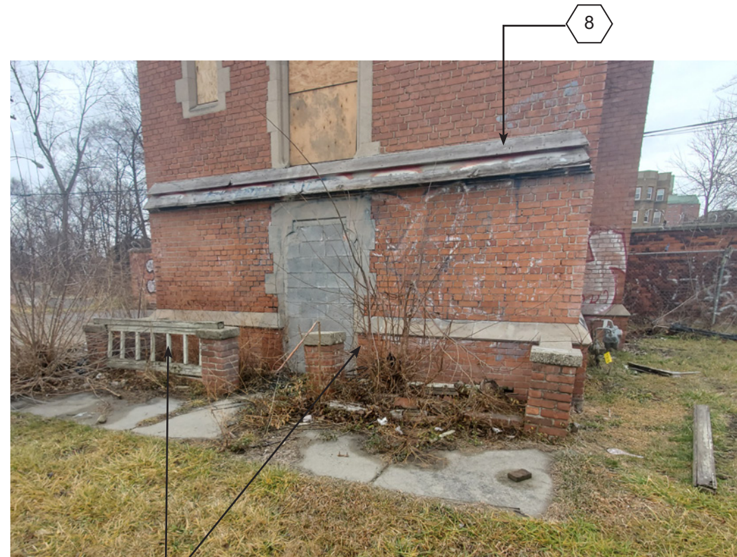
FRONT PORCH DETAIL
