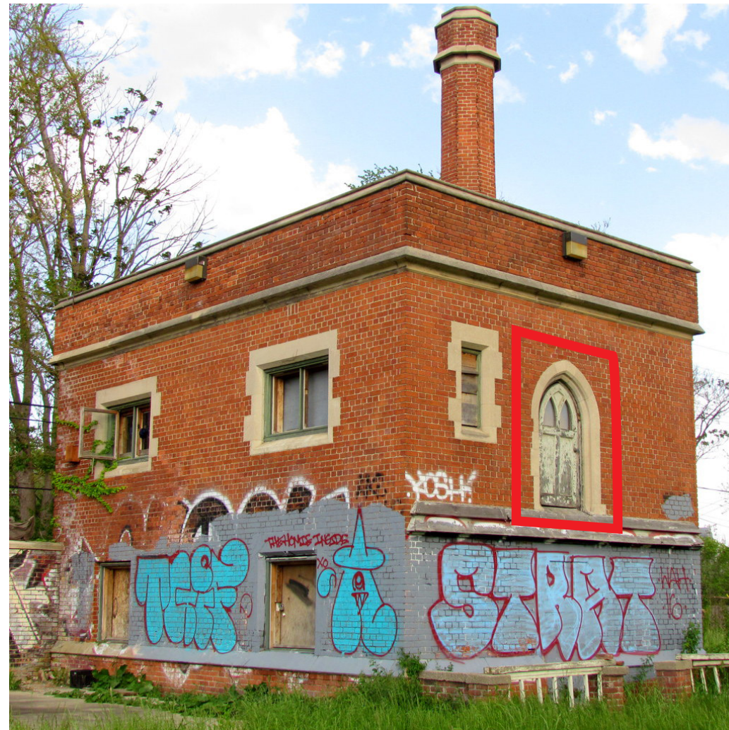
POWER HOUSE PRE-FIRE
