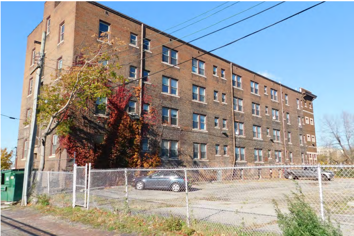
Figure #16: Exterior, East Façade, Looking Northwest. 10/28/20
