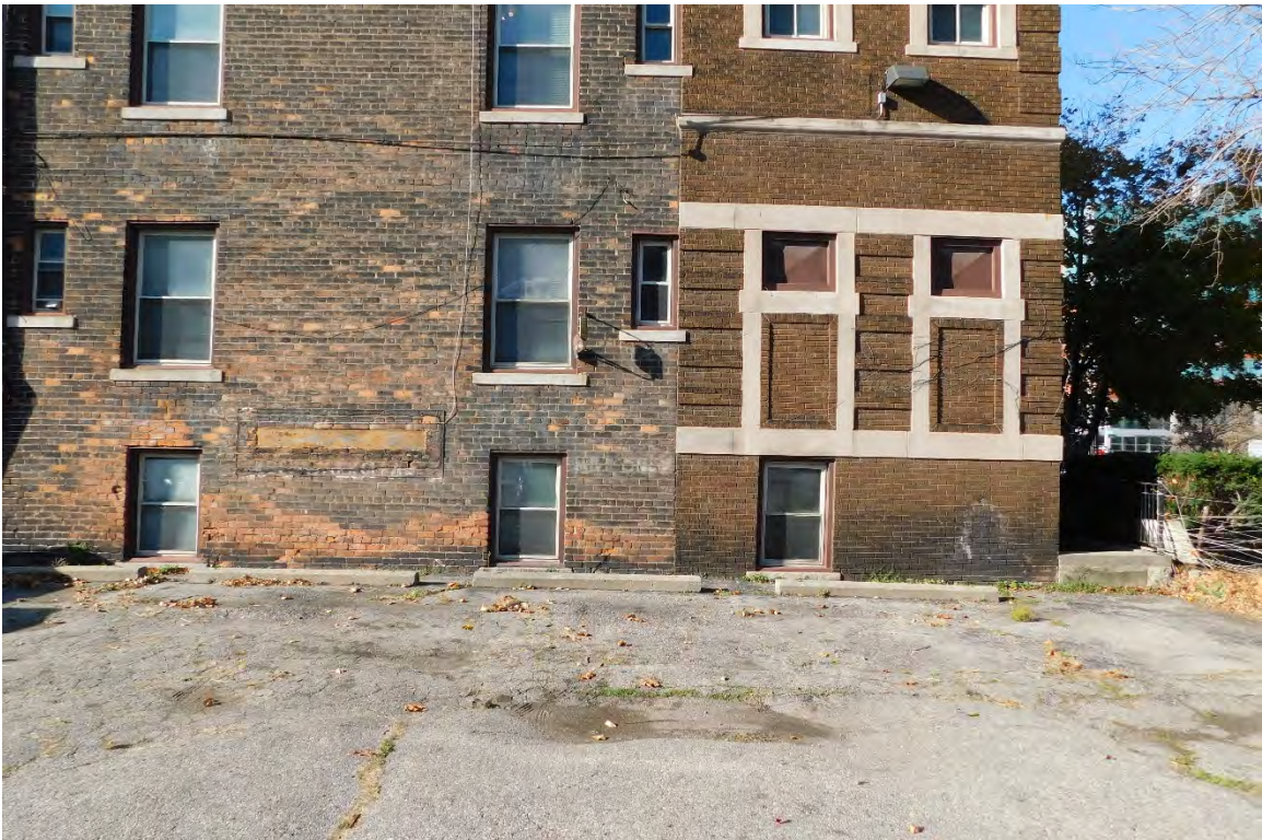
Figure #11: Exterior, East Façade, Looking West. 10/28/20
