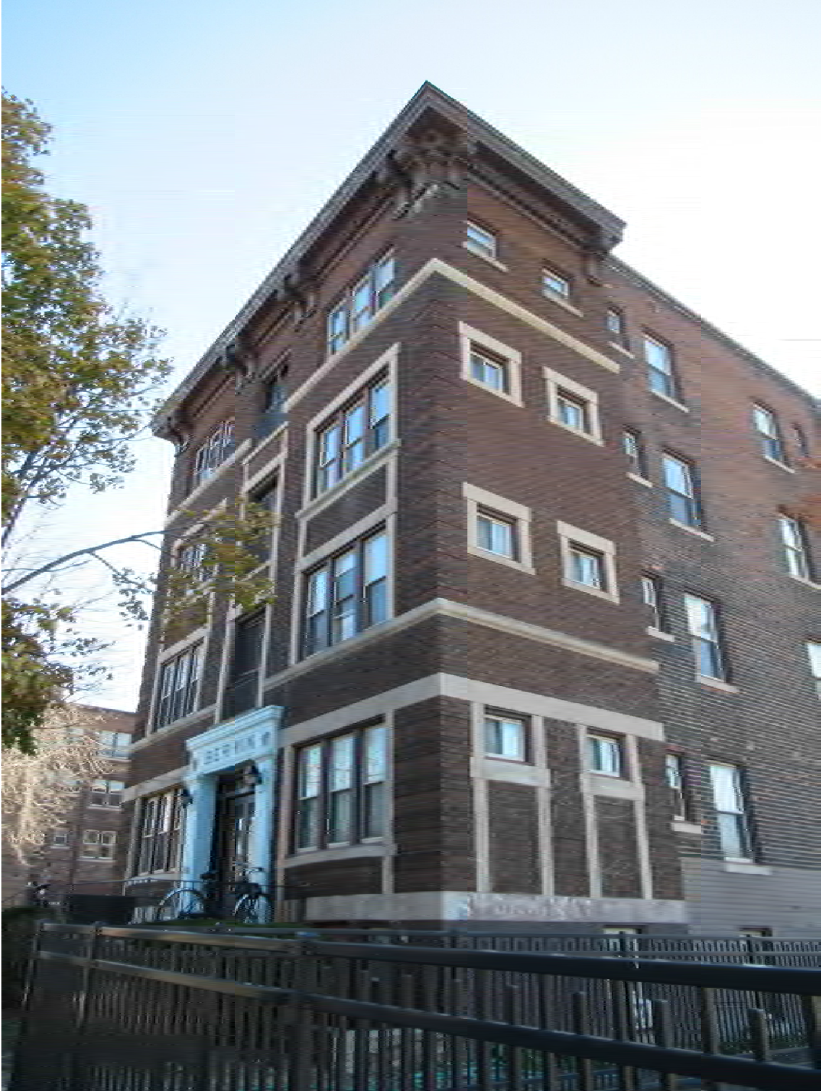
Figure #01: Exterior, North and West Facades, Looking Southeast. 10/28/20
