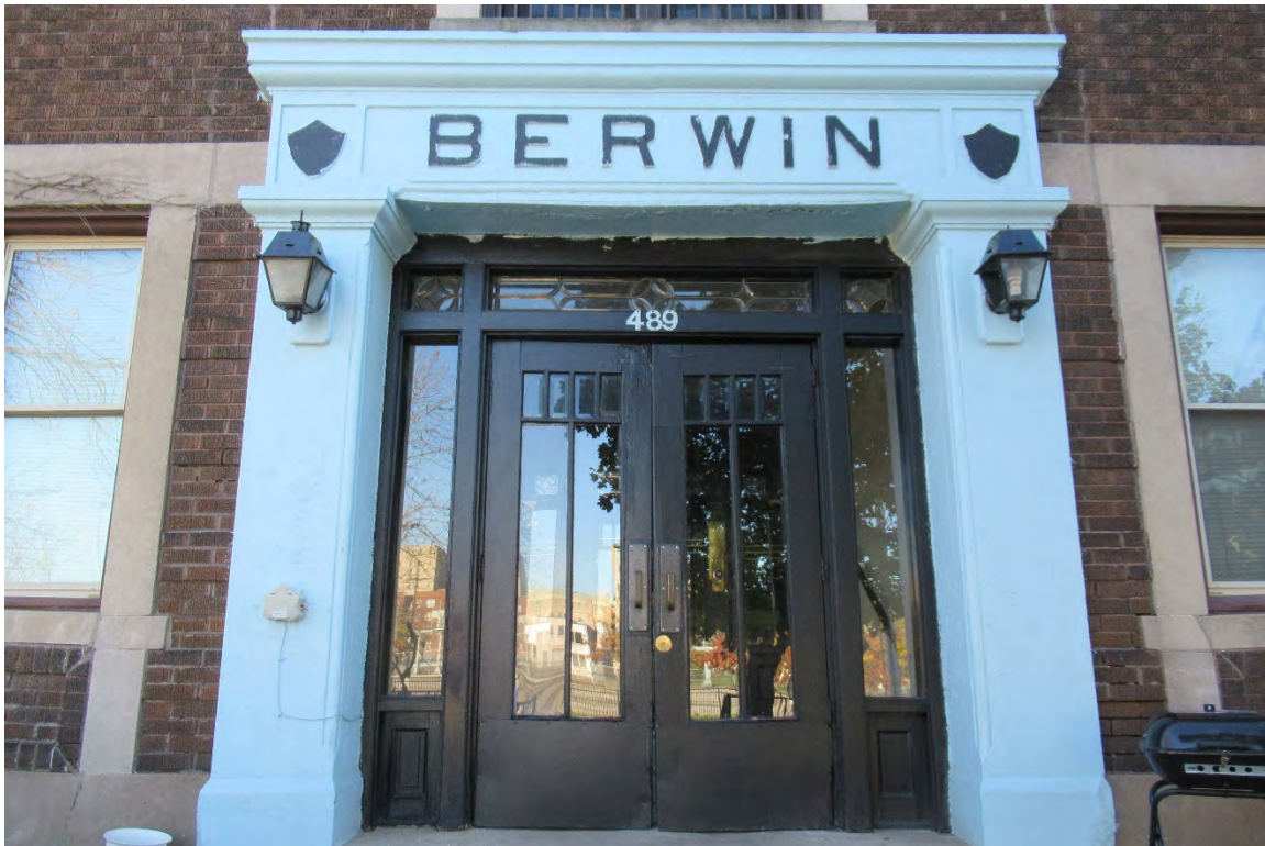
Figure #08: Exterior, North Façade, Looking South. 10/28/20
