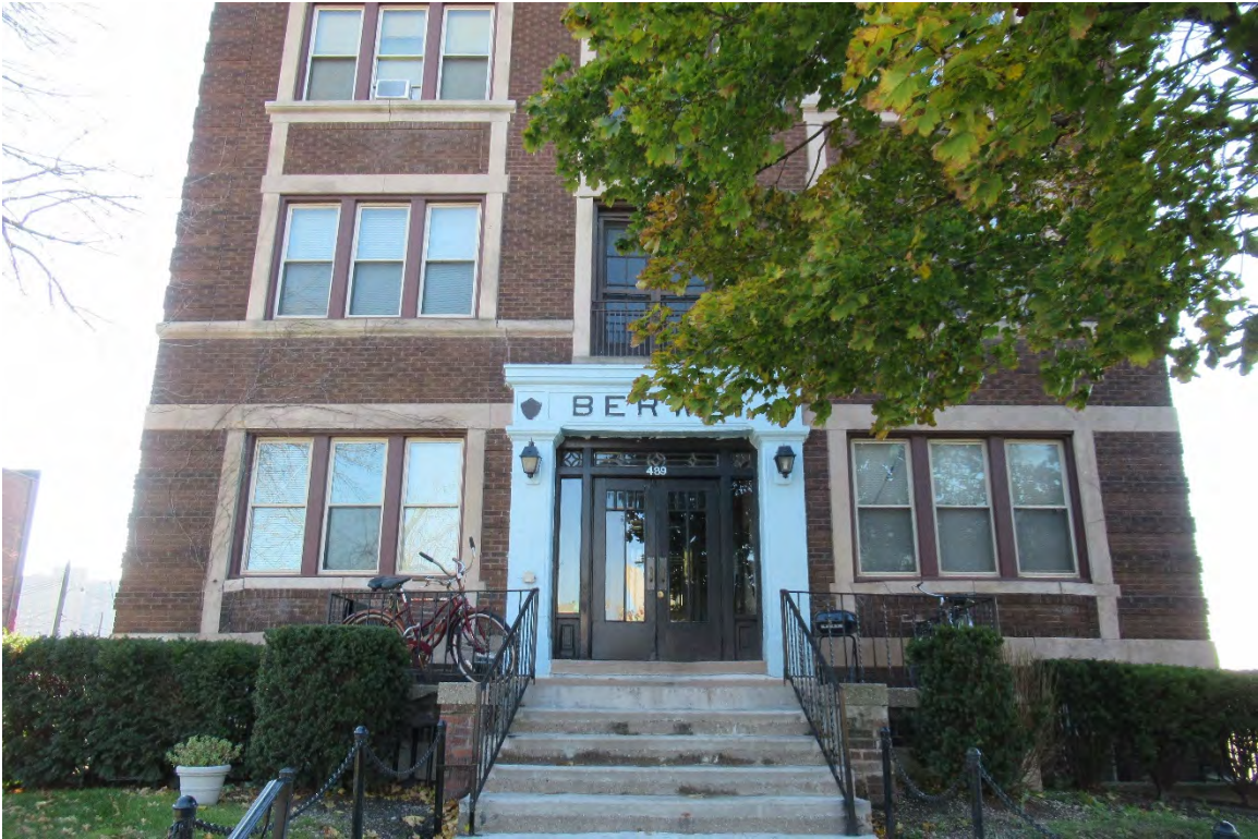
Figure #02: Exterior, North Façade, Looking South. 10/28/20
