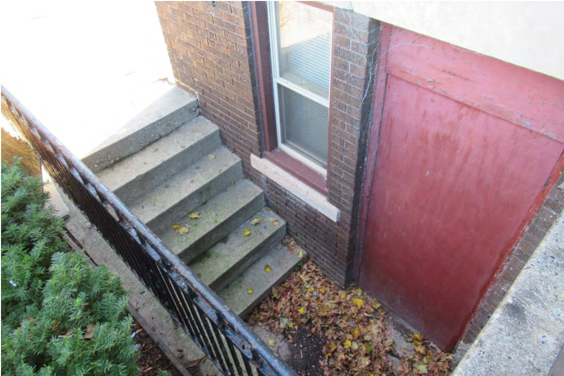
Figure #04: Exterior, North Façade, Looking Down. 10/28/20
