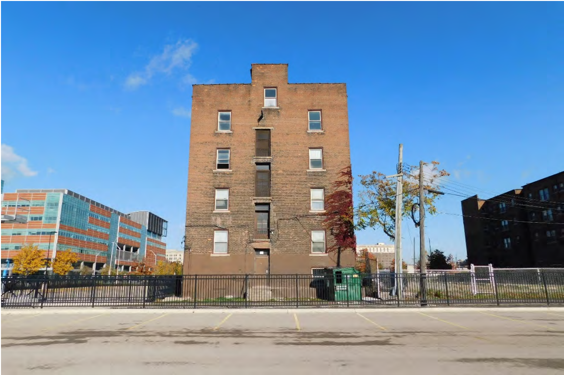
Figure #18: Exterior, South Façade, Looking North. 10/28/20
