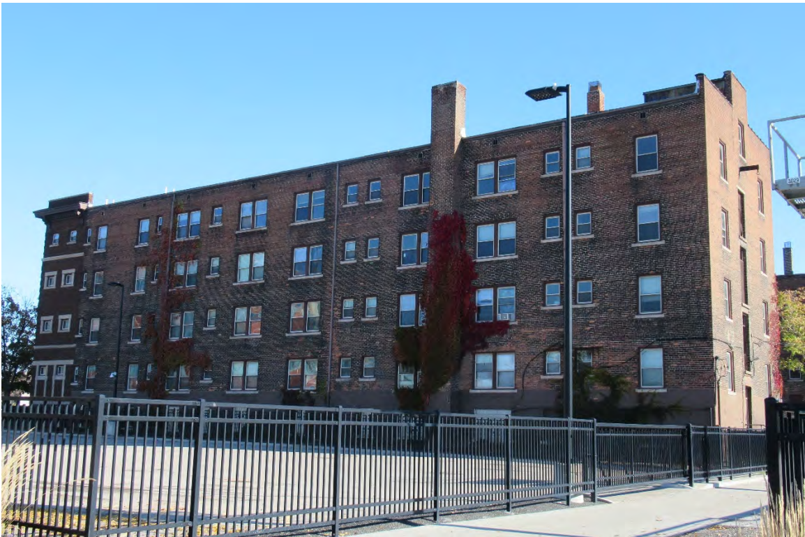
Figure #07: Exterior, West Façade, Looking Northeast. 10/28/20
