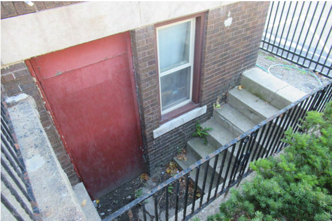
Figure #05: Exterior, North Façade, Looking Down. 10/28/20
