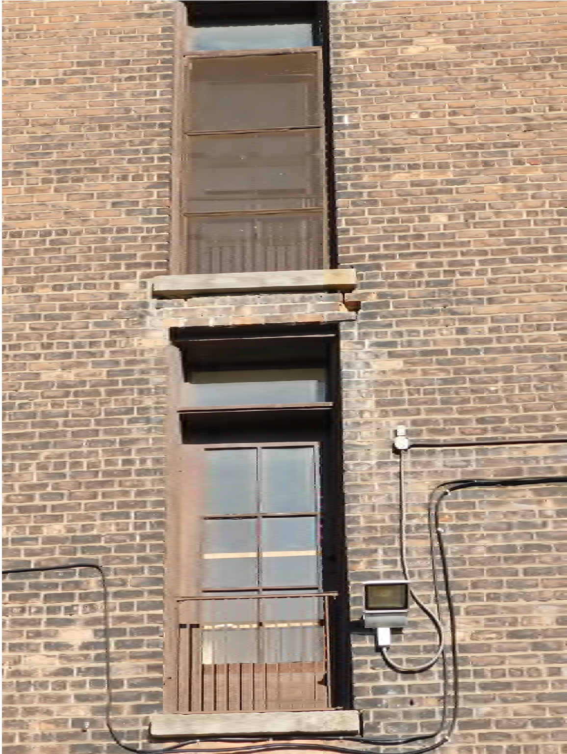
Figure #17: Exterior, South Façade, Looking Up. 10/28/20
