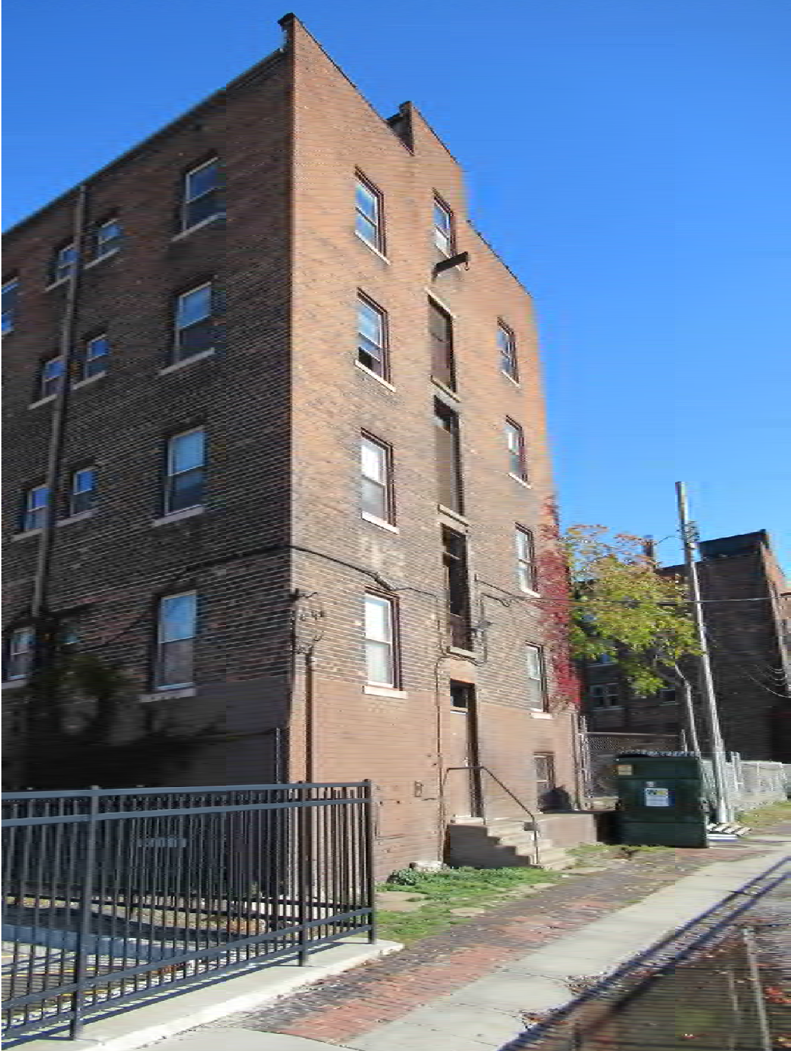
Figure #14: Exterior, West and South Facades, Looking Northeast. 10/28/20
