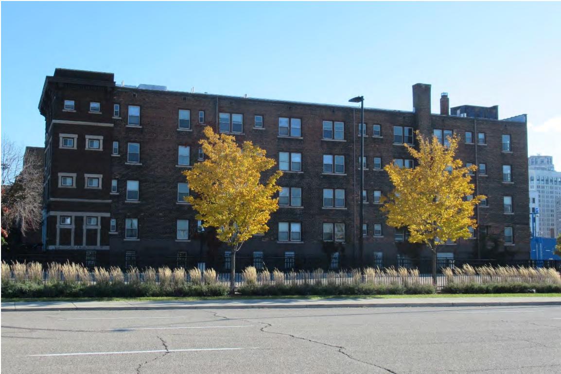
Figure #06: Exterior, West Façade, Looking East. 10/28/20
