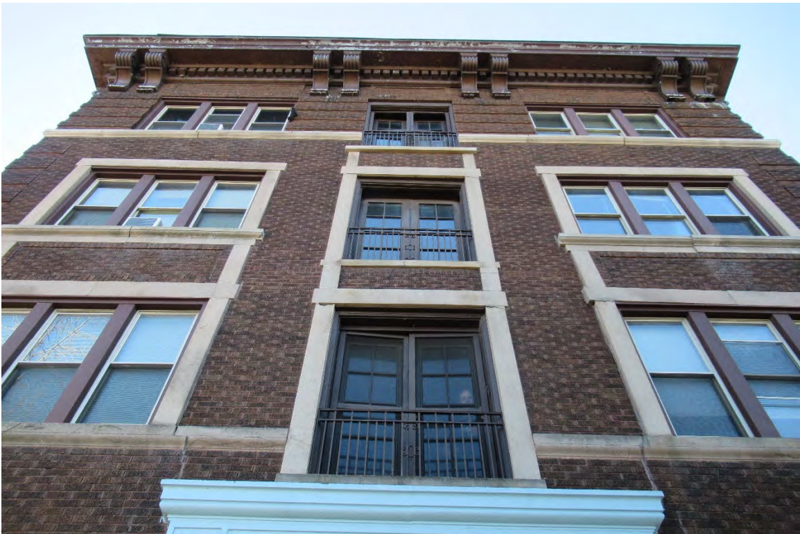
Figure #03: Exterior, North Façade, Looking Up. 10/28/20
