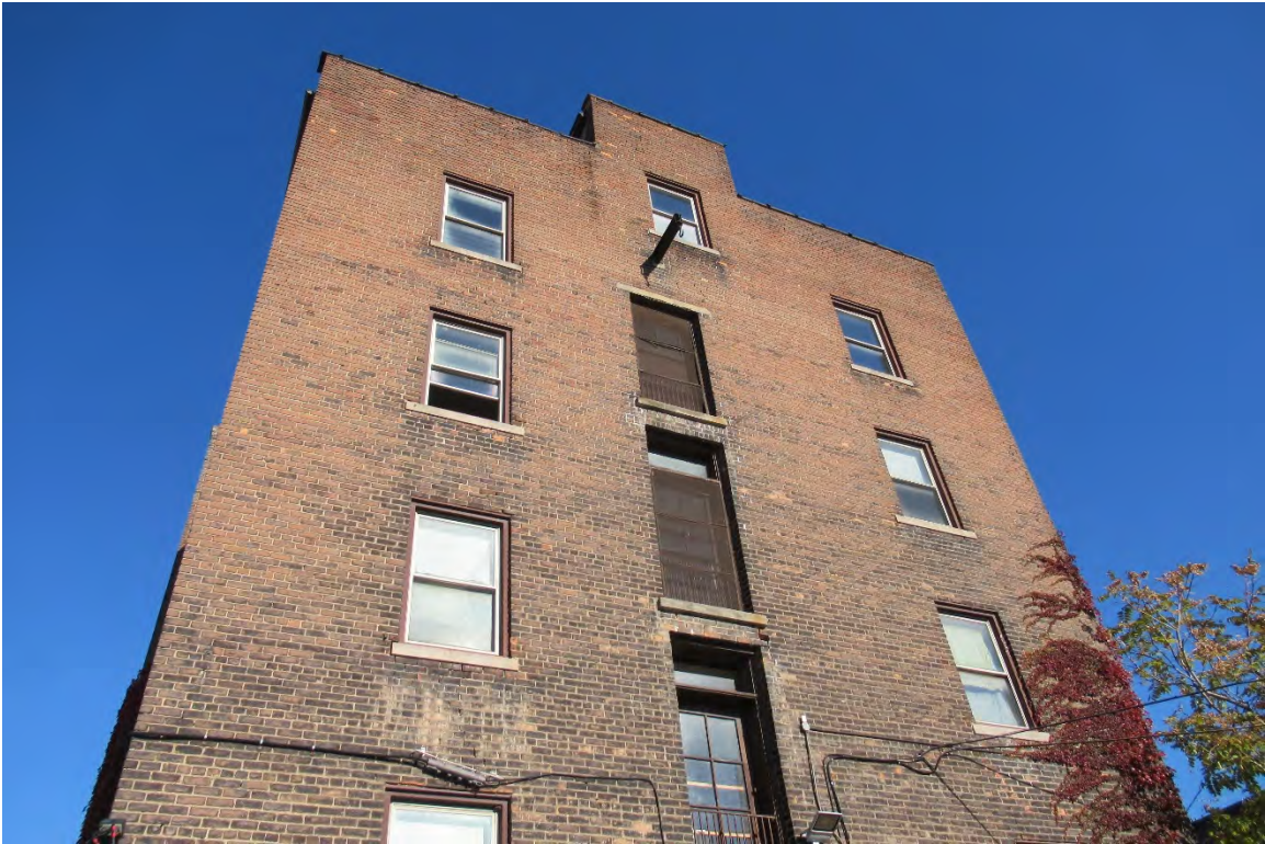
Figure #15: Exterior, South Façade, Looking Up. 10/28/20
