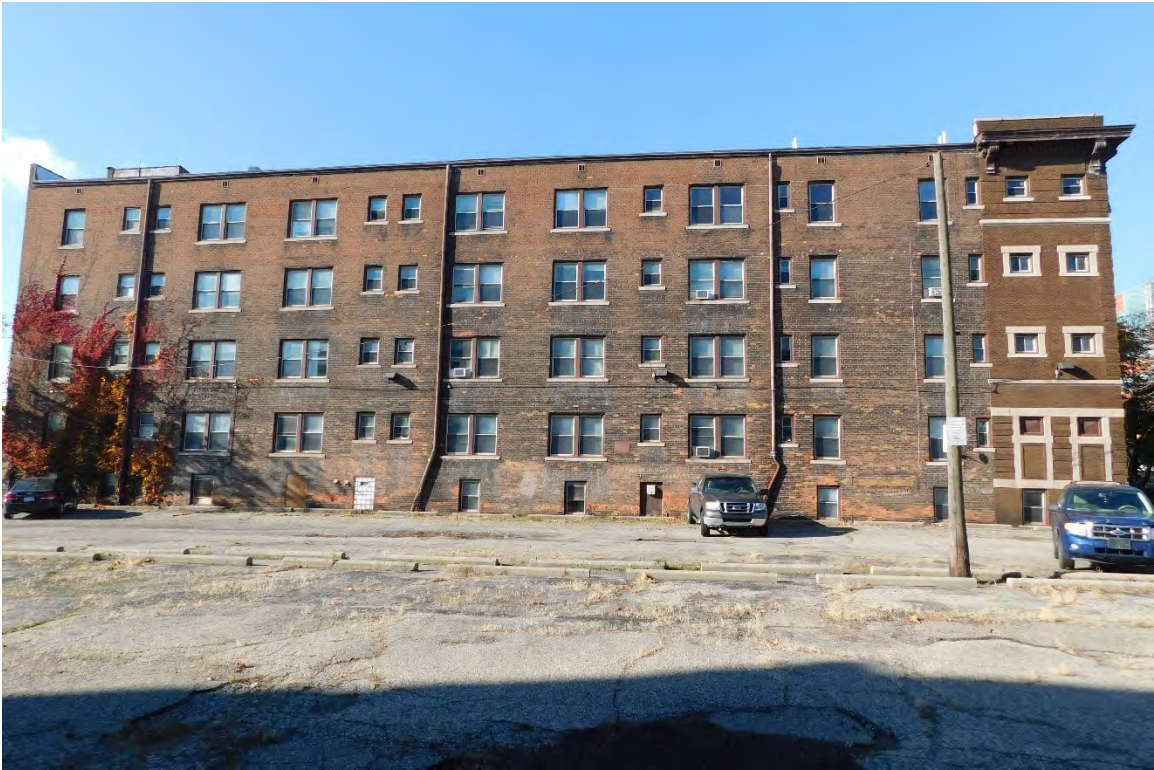
Figure #12: Exterior, East Façade, Looking West. 10/28/20
