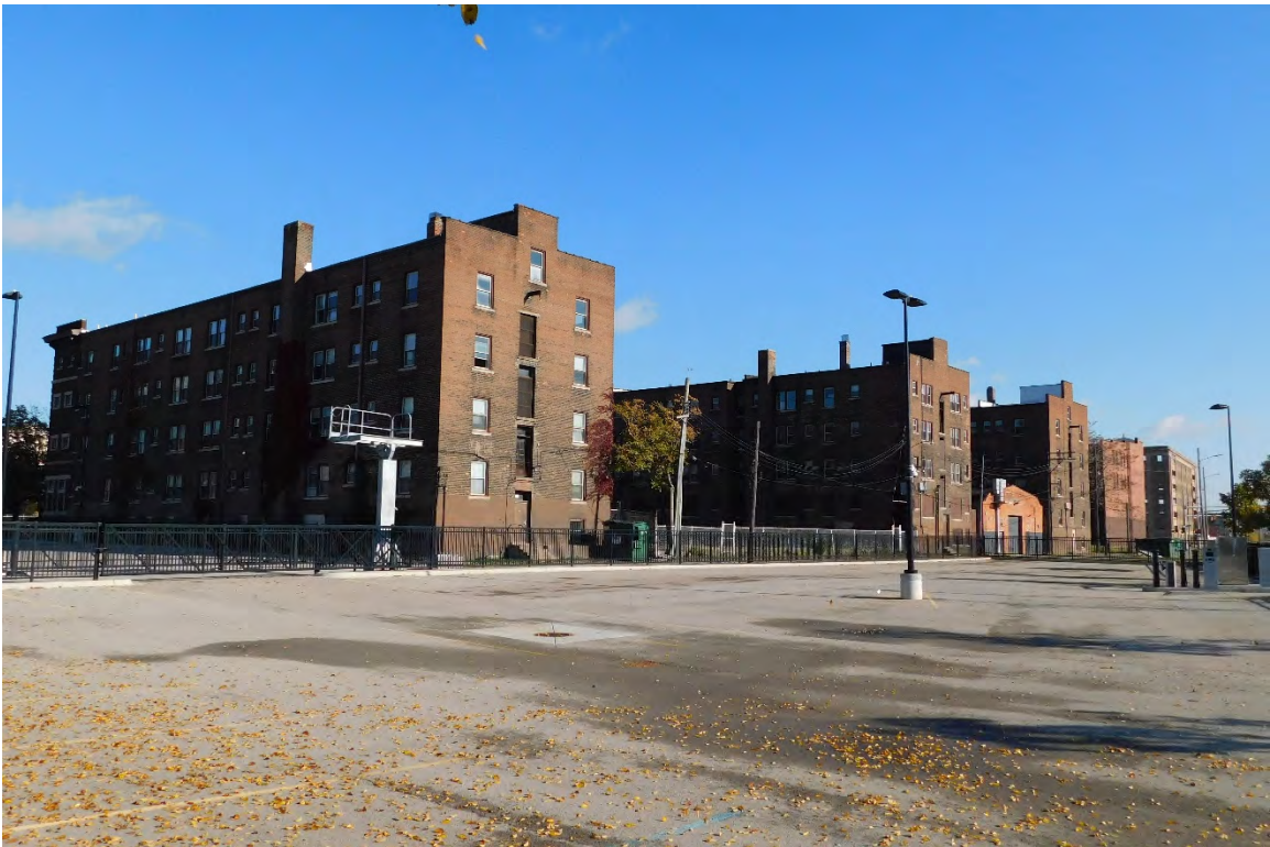
Figure #04: Exterior, View from W Fisher Service Drive, Looking Northeast. 10/28/20.
