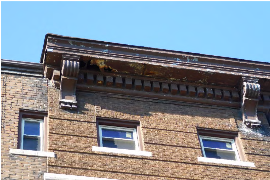
Figure #09: Exterior, East Façade Pressed Tin Cornice Detail, Looking Up. 10/28/20
