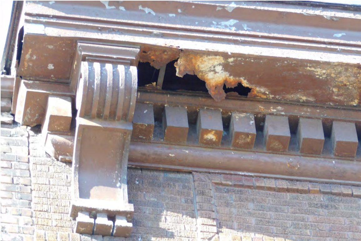
Figure #10: Exterior, East Façade Pressed Tin Cornice Detail, Looking Up. 10/28/20
