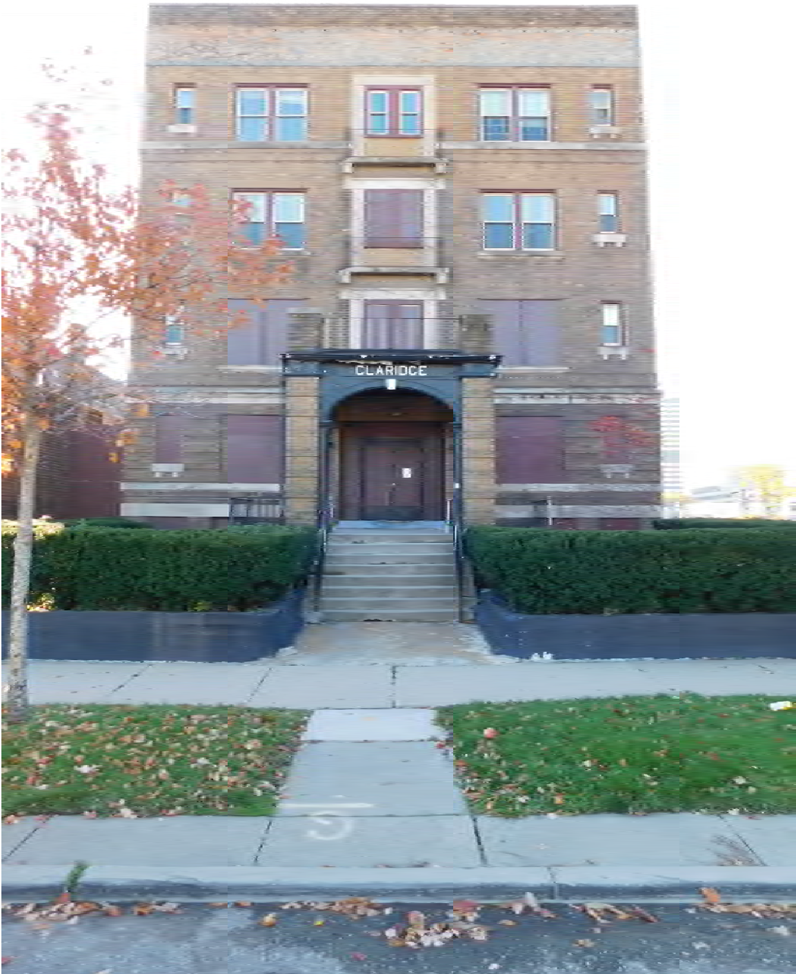
Figure #01: Exterior, North façade, Looking South. 10/28/20.
