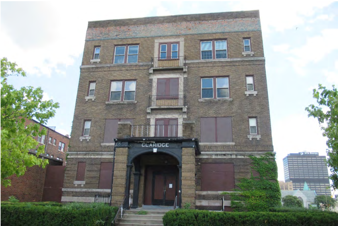
Figure #02: Exterior, North façade, Looking South. 10/28/20.
