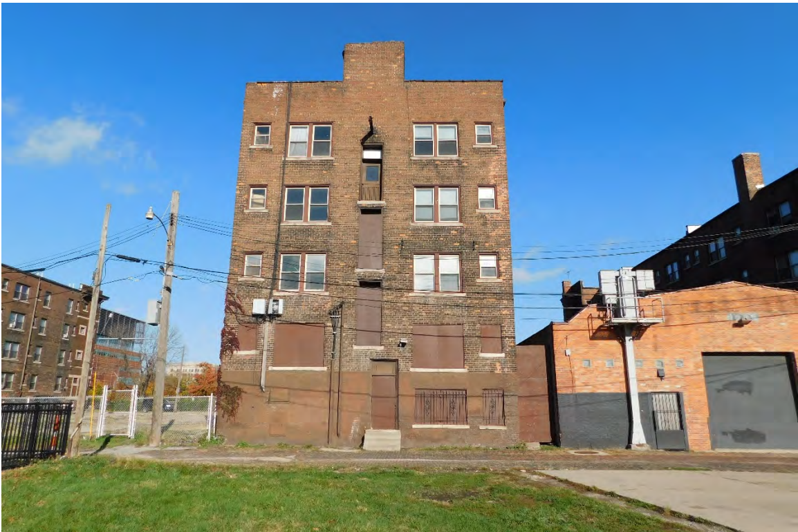
Figure #03: Exterior, South façades, Looking North. 10/28/20.
