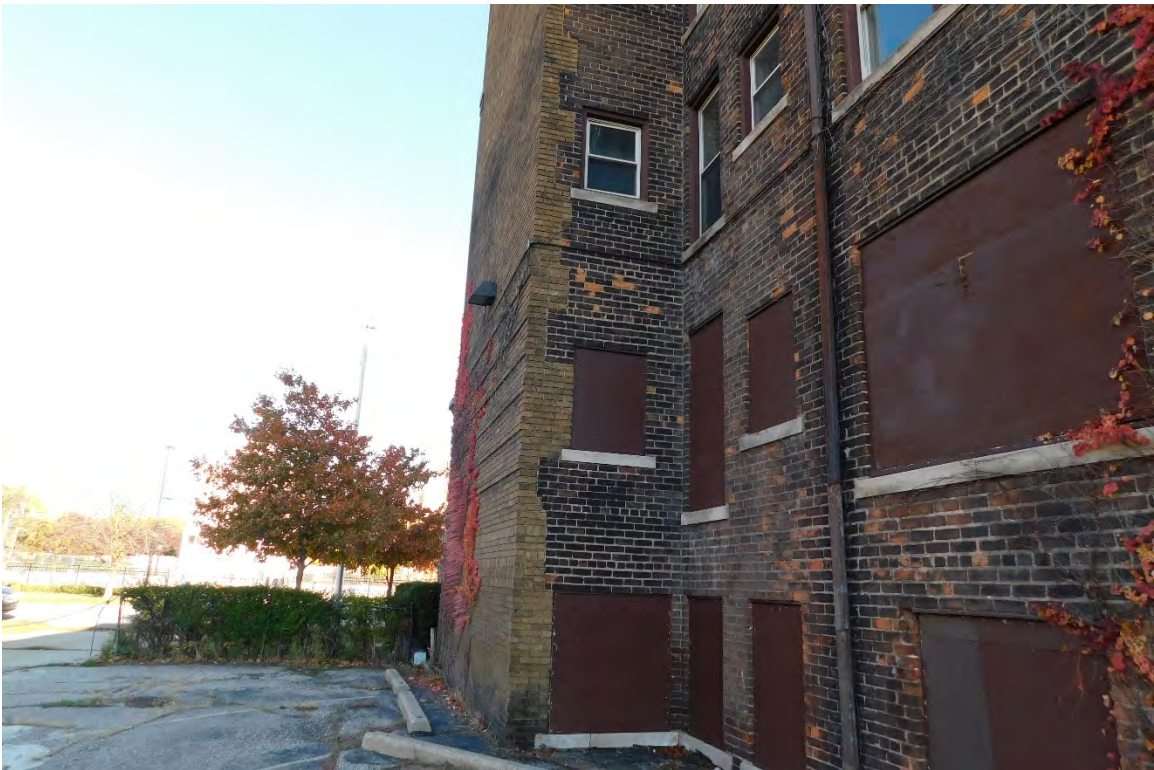
Figure #19: Exterior, West façade detail, Looking North. 10/28/20.
