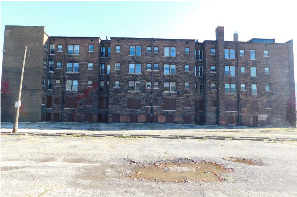
Figure #05: Exterior, West façade, Looking East. 10/28/20.
