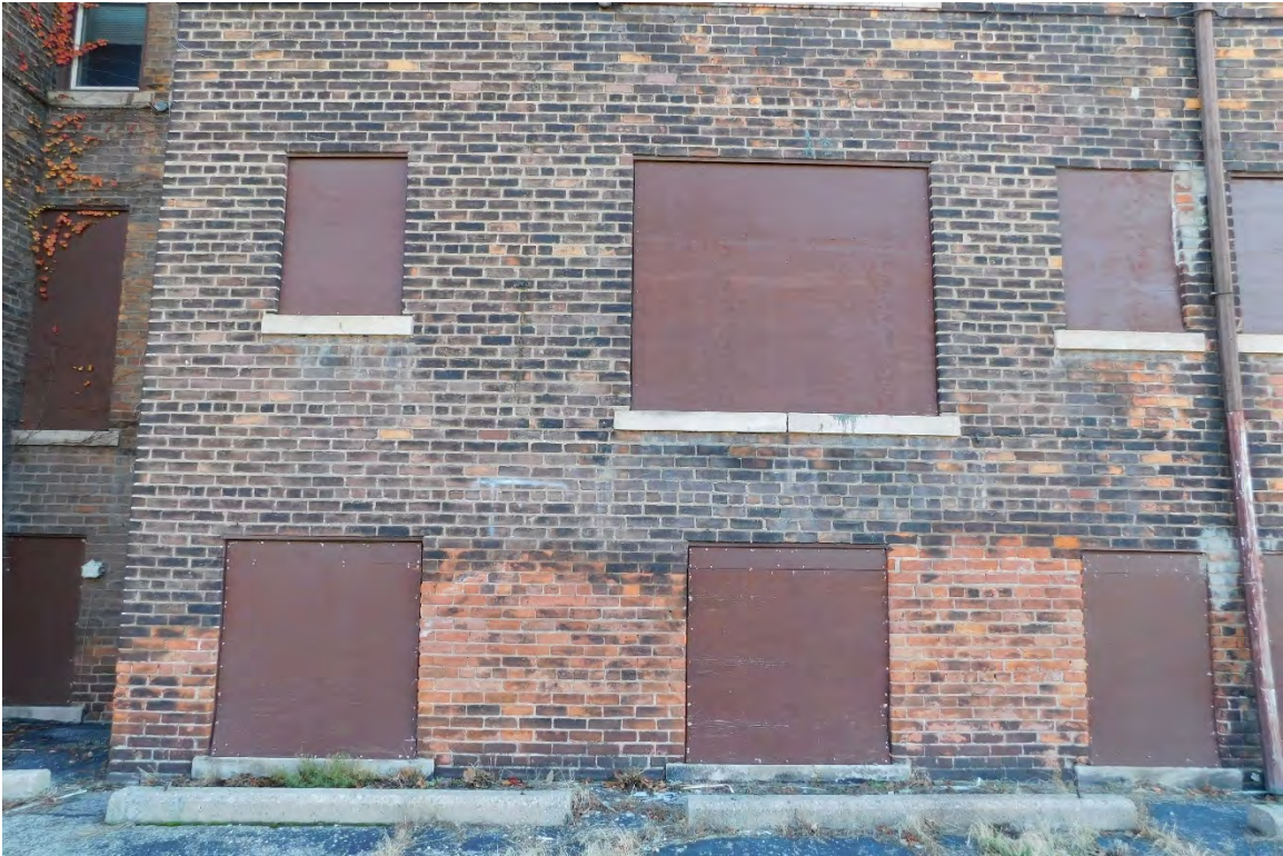
Figure #16: Exterior, West façade window detail, Looking East. 10/28/20.
