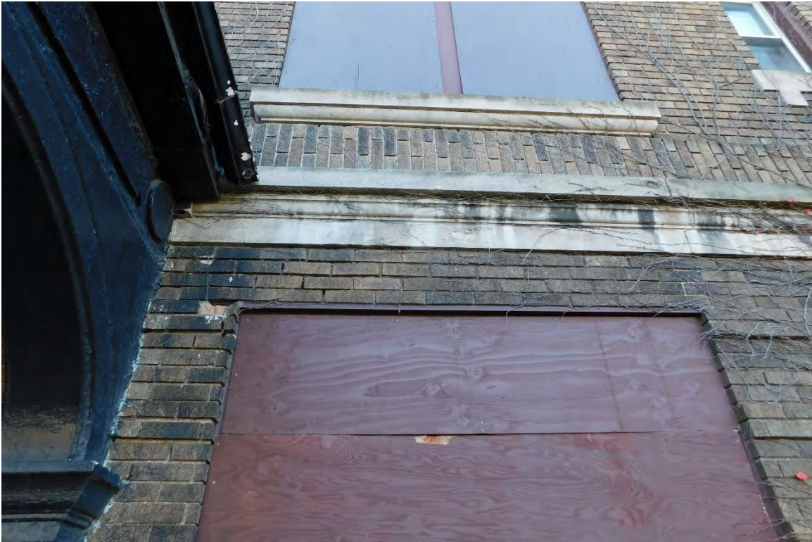
Figure #14: Exterior, North façade window and masonry detail, Looking Up. 10/28/20.
