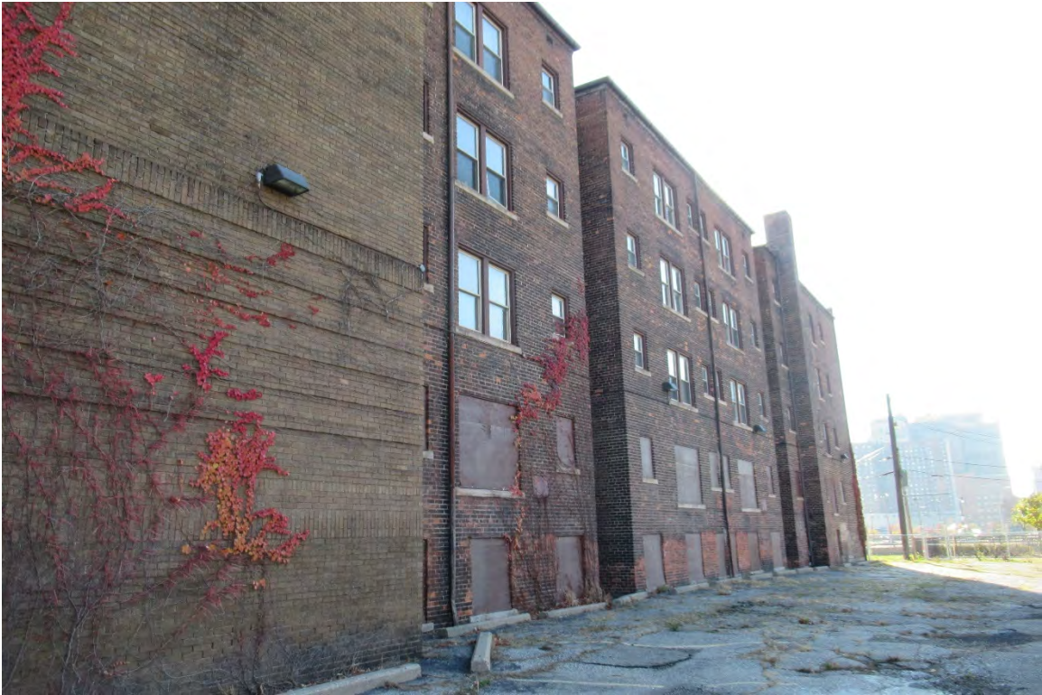
Figure #18: Exterior, West façade detail, Looking Southeast. 10/28/20.
