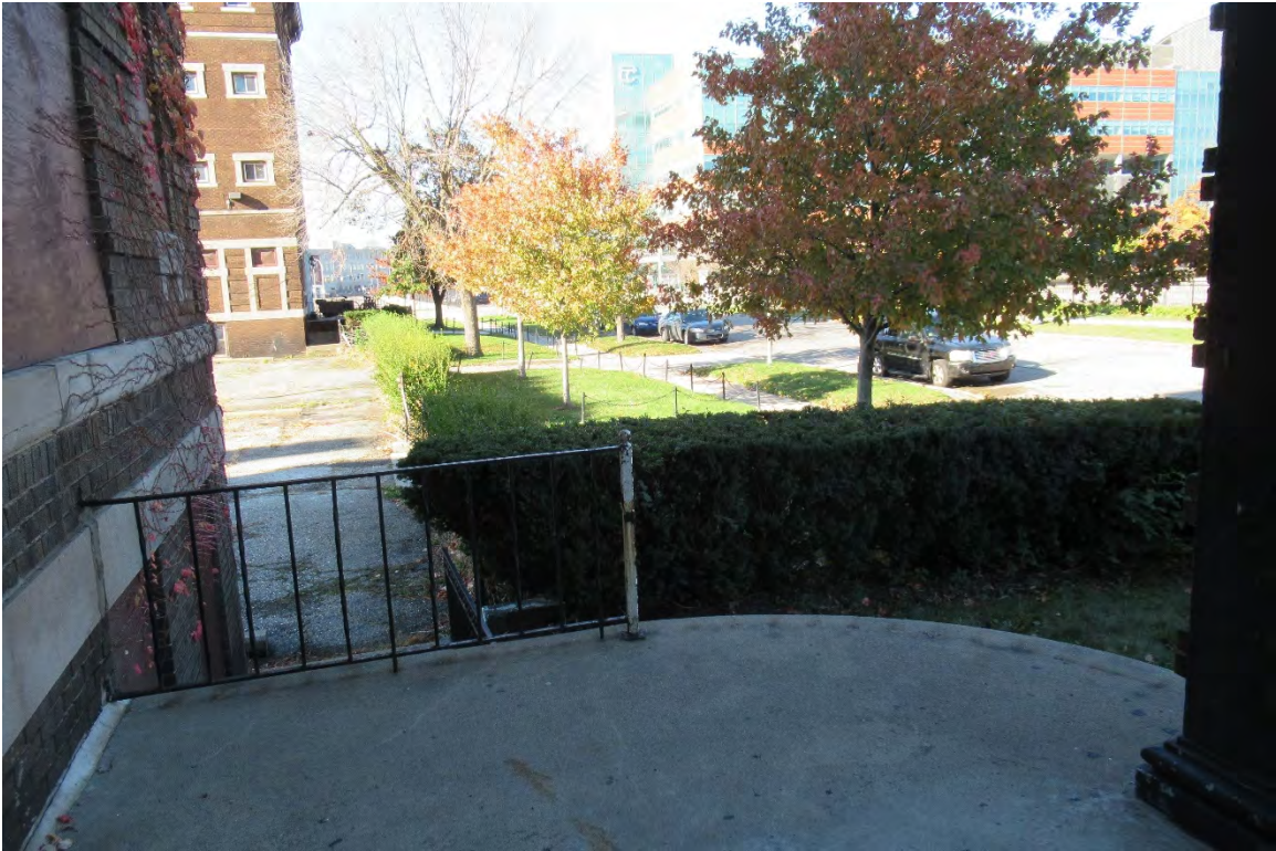
Figure #10: Exterior, North façade porch detail, Looking West. 10/28/20.
