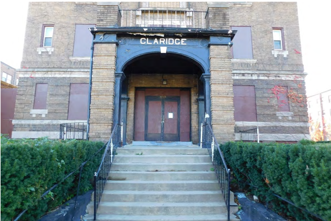
Figure #07: Exterior, North façade covered porch detail, Looking South. 10/28/20.
