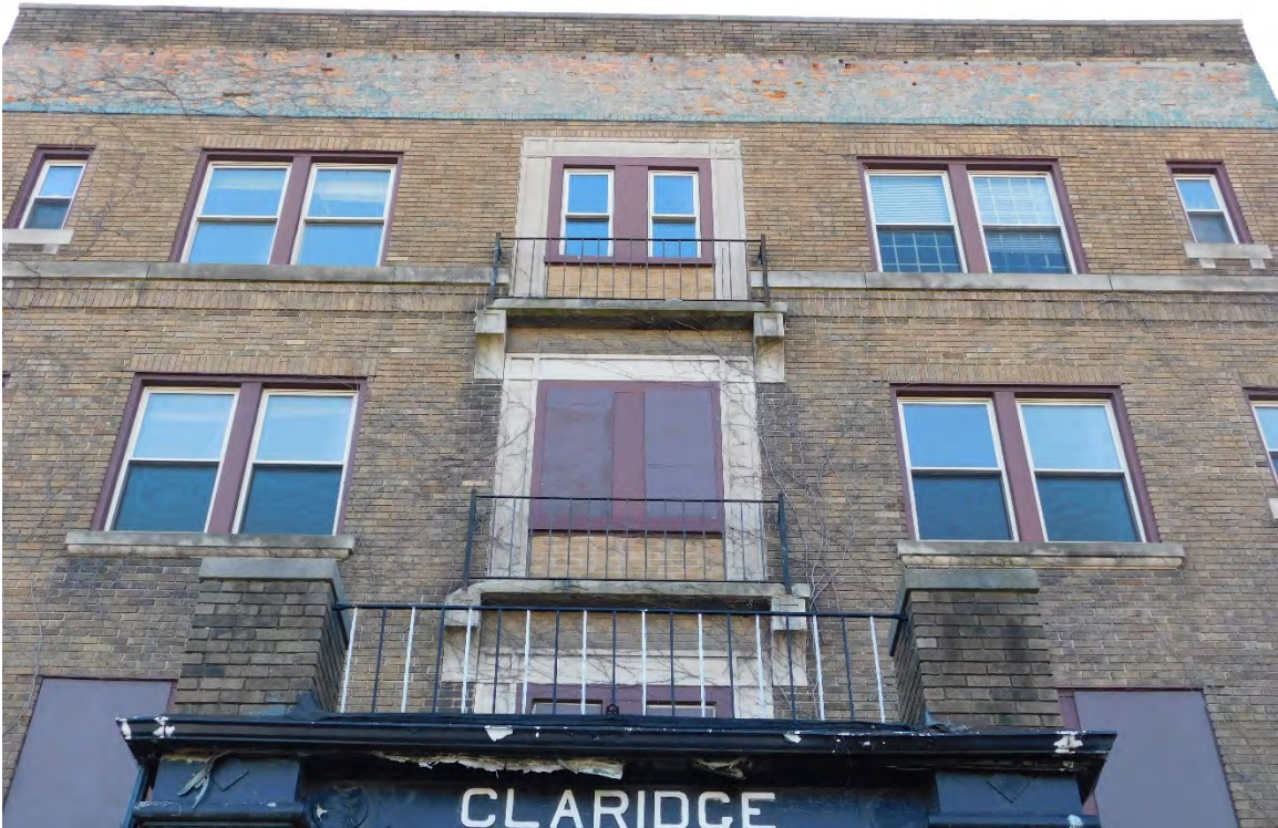
Figure #15: Exterior, North façade window and masonry detail, Looking Up. 10/28/20.
