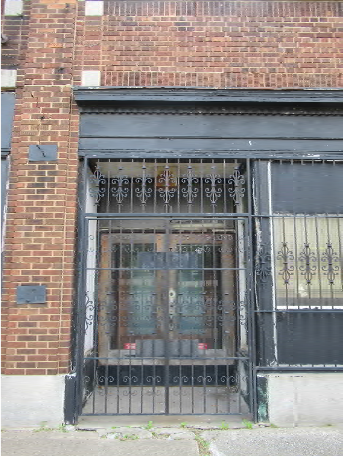
Figure #05: Exterior, North façade Storefront Entrance, Looking South. 07/28/20.
