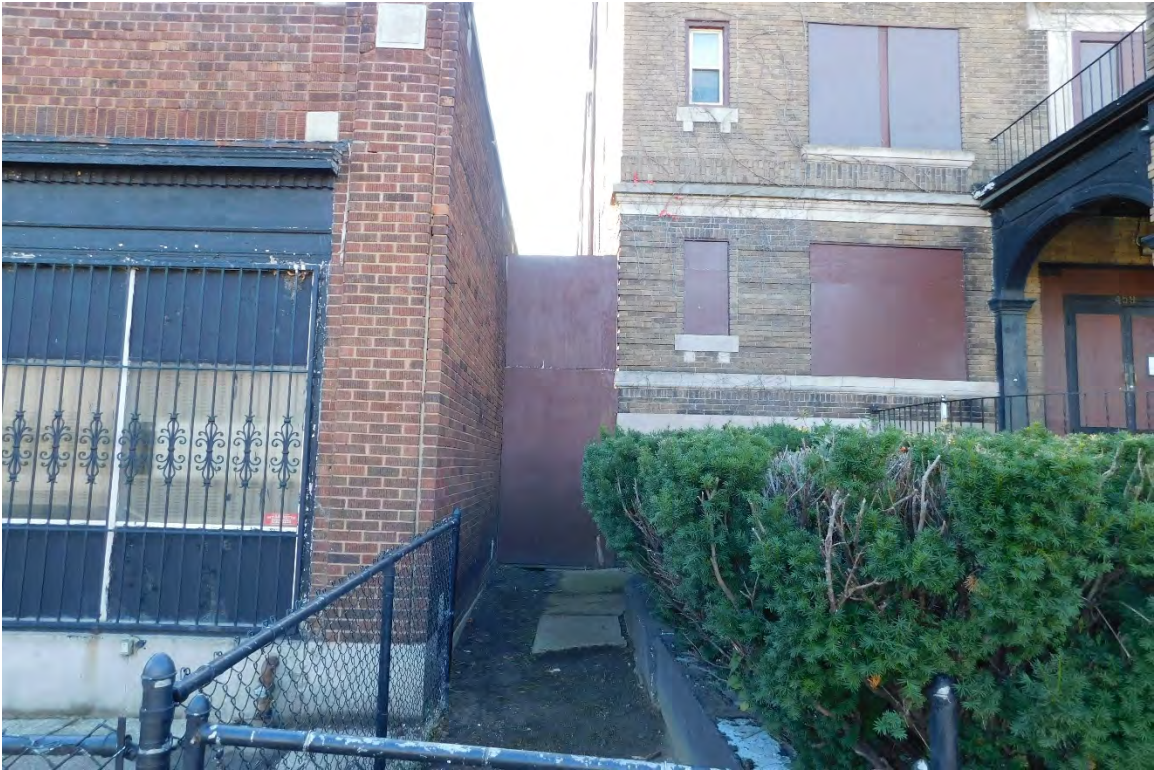
Figure #08: Exterior, Adjacency to 459 Henry (to right), Looking South. 10/28/20.
