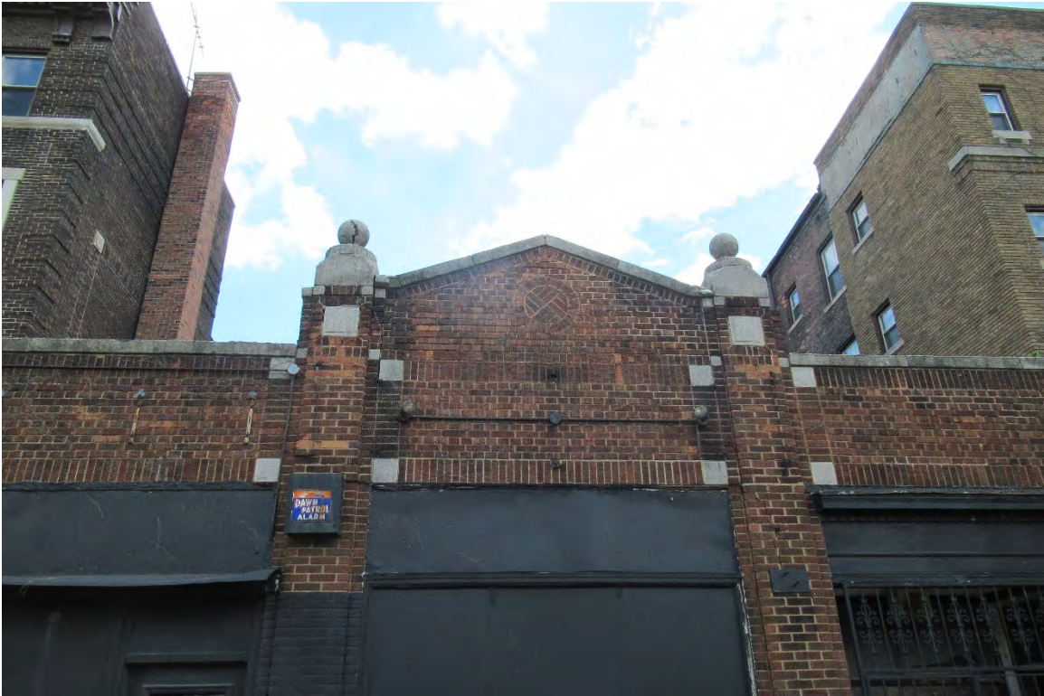
Figure #10: Exterior, North façade masonry and cast stone detail, Looking Up. 10/28/20.
