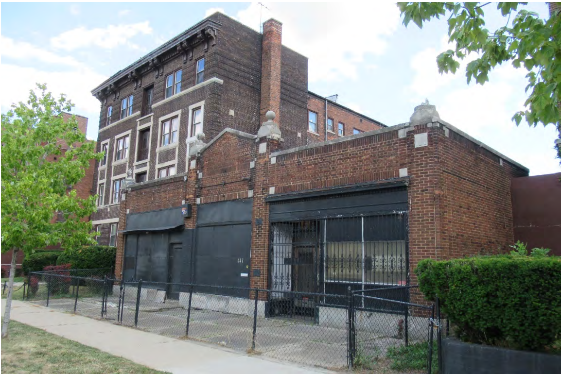
Figure #02: Exterior, West and North façades, Looking Southeast. 10/28/20.
