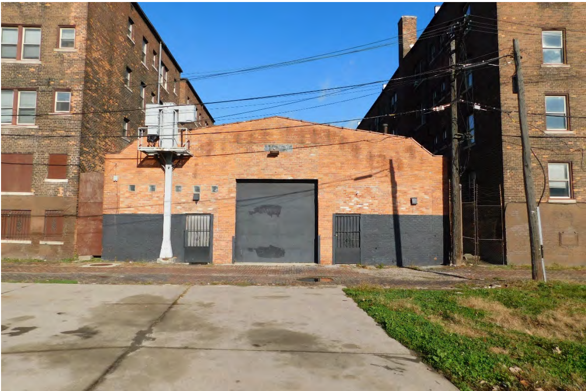
Figure #04: Exterior, South façade, Looking North. 10/28/20.
