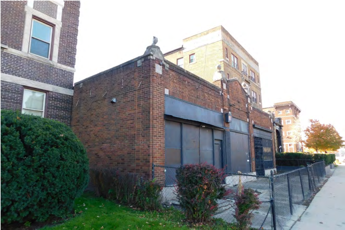
Figure #03: Exterior, East and North façade, Looking Southwest. 10/28/20.
