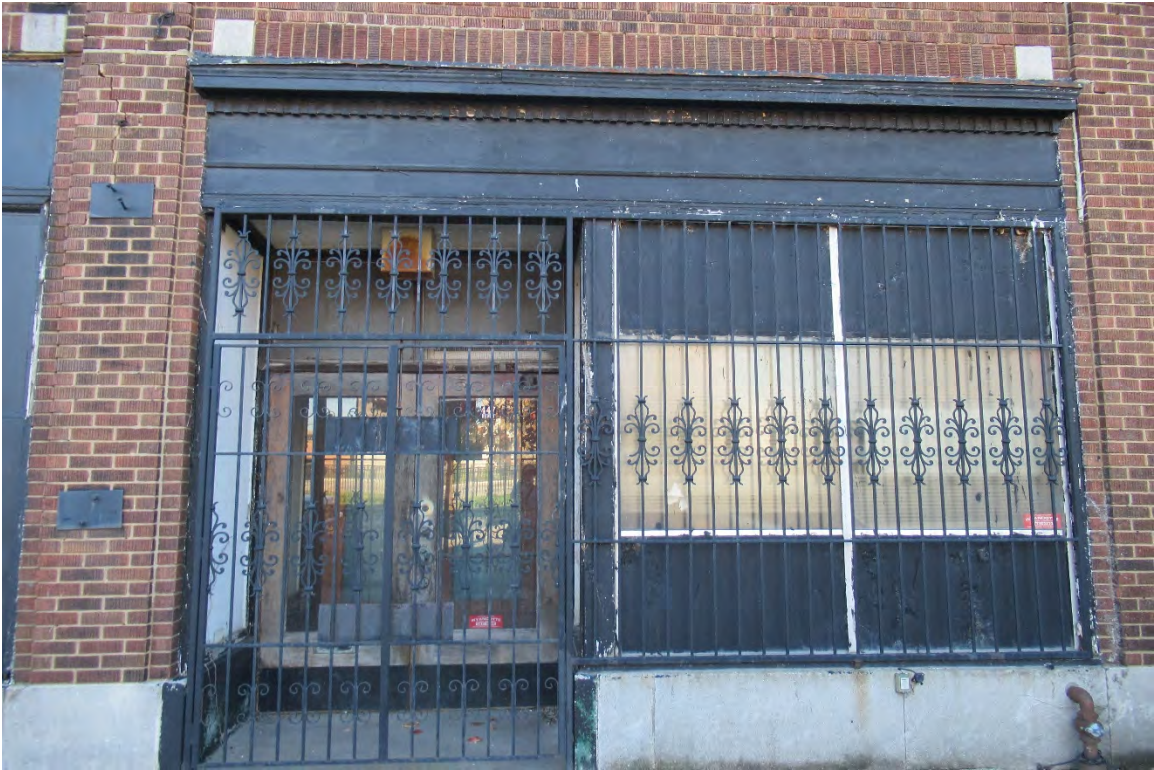
Figure #06: Exterior, North façade Storefront Entrance, Looking South. 10/28/20.
