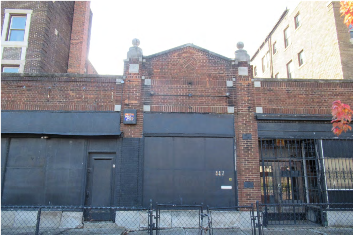
Figure #01: Exterior, North façade, Looking South. 10/28/20.
