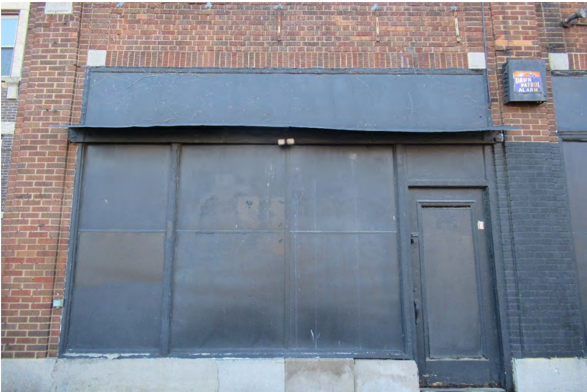
Figure #07: Exterior, North façade Storefront Entrance, Looking South. 10/28/20.
