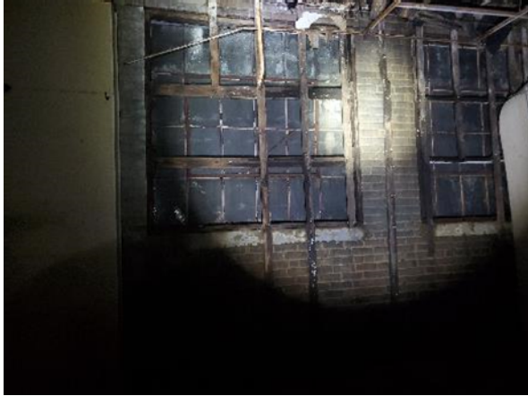
447 Henry- Steel Factory sash behind CMU infill- examine after CMU removed.
