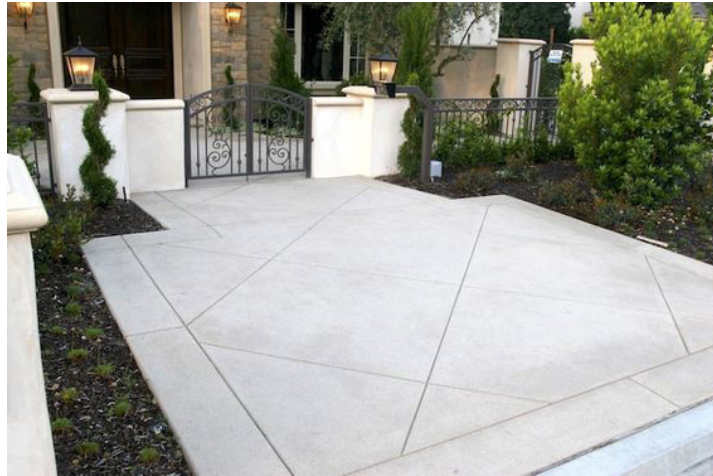
Concrete Pavement with Diamond Joint Pattern
