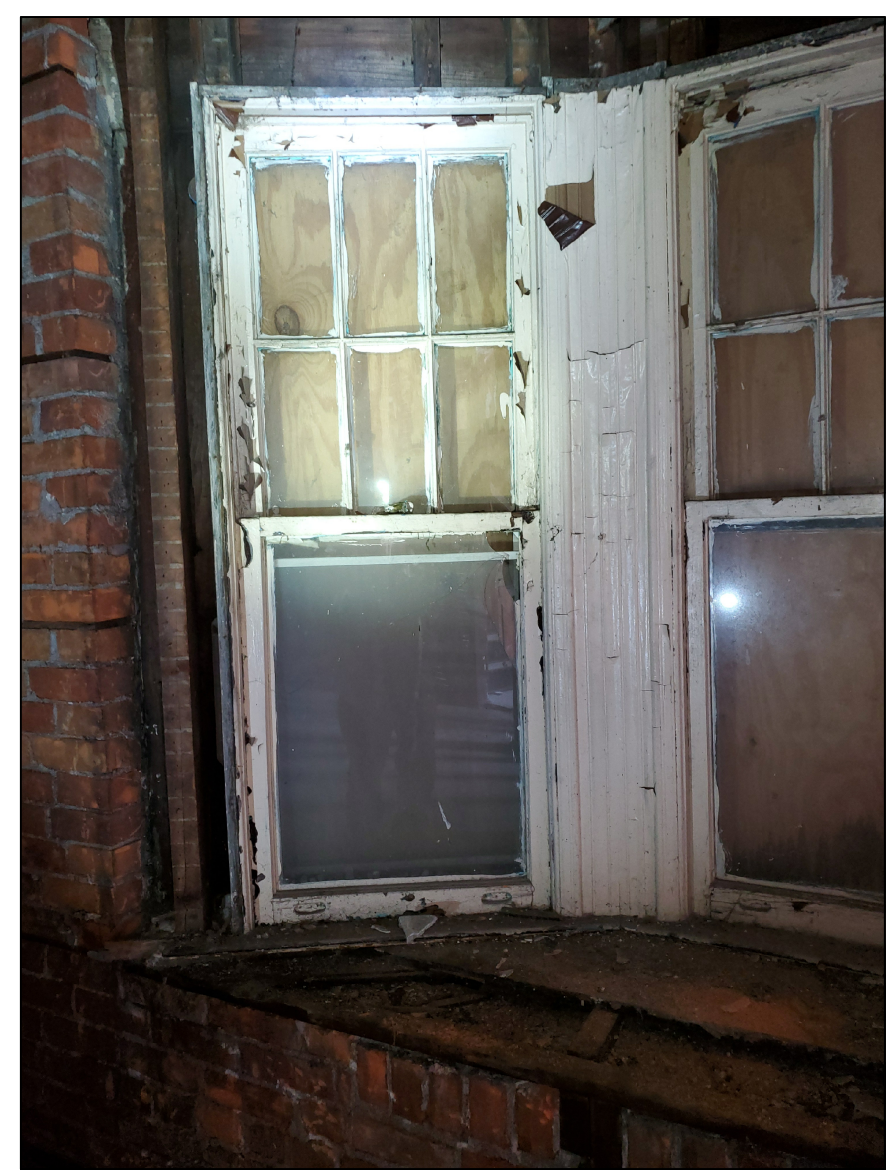
17 5A401 427 HENRY EXISTING PHOTO SCALE AS NOTED
