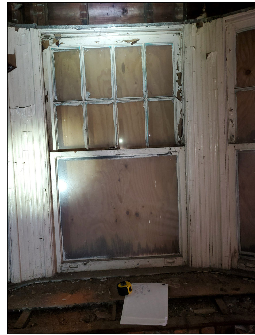
15 5A401 427 HENRY EXISTING PHOTO SCALE AS NOTED
