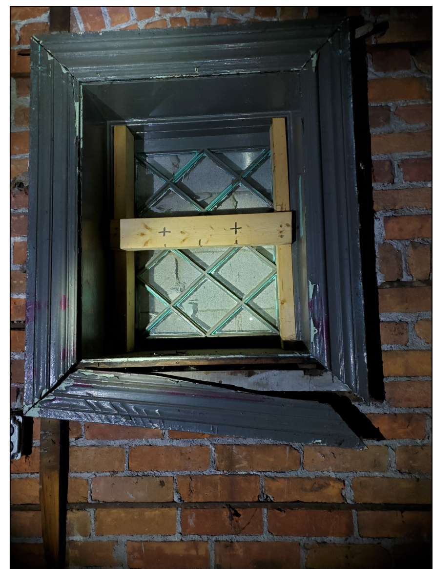
16 5A401 427 HENRY EXISTING PHOTO SCALE AS NOTED
