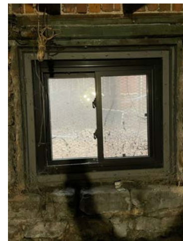
EXISTING BASEMENT VINYL WINDOW 7 (EAST)
