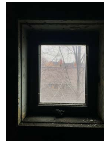
WINDOW 3D - EAST (INTERIOR) OUTSWING VINYL CASEMENT
