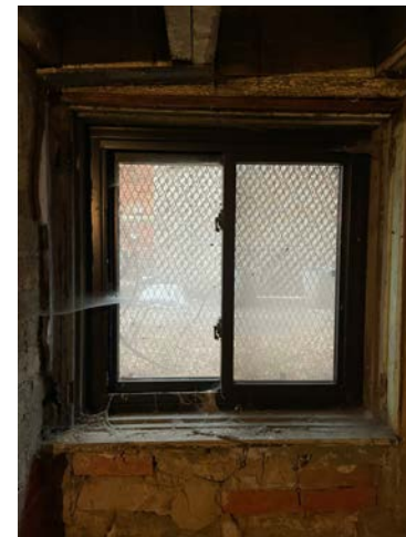
EXISTING BASEMENT VINYL WINDOW 3 (EAST)
