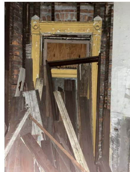
WINDOW 1E - WEST INTERIOR WOOD DOUBLE-HUNG
