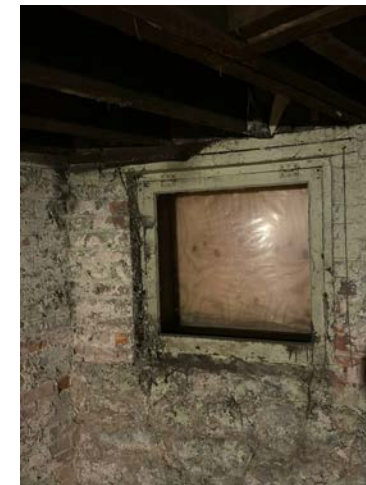
EXISTING BASEMENT WOOD WINDOW 3 (WEST)
