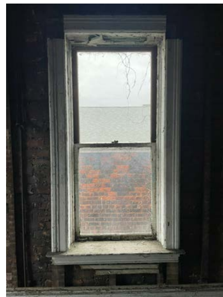
WINDOW 2G - WEST (INTERIOR) WOOD DOUBLE-HUNG
