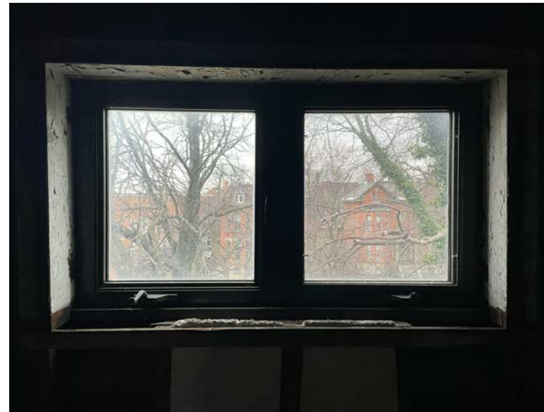
WINDOW 3B - EAST (INTERIOR) (2) OUTSWING VINYL CASEMENT
