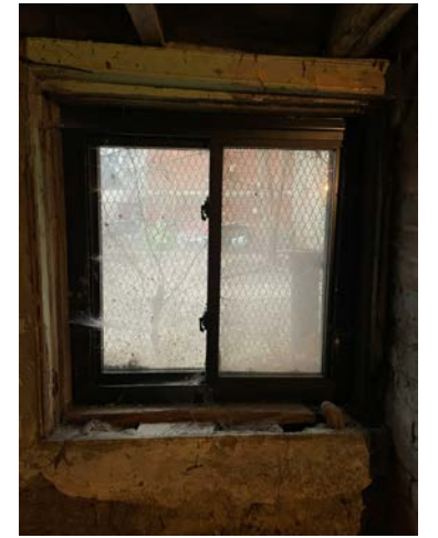
EXISTING BASEMENT VINYL WINDOW 2 (EAST)
