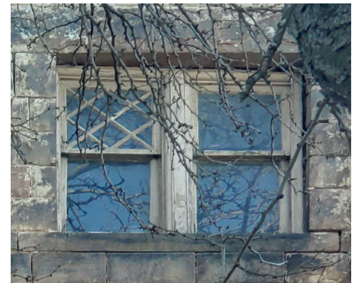
WINDOW 3A - WEST WOOD DOUBLE-HUNG
