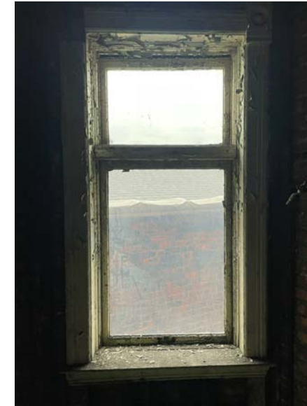
WINDOW 2D - WEST (INTERIOR) WOOD DOUBLE-HUNG
