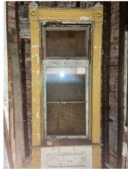
EXISTING WINDOW 1D - WEST WOOD DOUBLE-HUNG
