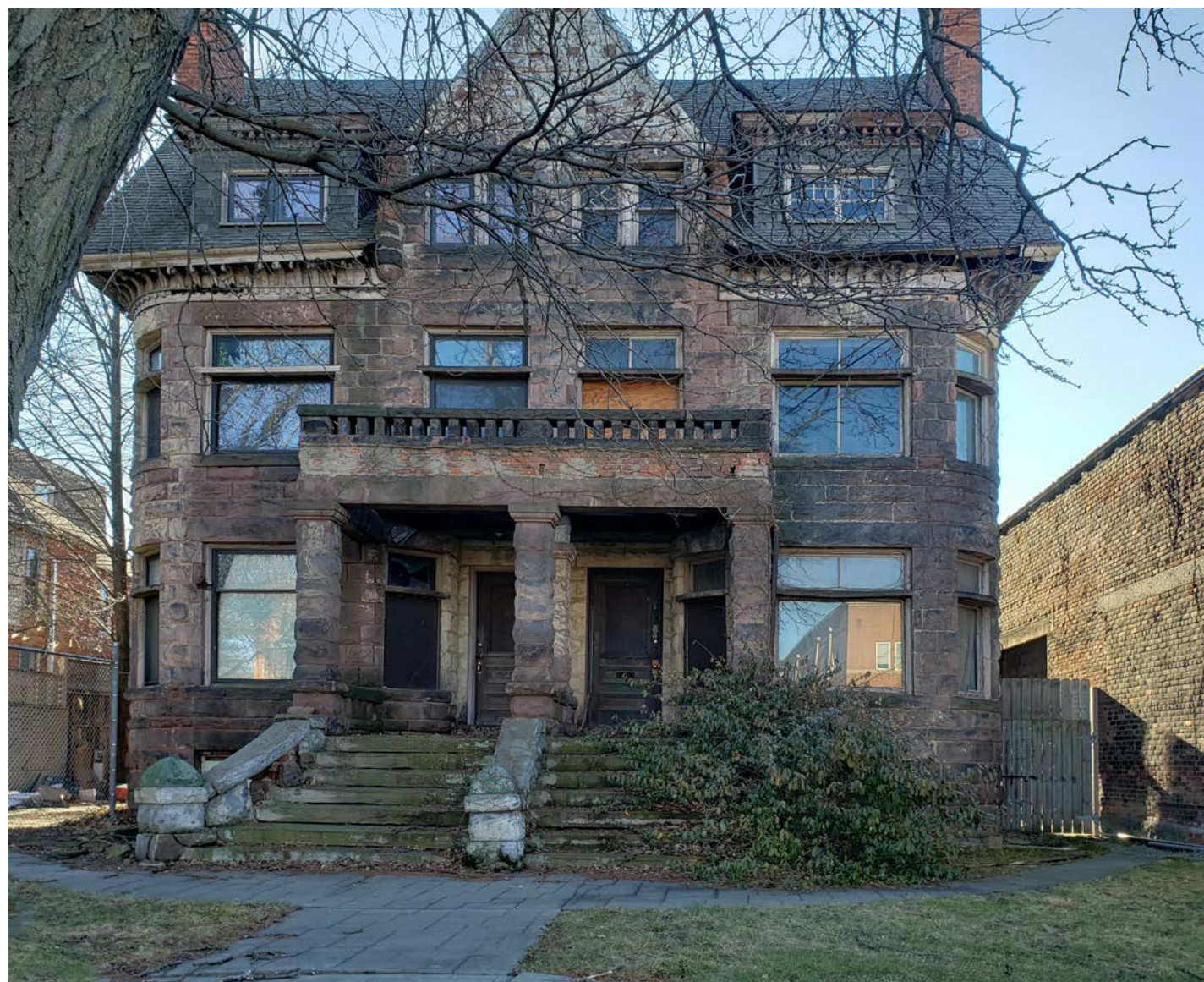
1. PHOTO FROM STREET - EXISTING CONDITIONS
