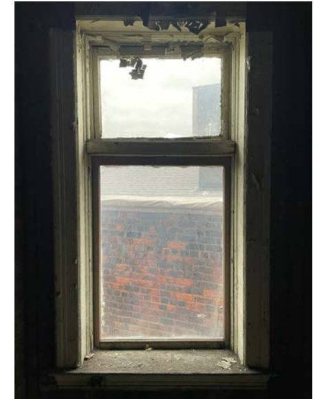
WINDOW 2E - WEST (INTERIOR) WOOD DOUBLE-HUNG
