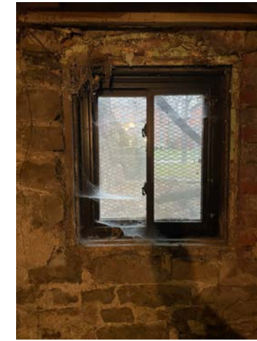
EXISTING BASEMENT VINYL WINDOW 1 (EAST)
