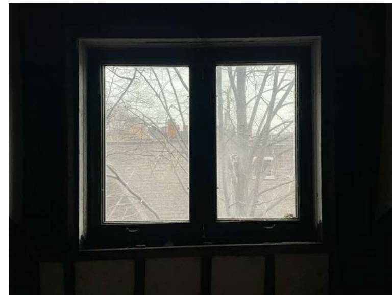
WINDOW 3E - EAST (INTERIOR) (2) OUTSWING VINYL CASEMENT
