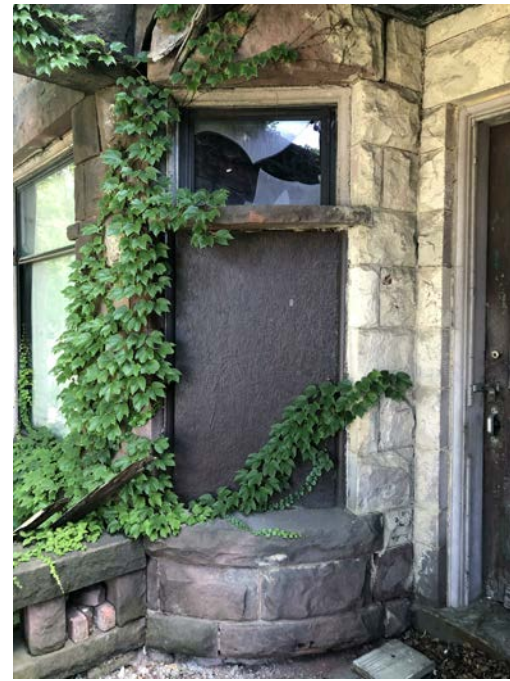
1A EAST - EXISTING EXTERIOR VINYL DOUBLE-HUNG
