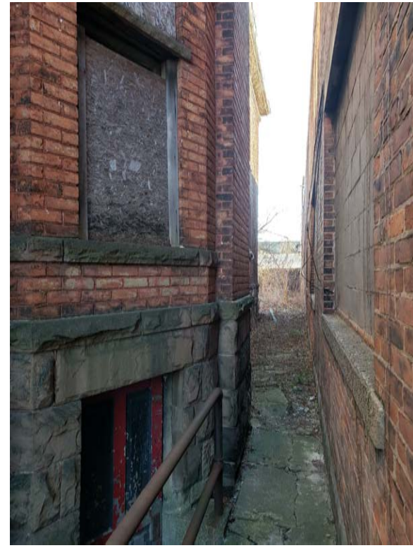
6. WEST ELEV. (TOWARD SOUTH)
