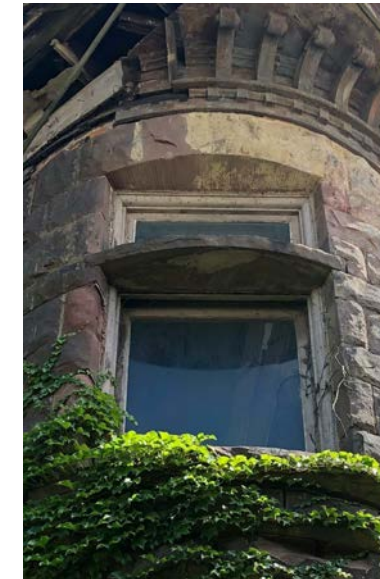
WINDOW 2C - WEST WOOD DOUBLE-HUNG
