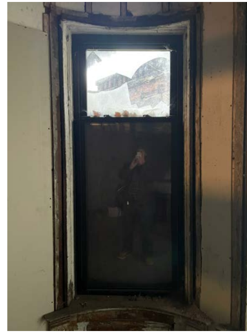
1A EAST - EXISTING INTERIOR VINYL DOUBLE-HUNG
