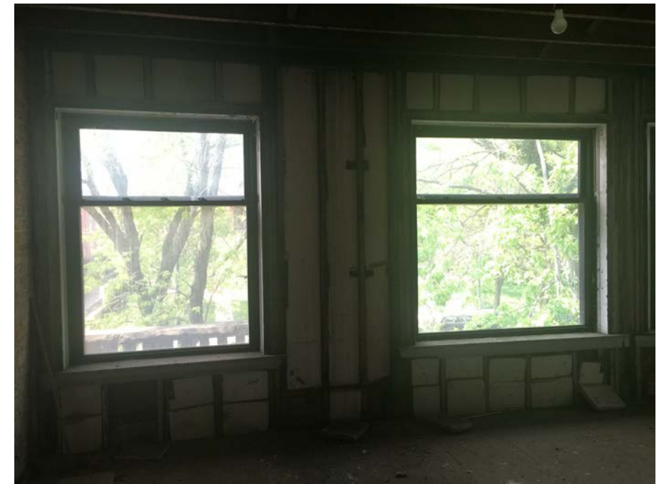
3. EXISTING WINDOW TYPES 2A & 2B (EAST)
