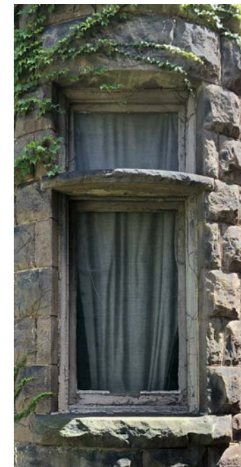
1C WEST - EXTERIOR WOOD DOUBLE-HUNG
