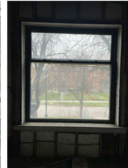
WINDOW 2B - EAST (INTERIOR) VINYL DOUBLE-HUNG
