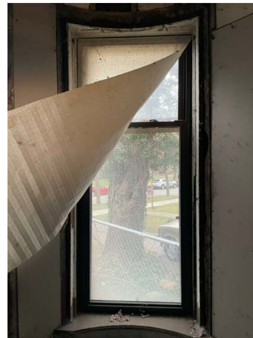
1C EAST - EXISTING INTERIOR WOOD DOUBLE-HUNG
