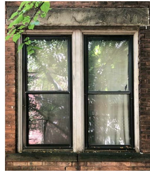
EXISTING WINDOW 1F - EAST VINYL DOUBLE-HUNG
