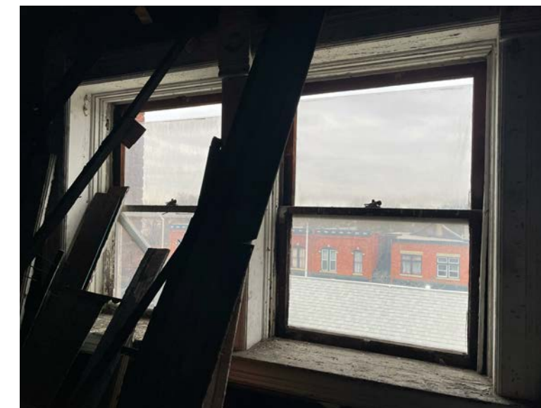
WINDOW 3C - WEST (2) WOOD DOUBLE-HUNG
