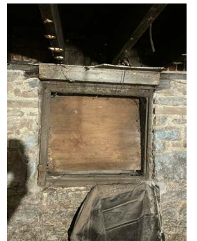
EXISTING BASEMENT WOOD WINDOW 4 (WEST)
