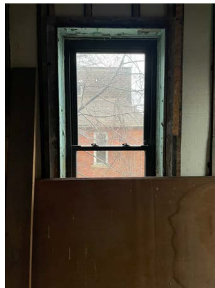
WINDOW 2G - EAST (INTERIOR) VINYL DOUBLE-HUNG
