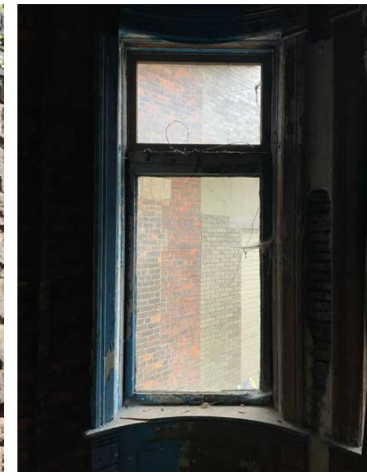
1C WEST - EXISTING INTERIOR WOOD DOUBLE-HUNG
