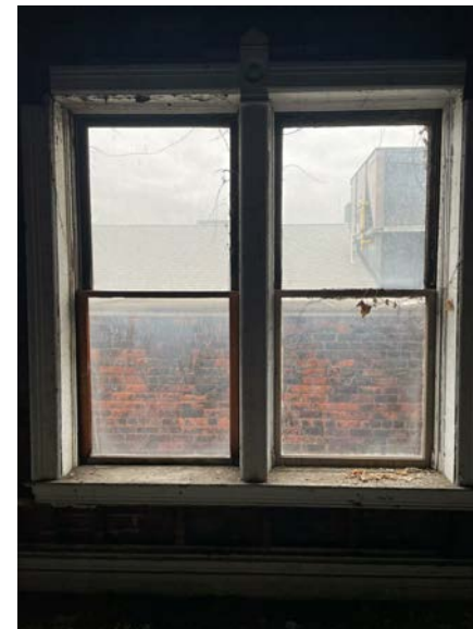
WINDOW 2F - WEST (INTERIOR) WOOD DOUBLE-HUNG
