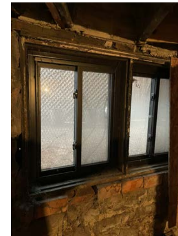
EXISTING BASEMENT VINYL WINDOWS 4 & 5 (EAST)
