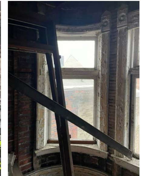
WINDOW 2C - WEST (INTERIOR) WOOD DOUBLE-HUNG
