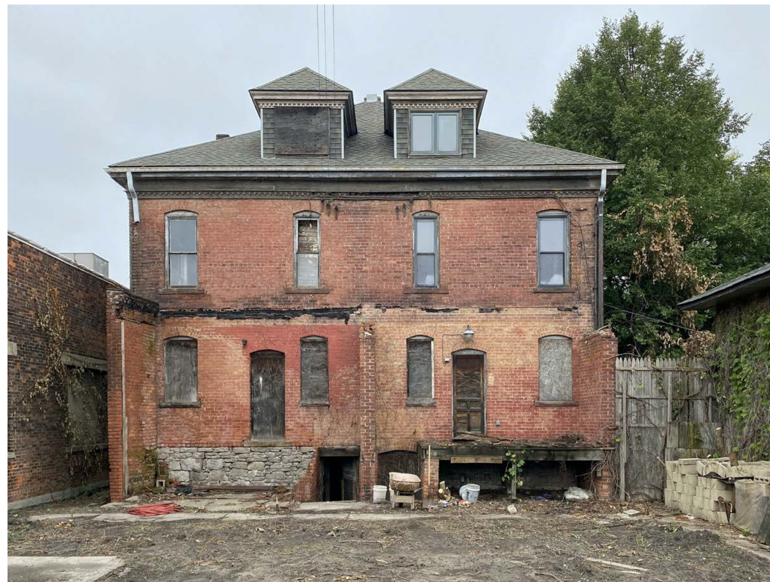
2. PHOTO FROM REAR - EXISTING CONDITIONS
