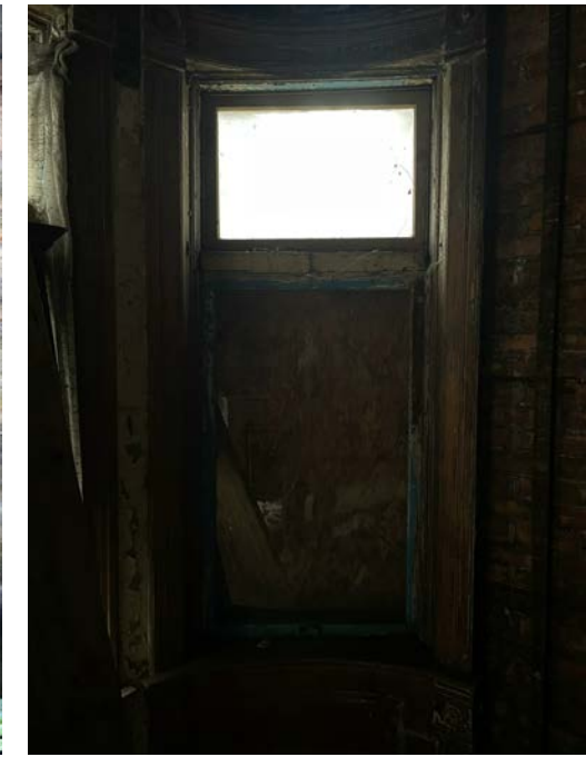
1A WEST - EXISTING INTERIOR WOOD DOUBLE-HUNG
