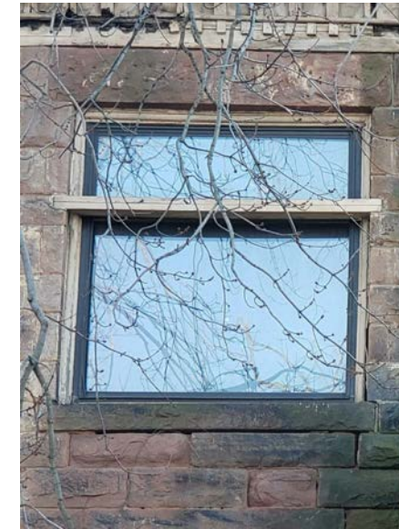
WINDOW 2B - EAST VINYL DOUBLE-HUNG
