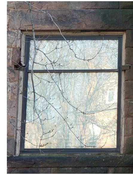
EXISTING WINDOW 1B - EAST VINYL DOUBLE-HUNG
