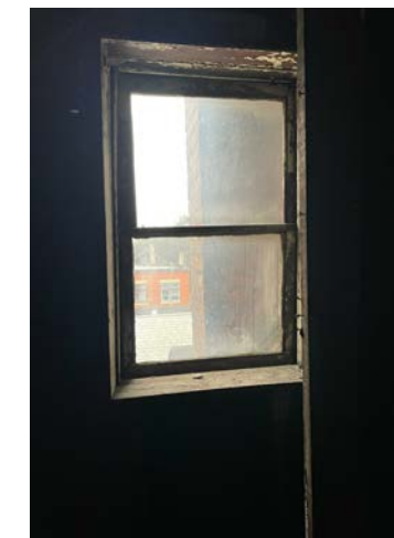
WINDOW 3D - WEST (INTERIOR) WOOD DOUBLE-HUNG
