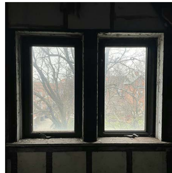
WINDOW 3A - EAST (INTERIOR) VINYL CASEMENT
