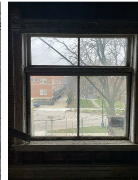
WINDOW 2B - WEST (INTERIOR) WOOD DOUBLE-HUNG
