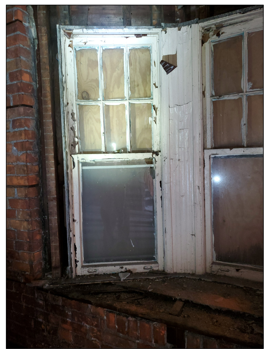
17 5A401 427 HENRY EXISTING PHOTO SCALE AS NOTED
