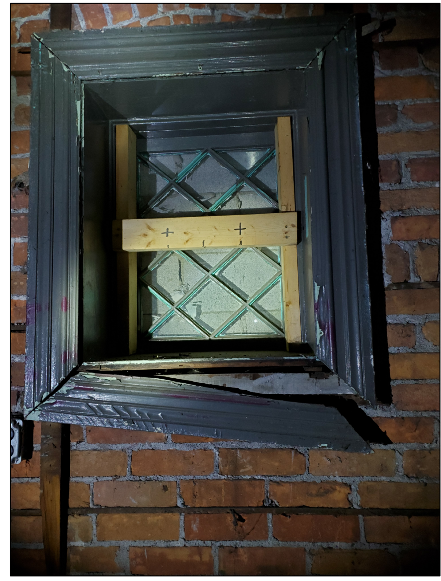
16 5A401 427 HENRY EXISTING PHOTO SCALE AS NOTED
