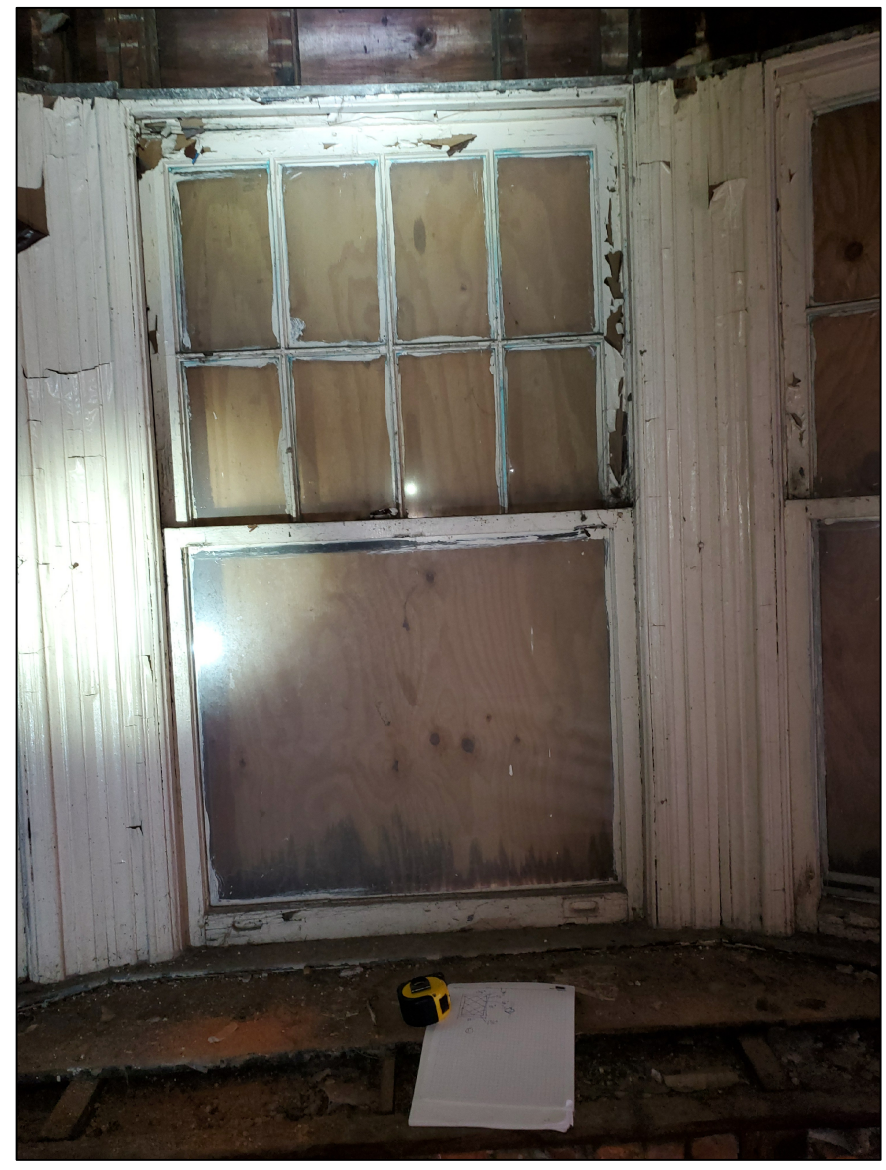
15 5A401 427 HENRY EXISTING PHOTO SCALE AS NOTED
