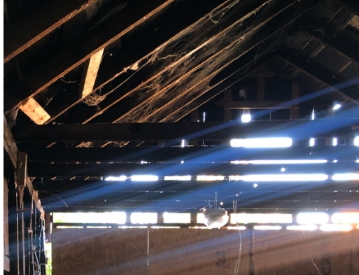
P1: Roof Framing Members
