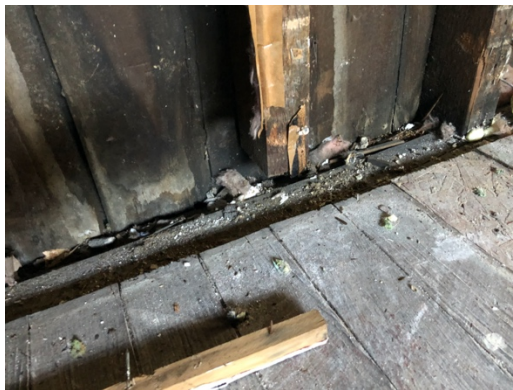
P6: Wall Framing Conditions
