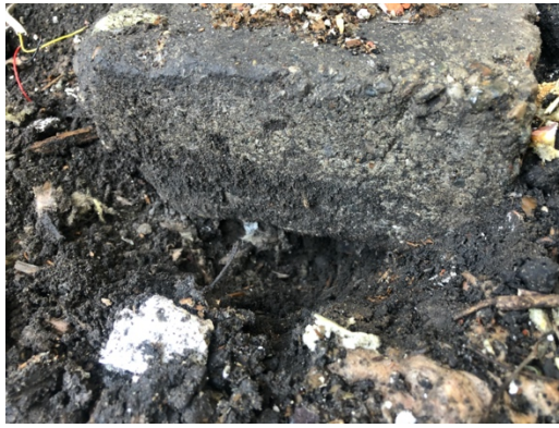
P8: Foundation Above Frost Depth
