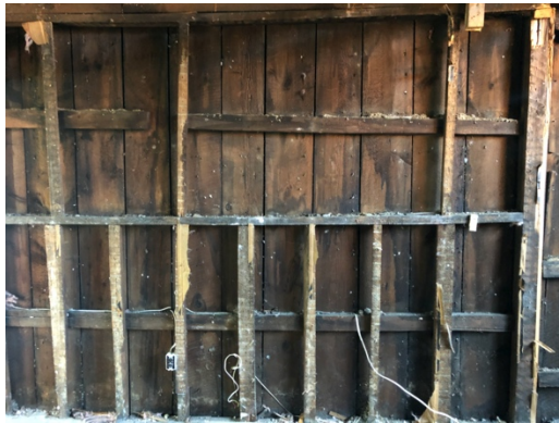
P5: Wall Framing Conditions
