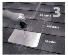
Locate, choose, and mark centers of rafters to be Carefully lift composition roof shingle with roofing Insert flashing between 1st and 2nd course. Slide up so top edge of flashing is at least 44\* higher than the butt-edge of the 3rd course and lower sealant. See "Proper Flashing Placement" on next flashing edge is above the butt-edge of 1st course. Mark center for drilling.
