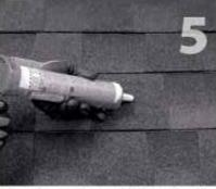
If attaching with lag bolt use a 3/22\* bit (Lag). Use a Clean off any sawdust, and fill hole with sealant
