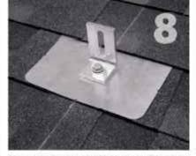
Follow all the directions of the rack manufacturer as well as the module manufacturer. NOTE: Make sure top of L-Foot makes solid contact with racking.
