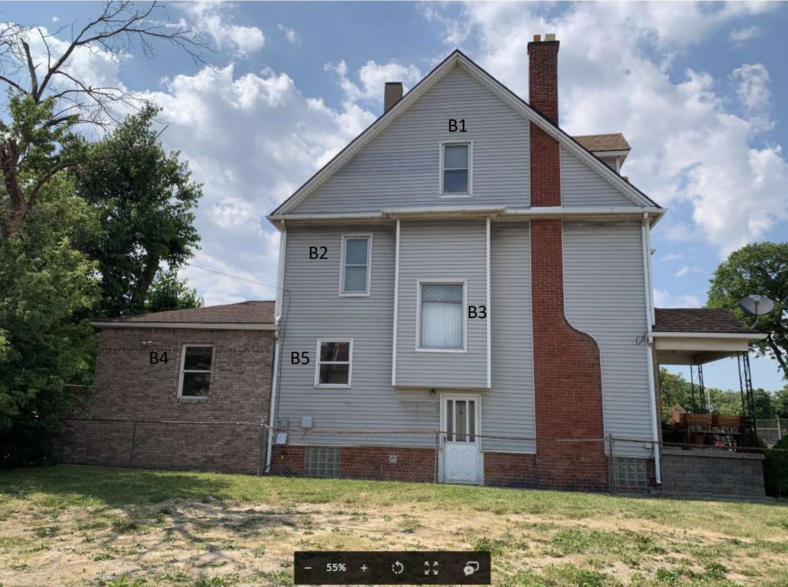
B4 and B5 are wood windows with vinyl cladding outside.
