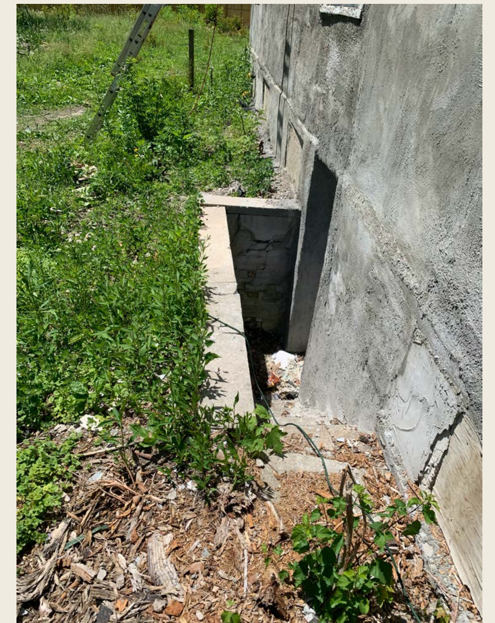
Existing side yard door the new driveway would need got be 3 feet away
