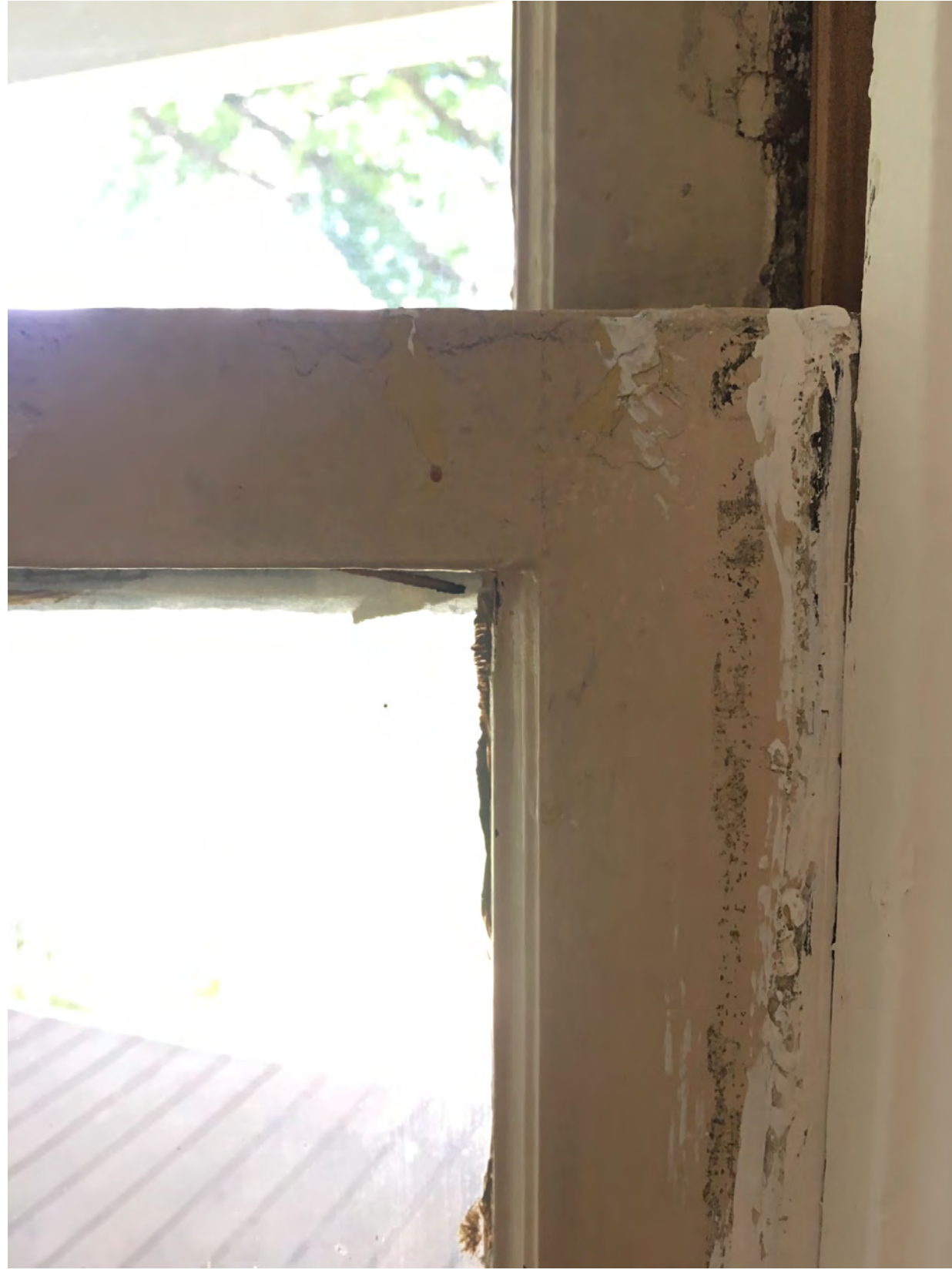
Current Interior Corner Profile, View 2
