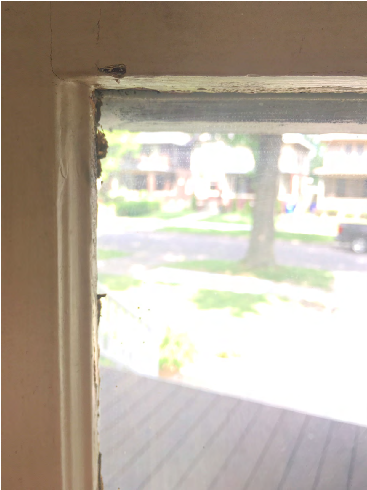
Current Interior Corner Profile, View 1
