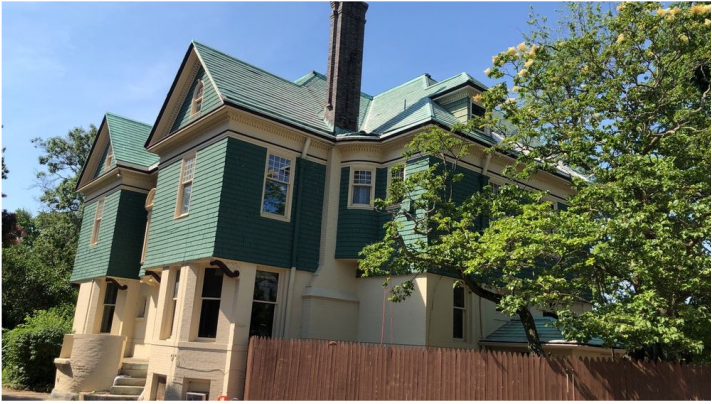
Project: Fay, Evan Date: June 20th, 2020, 10:56 a.m. Creator: Mason Mahaffey
