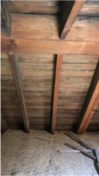
Project: Fay, Evan Date: June 20th, 2020, 11:17 a.m. Creator: Mason Mahaffey
