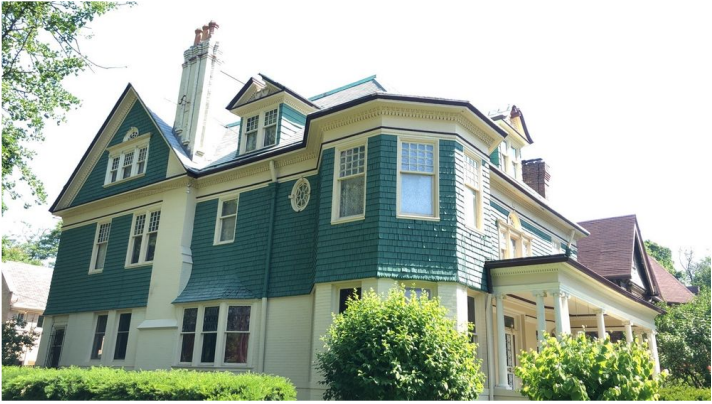
Project: Fay, Evan Date: June 20th, 2020, 11:05 a.m. Creator: Mason Mahaffey
