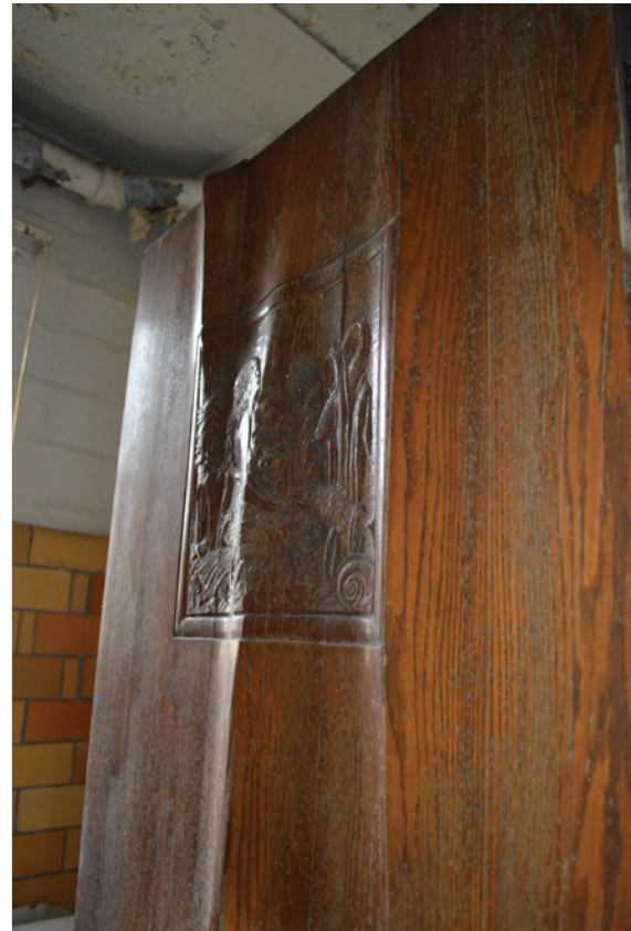
Carved veneer by Tabaczuk, warped and delaminated
