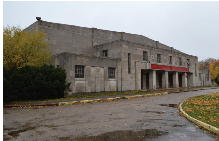
Iconic Jefferson Avenue north facade
