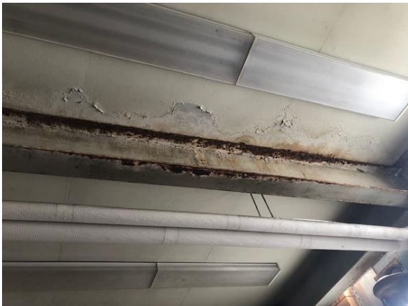
P-6: Mechanical Penetrations
