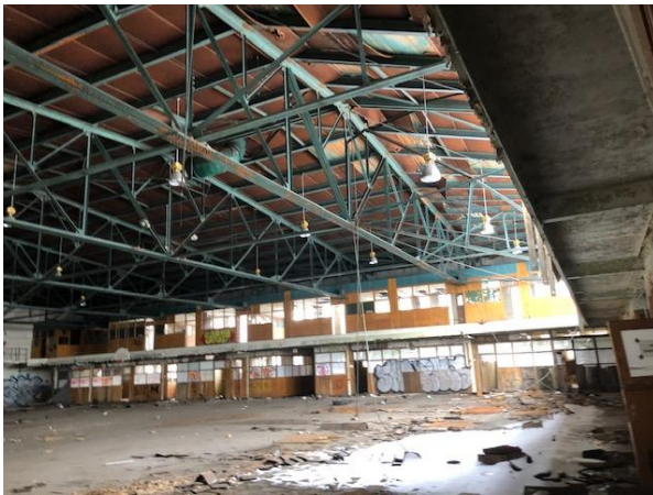
P-1 First-floor structural slab
