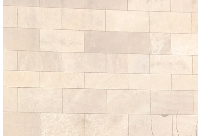
LIMESTONE PANELS FROM SOUTH BUILDING
