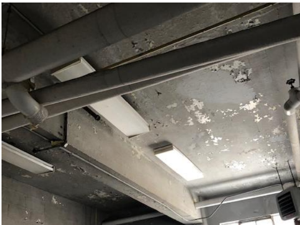
P-5 Mezzanine structural slab from below
