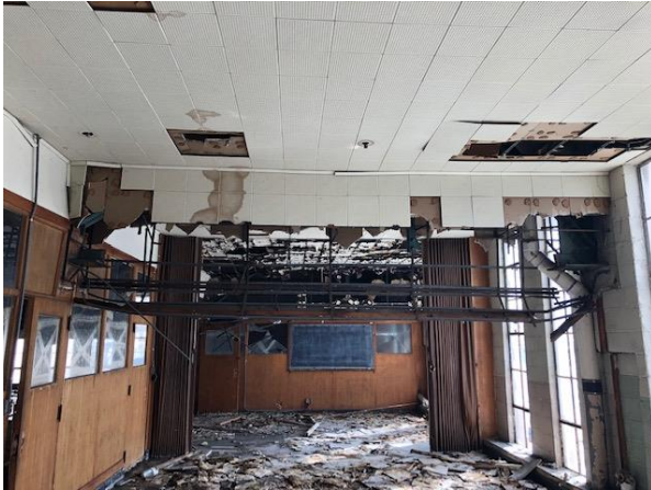
P-10 Removed truss bottom chord (2 nd truss)
