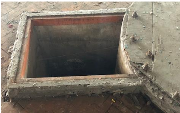
P-3: Mechanical penetrations
