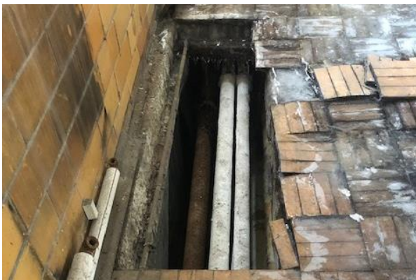
P-2 Mechanical penetrations
