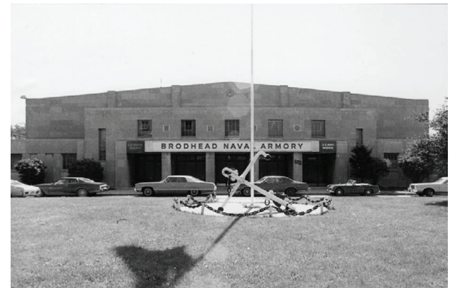
Front facade and lawn, c. 1970s. Source: G. Garner
