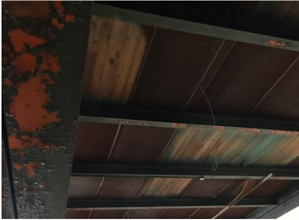
P-13 Roof purlins
