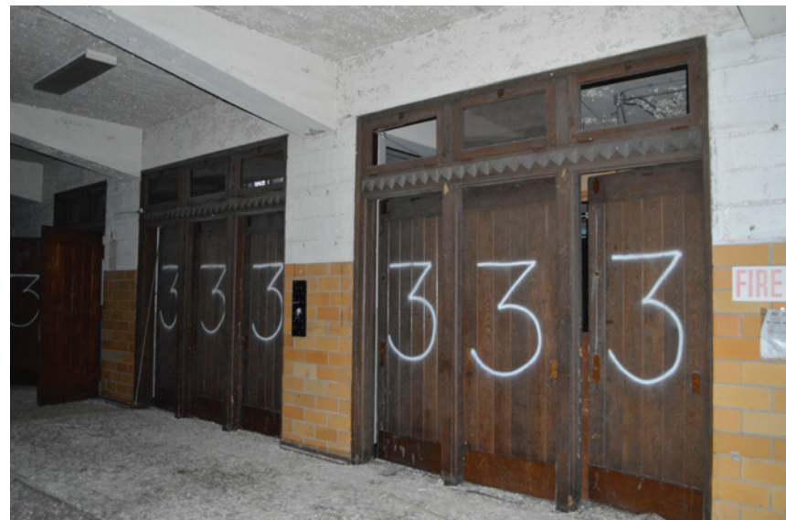
Entry vestibule interior doors
