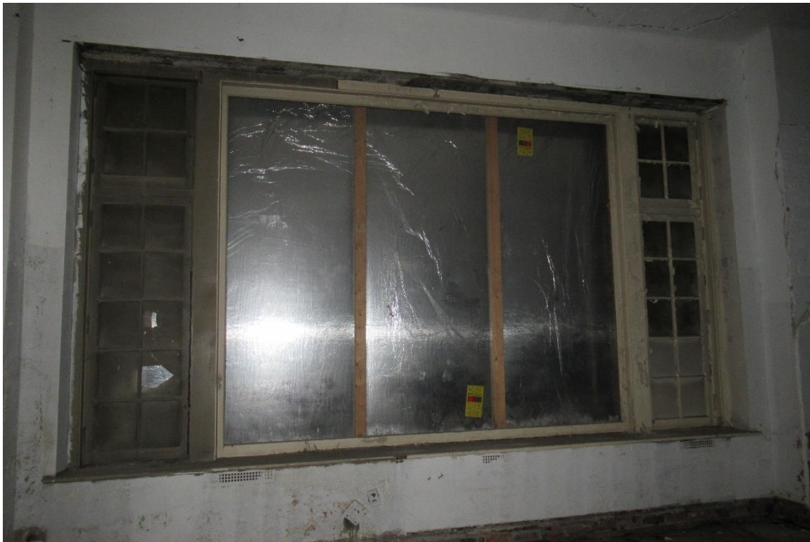
Figure #55: Interior, 2 nd floor, Looking East. 7/17/19
