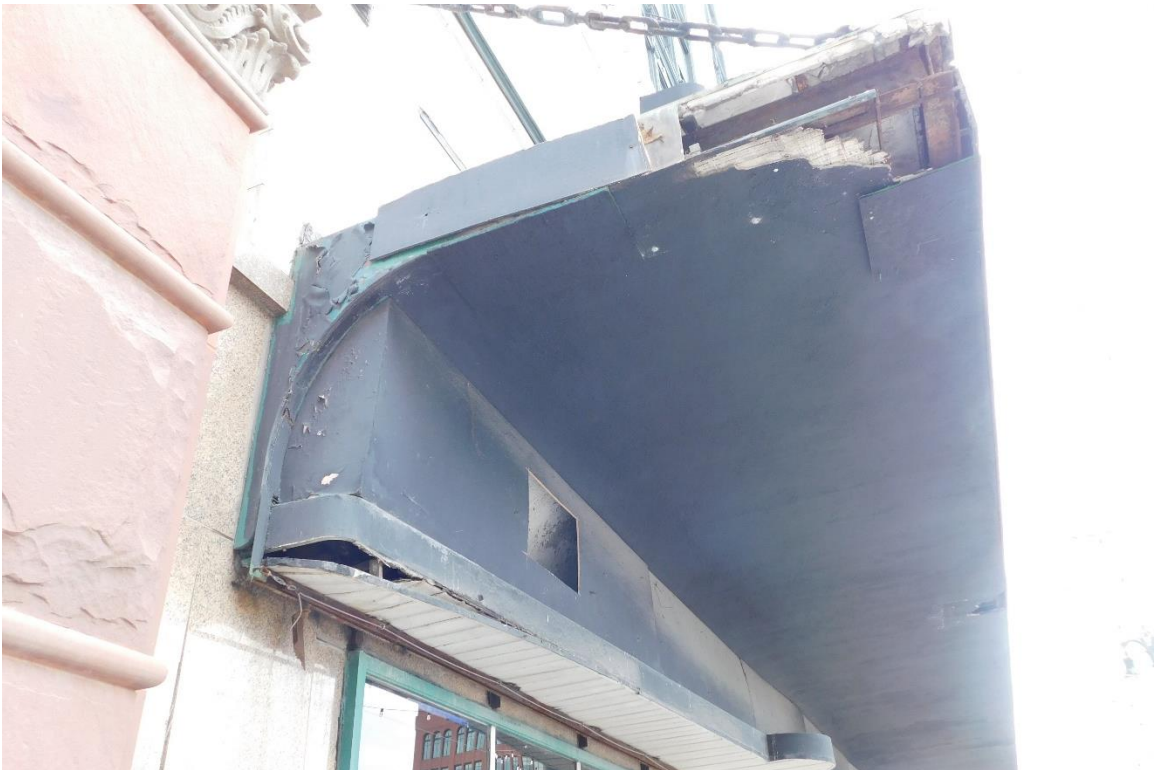
Figure #26: Exterior, Canopy, Looking Northwest. 7/17/19
