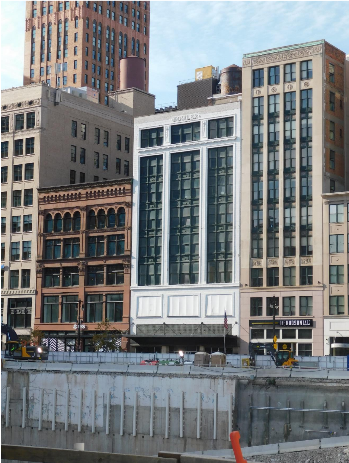
Exterior #2: Exterior, Looking Southwest. 10/15/2019
