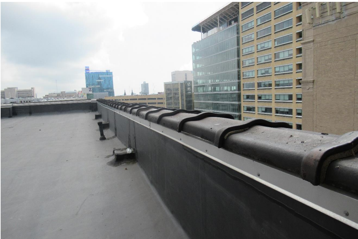
Figure #85: Exterior, Roof, Looking East. 7/17/19
