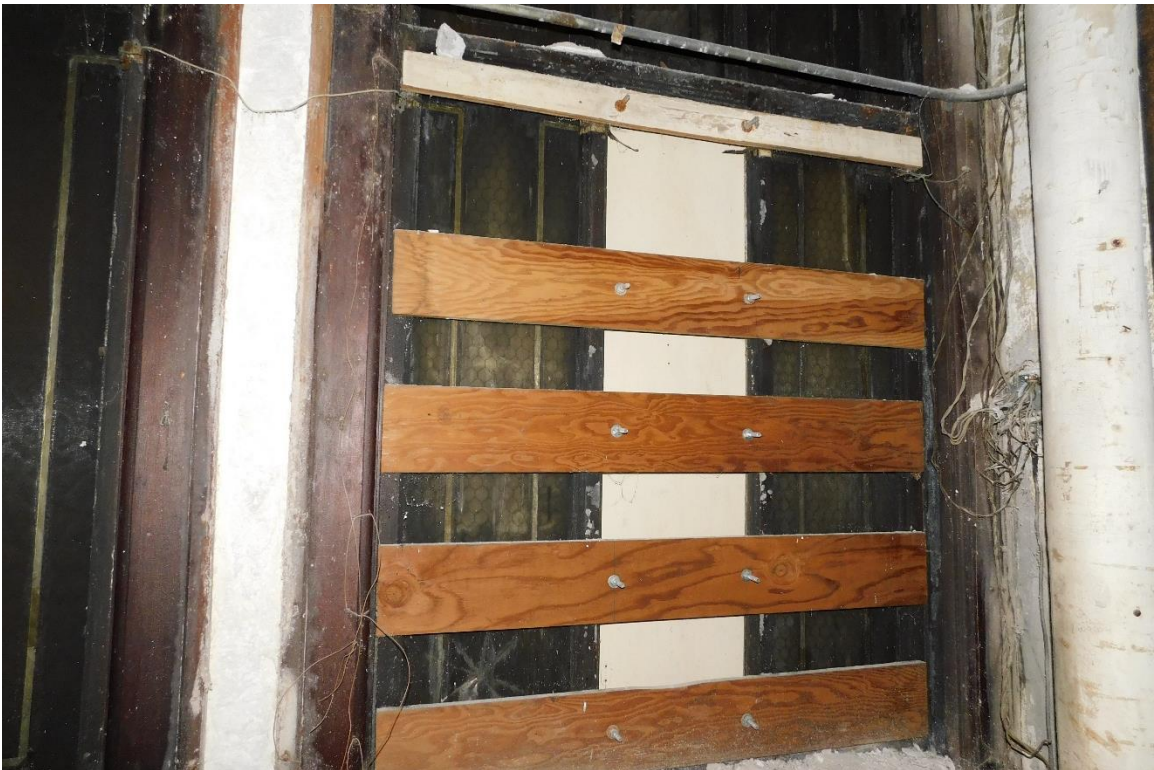
Figure #83: Interior, 8 th floor, Window Detail. 10/15/19
