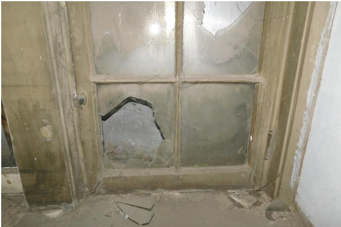
Figure #57: Interior, 2 nd floor, Window Detail. 10/15/19
