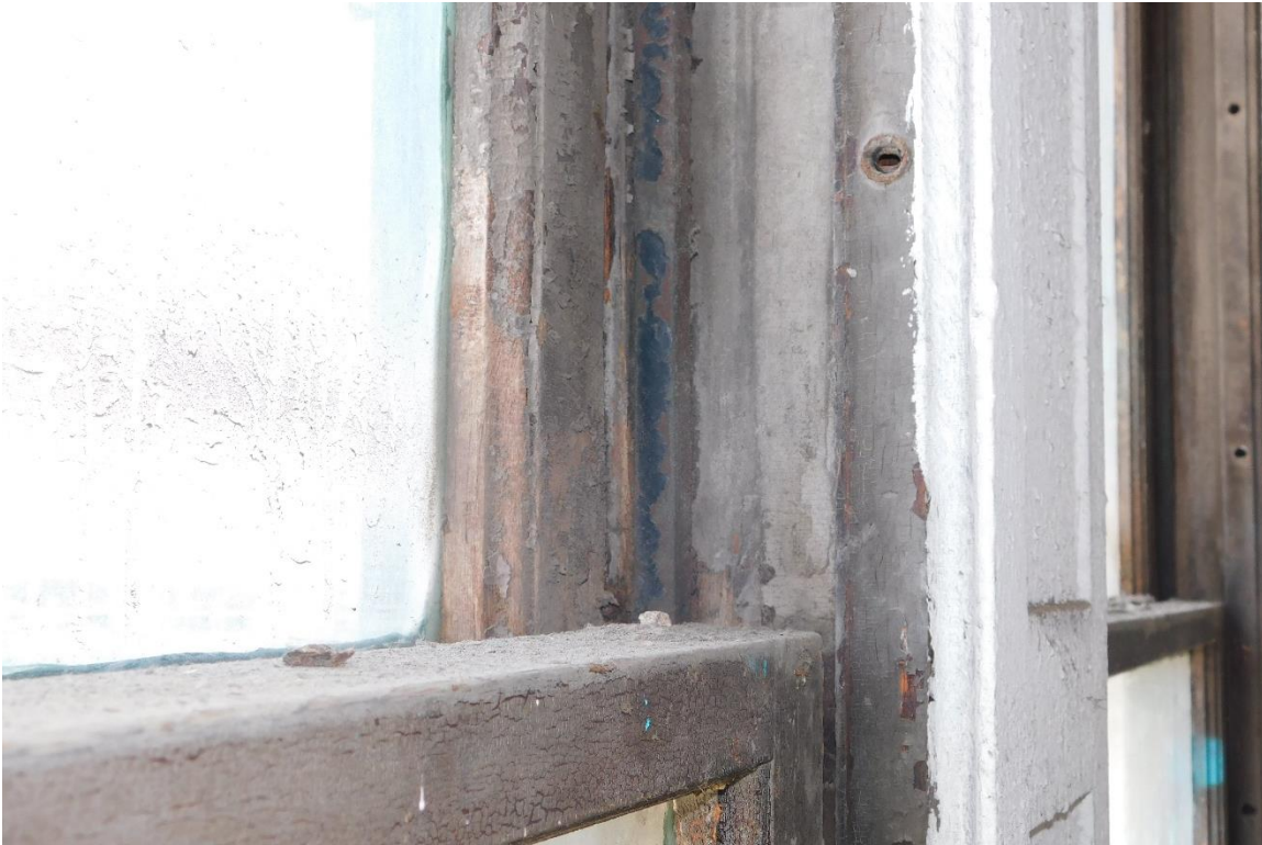
Figure #65: Interior, 3 rd floor, Window Detail. 10/15/19
