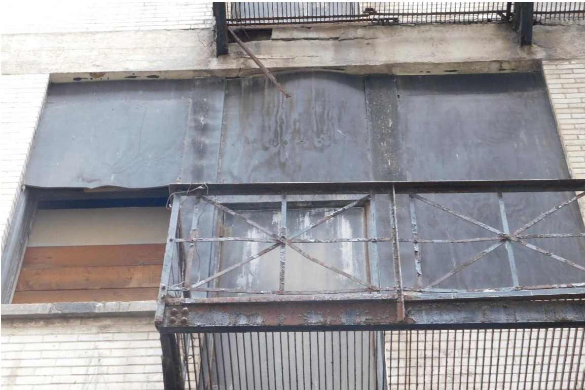
Figure #45: Exterior, Fire Escape, Looking Up. 10/15/19
