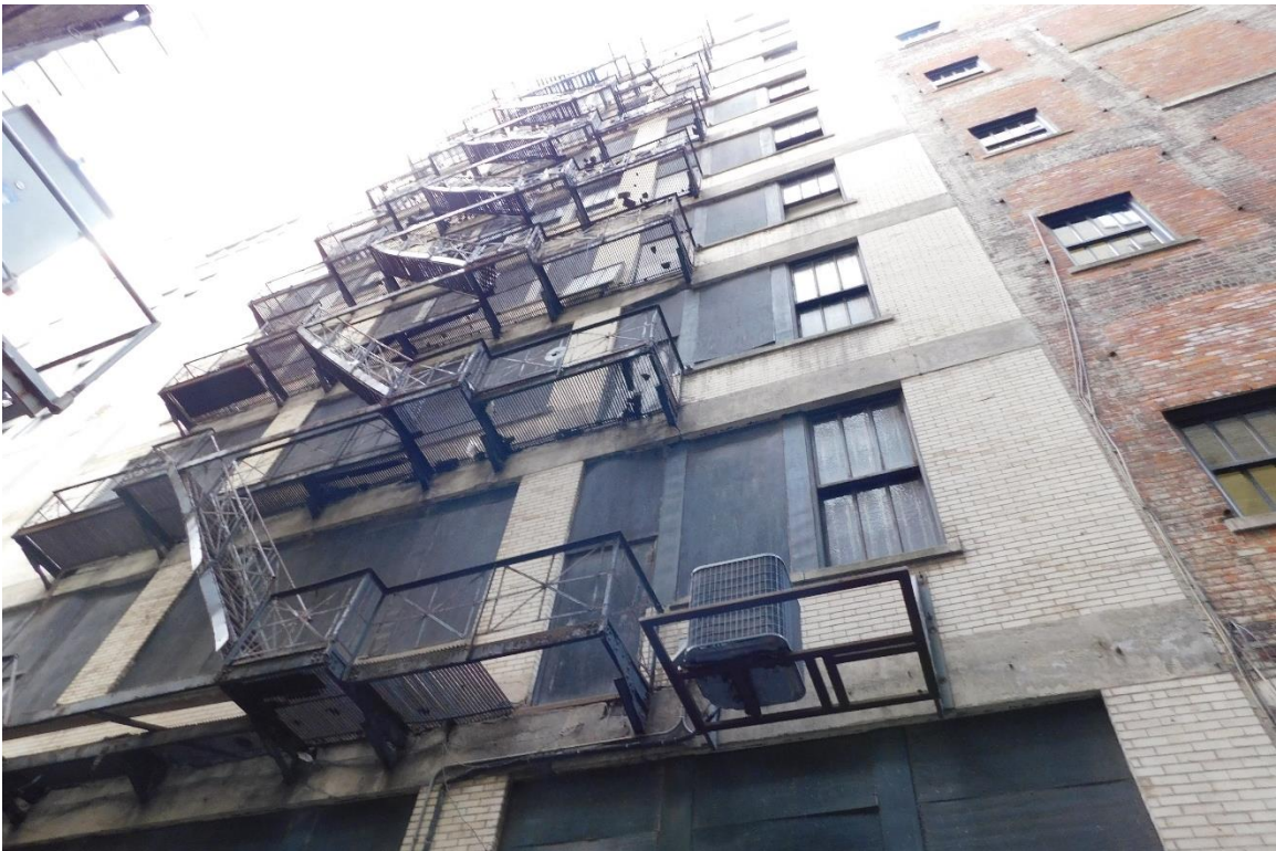
Figure #38: Exterior, Alley Façade, Looking Up. 10/15/19
