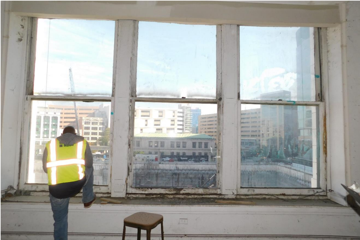
Figure #61: Interior, 3 rd Floor, Looking East. 10/15/19
