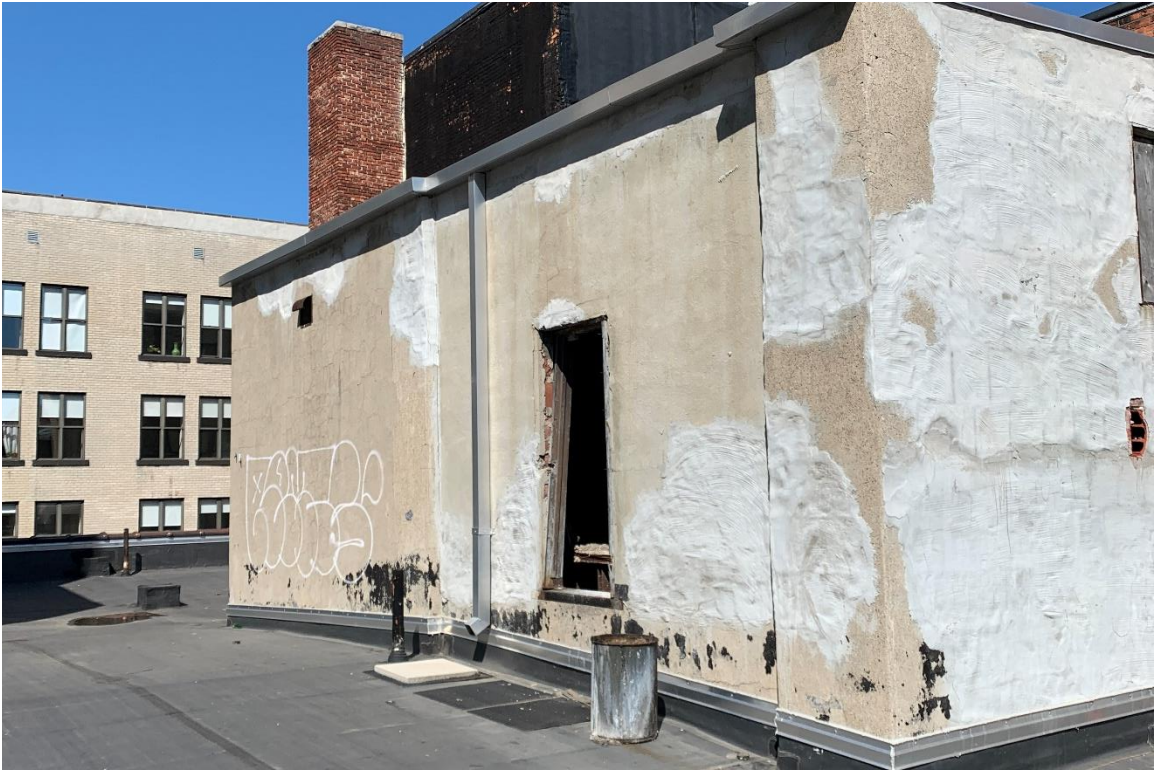
Figure #89: Exterior, Roof and Penthouse, Looking Northwest. 6/12/20
