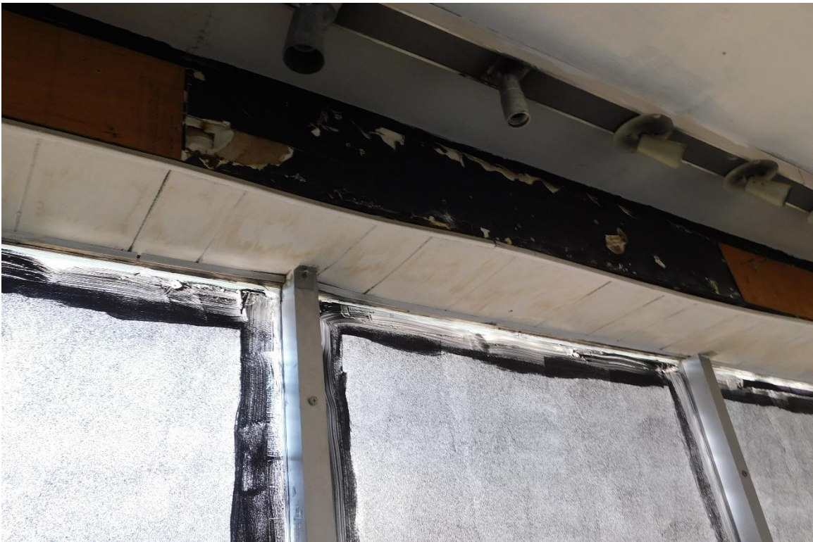
Figure #49: Interior, 1 st Floor Storefront, Looking Up. 10/15/19
