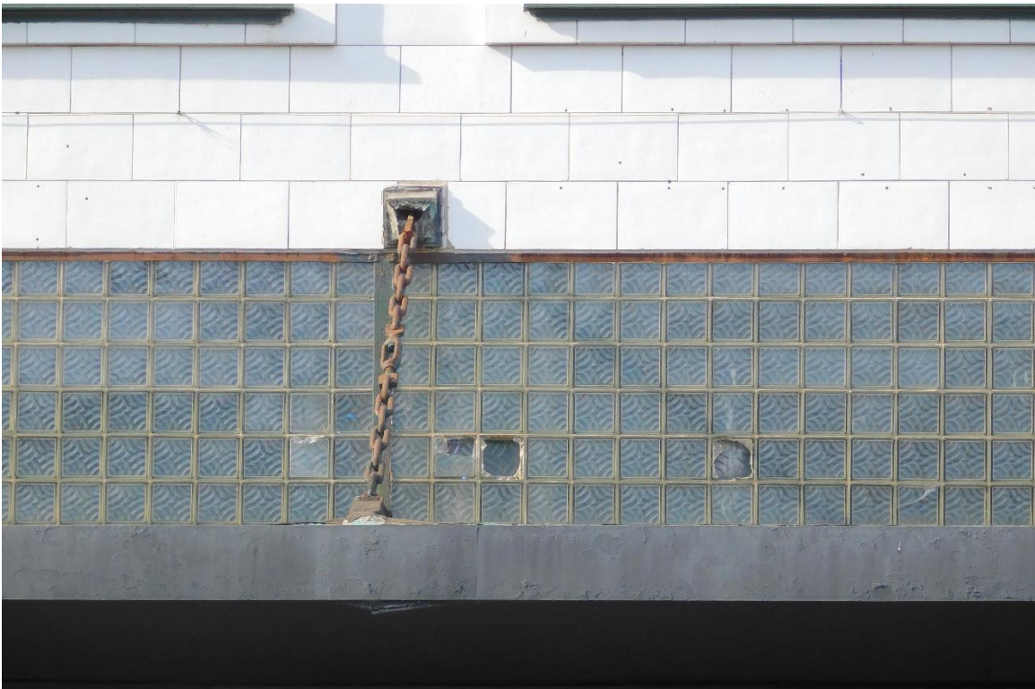
Figure #28: Exterior, Mezzanine Glass Block, Looking West. 10/15/19
