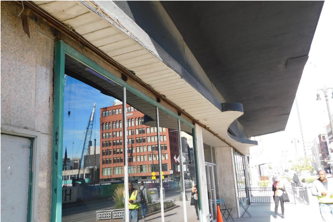
Figure #29: Exterior, Storefront and Canopy Detail, Looking Northwest. 10/15/19
