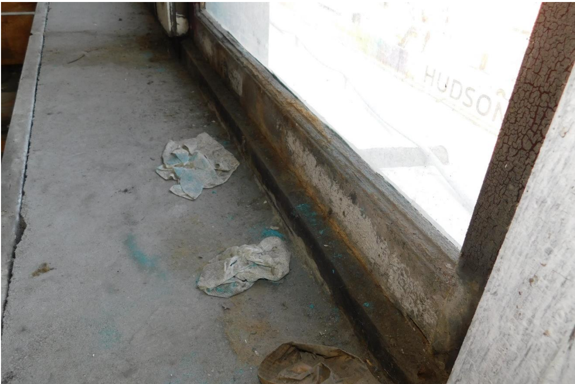
Figure #64: Interior, 3 rd Floor, Window Detail. 10/15/19
