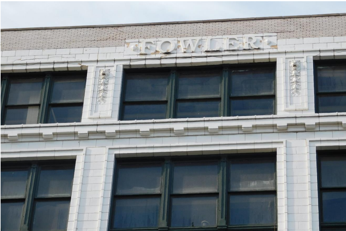
Figure #7: Exterior, Looking Up. 10/15/19
