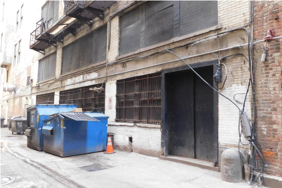
Figure #35: Exterior, Alley Façade, Looking Northeast. 10/15/19
