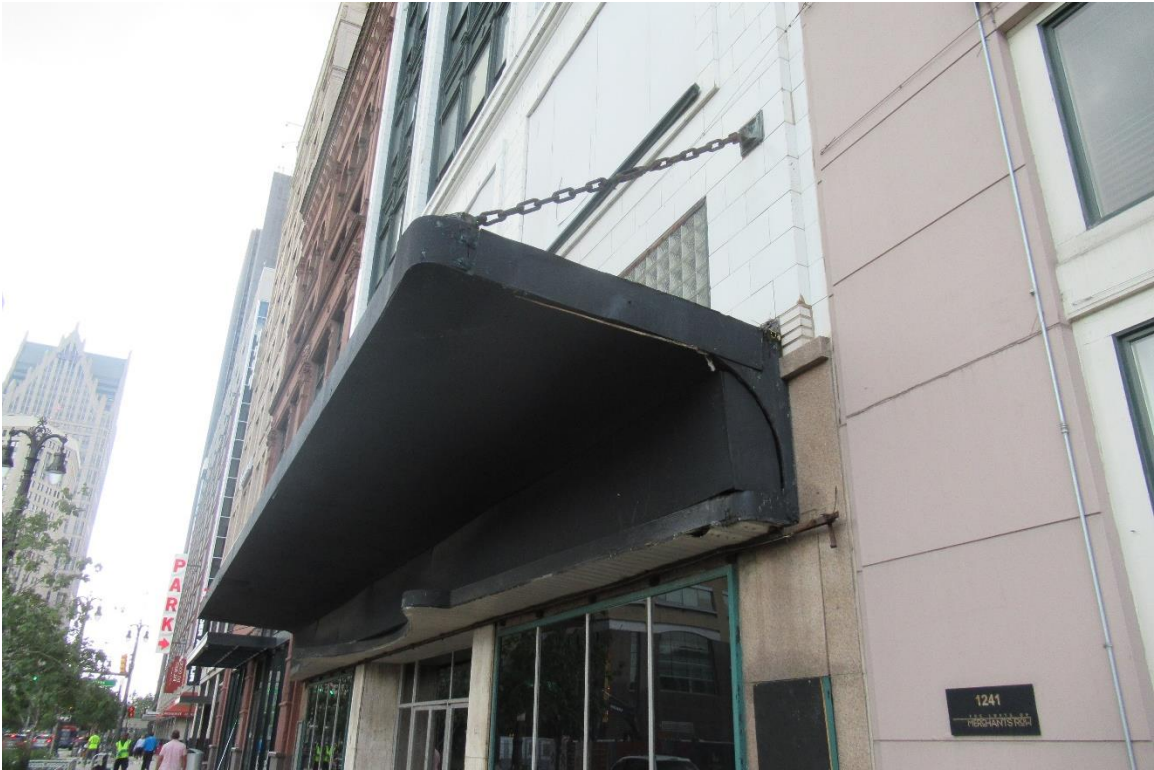
Figure #18: Exterior, Looking Up. 7/17/19
