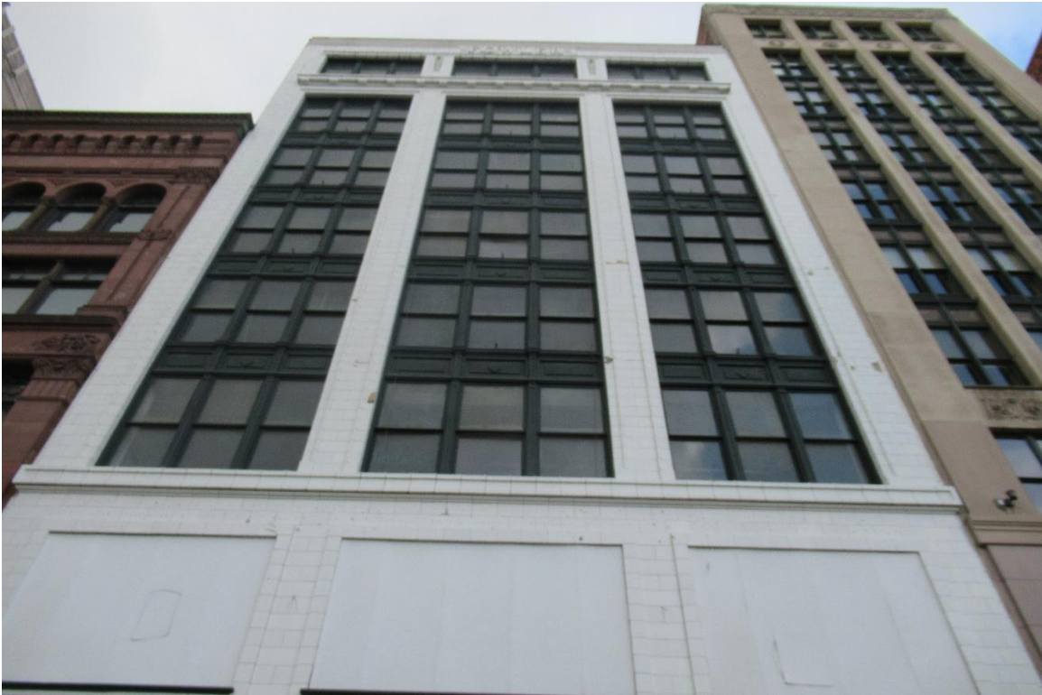
Figure #4: Exterior, Looking up. 7/17/19
