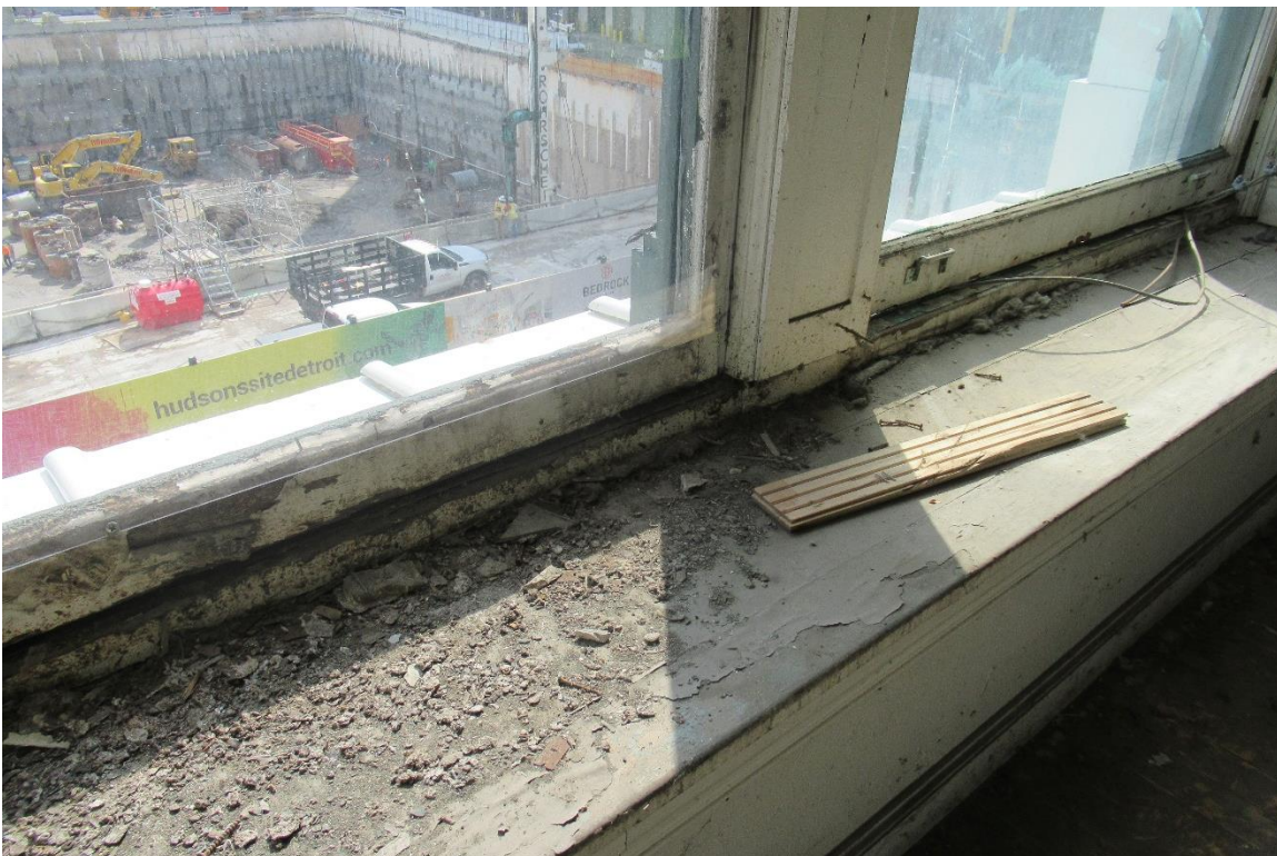
Figure #66: Interior, 3 rd floor, Window Detail. 7/17/19
