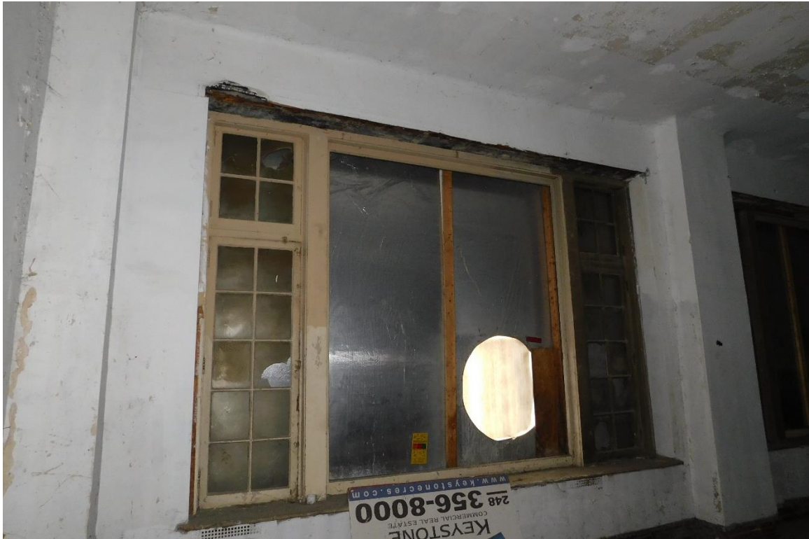
Figure #56: Interior, 2 nd floor, Looking East. 10/15/19
