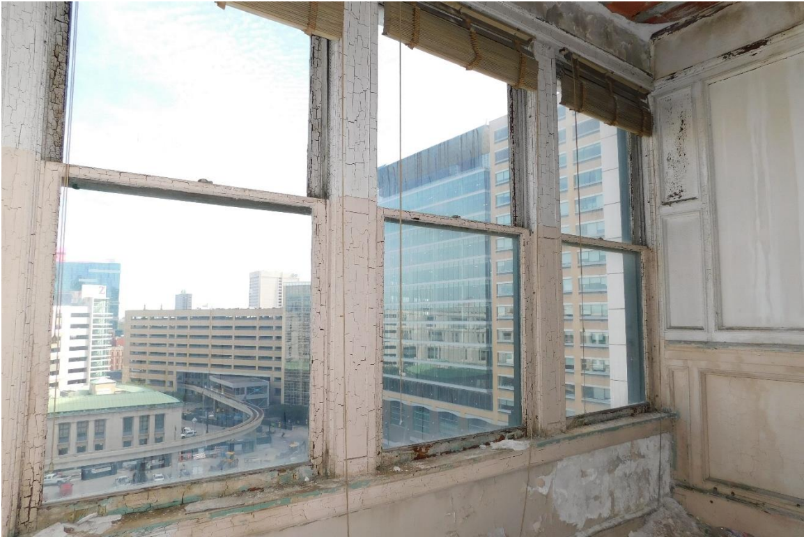
Figure #80: Interior, 8 th floor, Looking Southeast. 10/15/19
