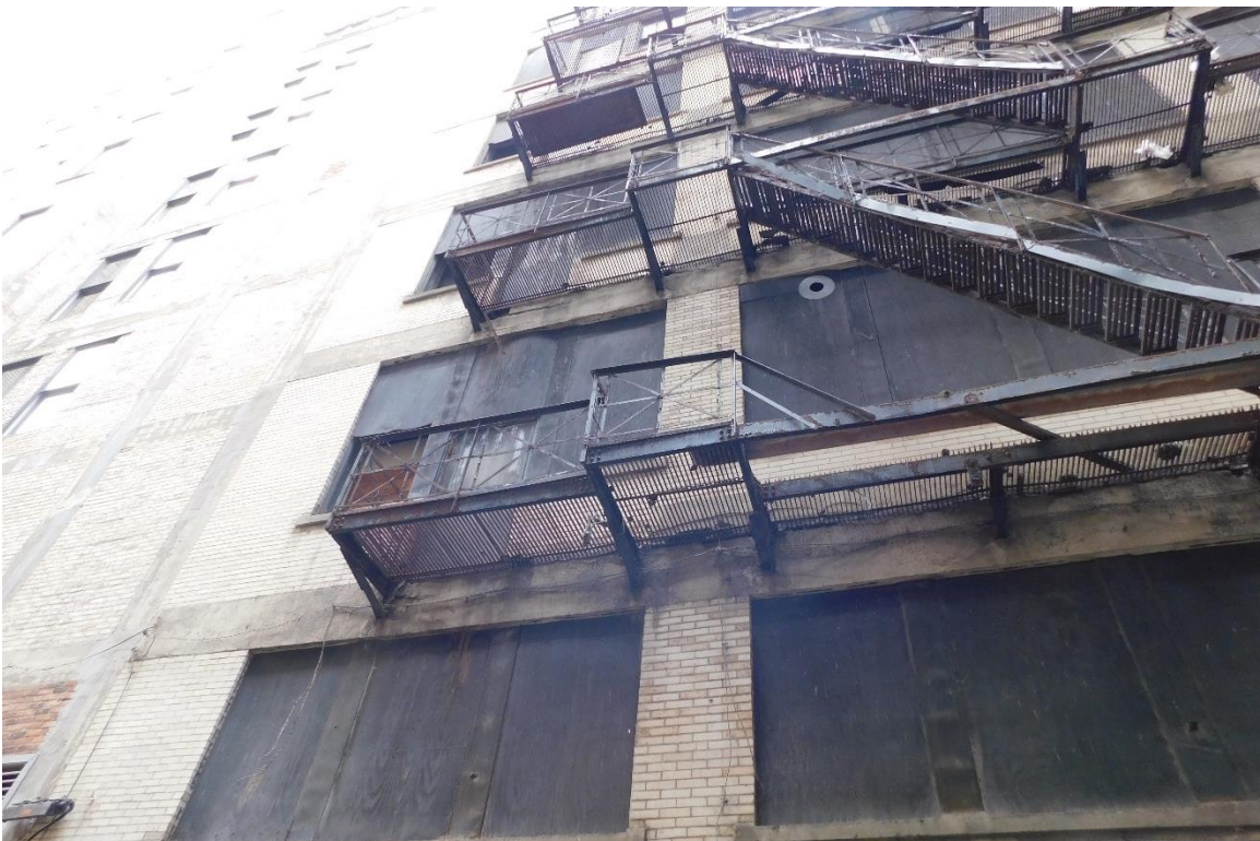
Figure #41: Exterior, Alley Façade, Looking Up. 10/15/19
