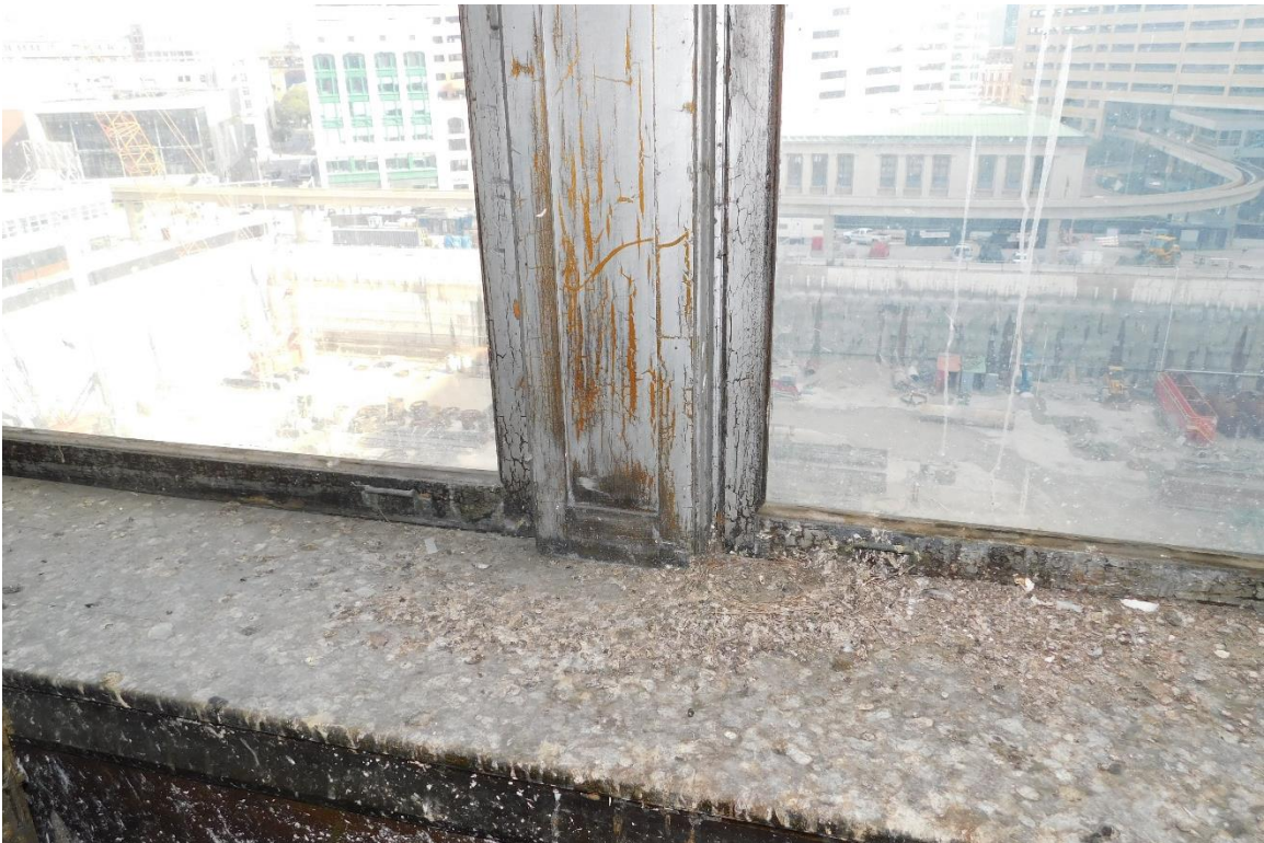
Figure #77: Interior, 6 th floor, Window Detail, Looking Down. 10/15/19
