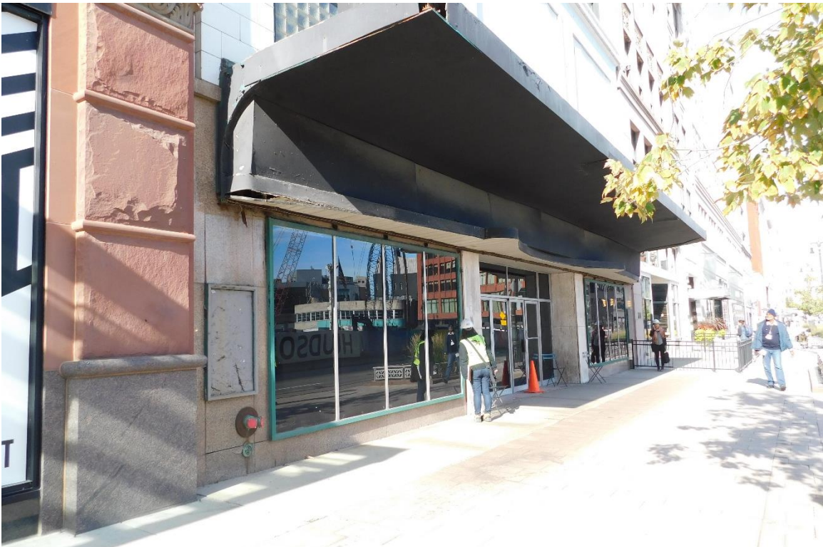
Figure #30: Exterior, Looking Northwest. 10/15/19
