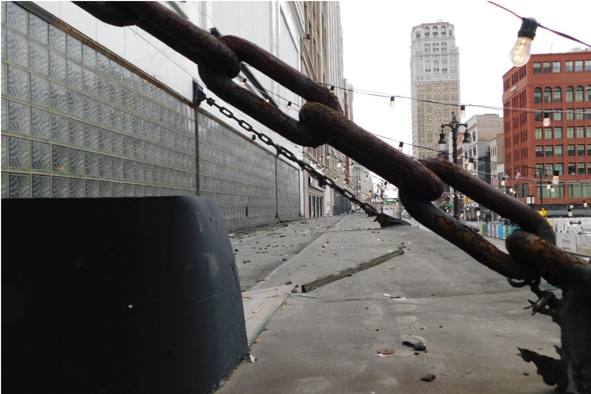
Figure #25: Exterior, Canopy, Looking North. 10/15/19
