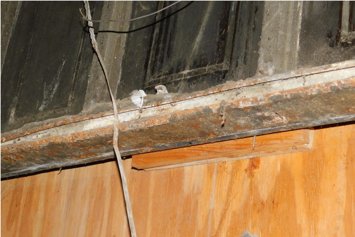
Figure #72: Interior, 4 th floor, Window Detail. 10/15/19
