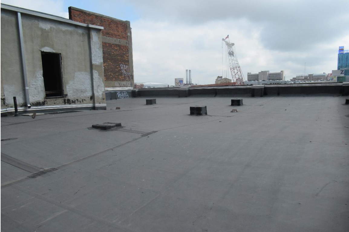
Figure #86: Exterior, Roof, Looking East. 7/17/19
