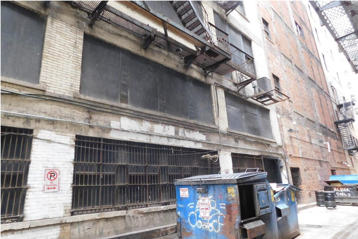
Figure #42: Exterior, Alley Façade, Looking Southeast. 10/15/19
