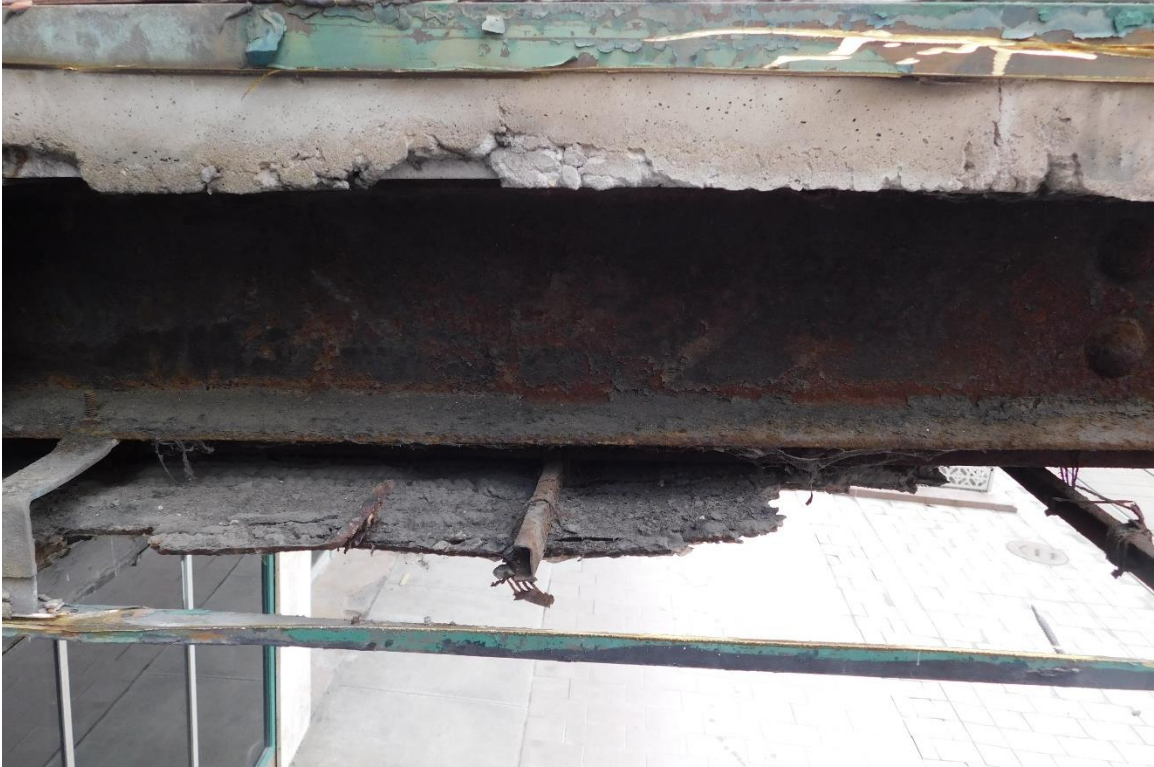
Figure #23: Exterior, Canopy Detail, Looking North. 10/15/19
