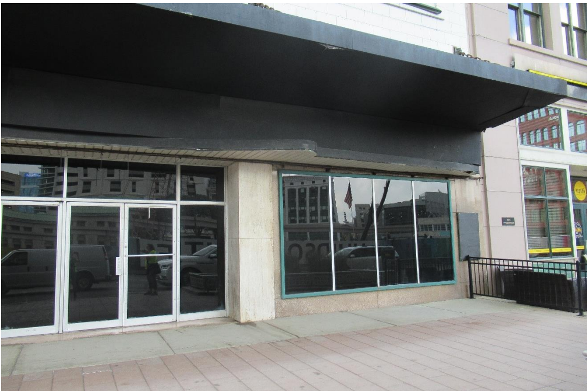
Figure #19: Exterior, Looking Northwest. 7/17/19
