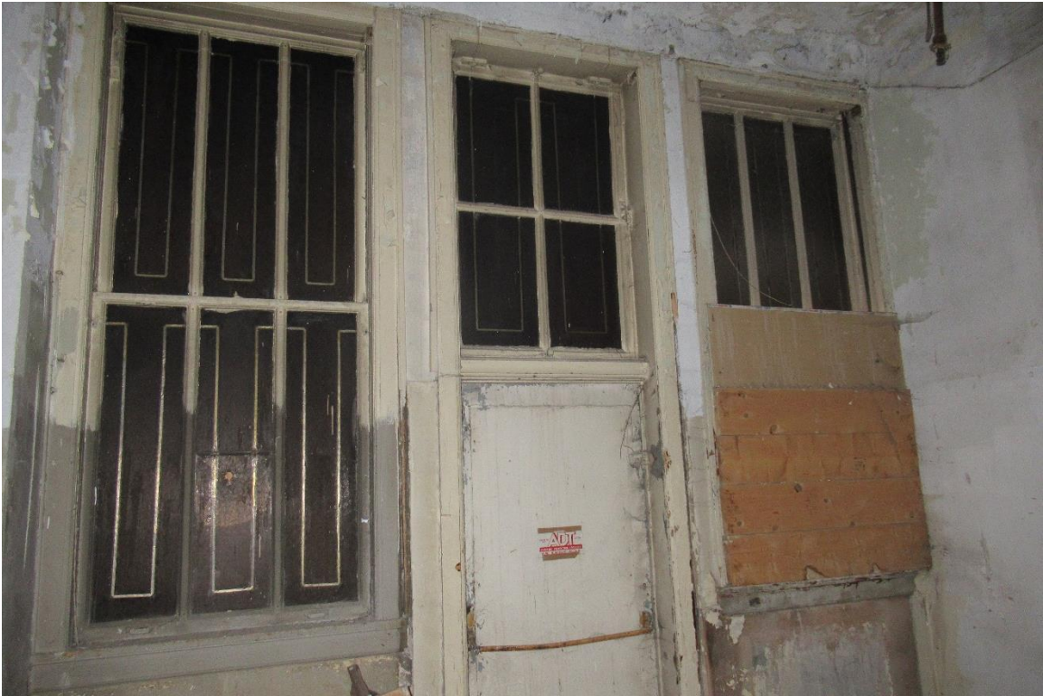
Figure #58: Interior, 2 nd floor, Looking West. 7/17/19
