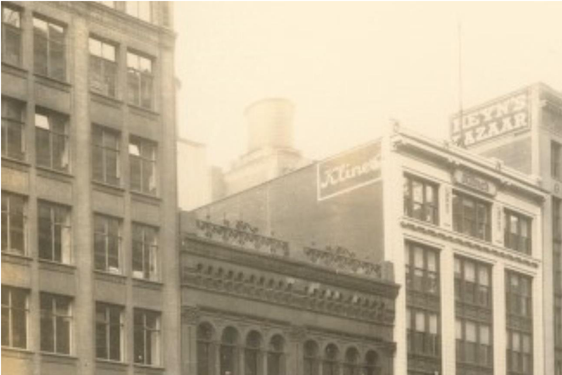
Figure #93: Cornice detail zoomed in from previous photo #92 – 1920s
