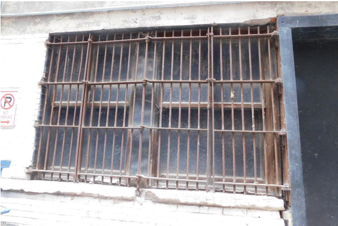
Figure #36: Exterior, Alley Façade Window, Looking East. 10/15/19
