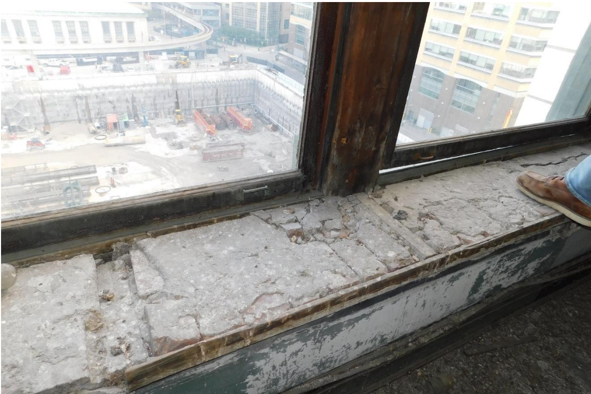
Figure #79: Interior, 7 th floor, Looking Down. 10/15/19
