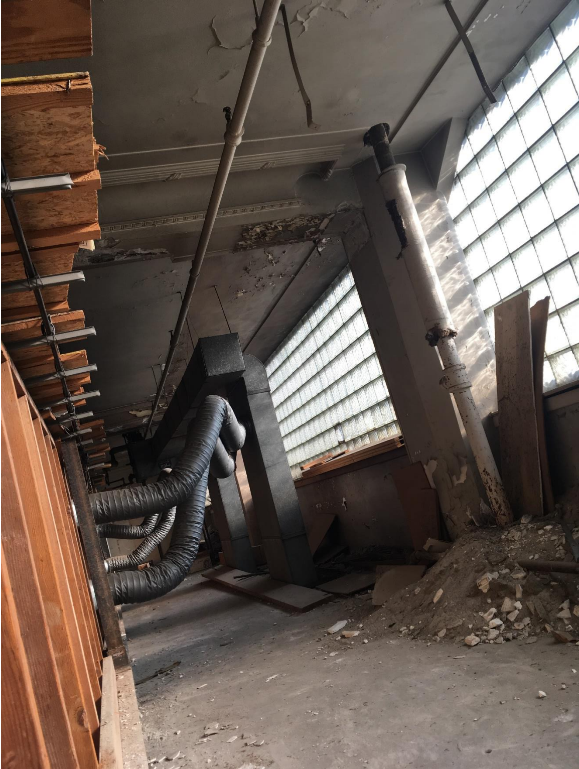
Figure #51: Interior, Mezzanine Windows, Looking Northeast. 5/31/19
