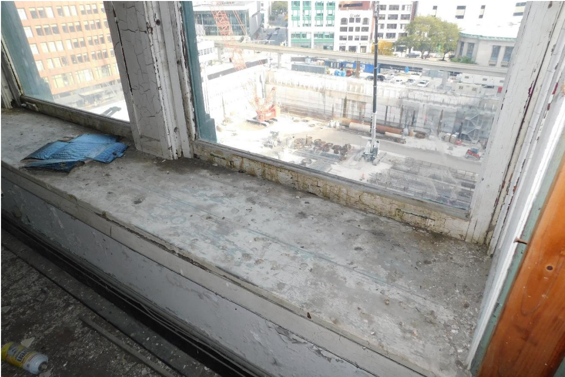
Figure #78: Interior, 7 th floor, Window Detail. 10/15/19
