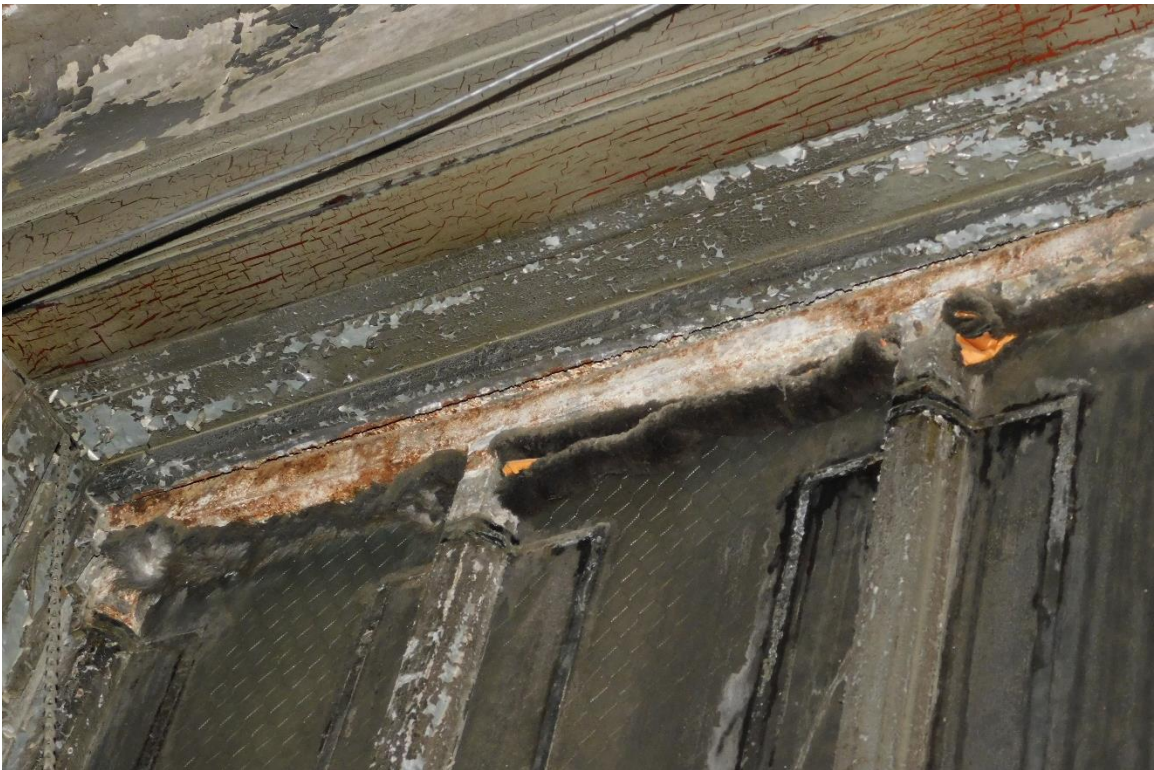
Figure #71: Interior, 4 th floor, Window Detail. 10/15/19
