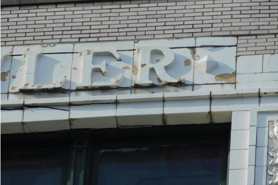
Figure #10: Exterior, Detail, Looking Up. 10/15/19
