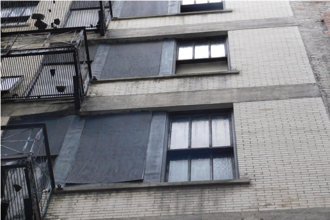
Figure #46: Exterior, Alley Façade, Looking Up. 10/15/19
