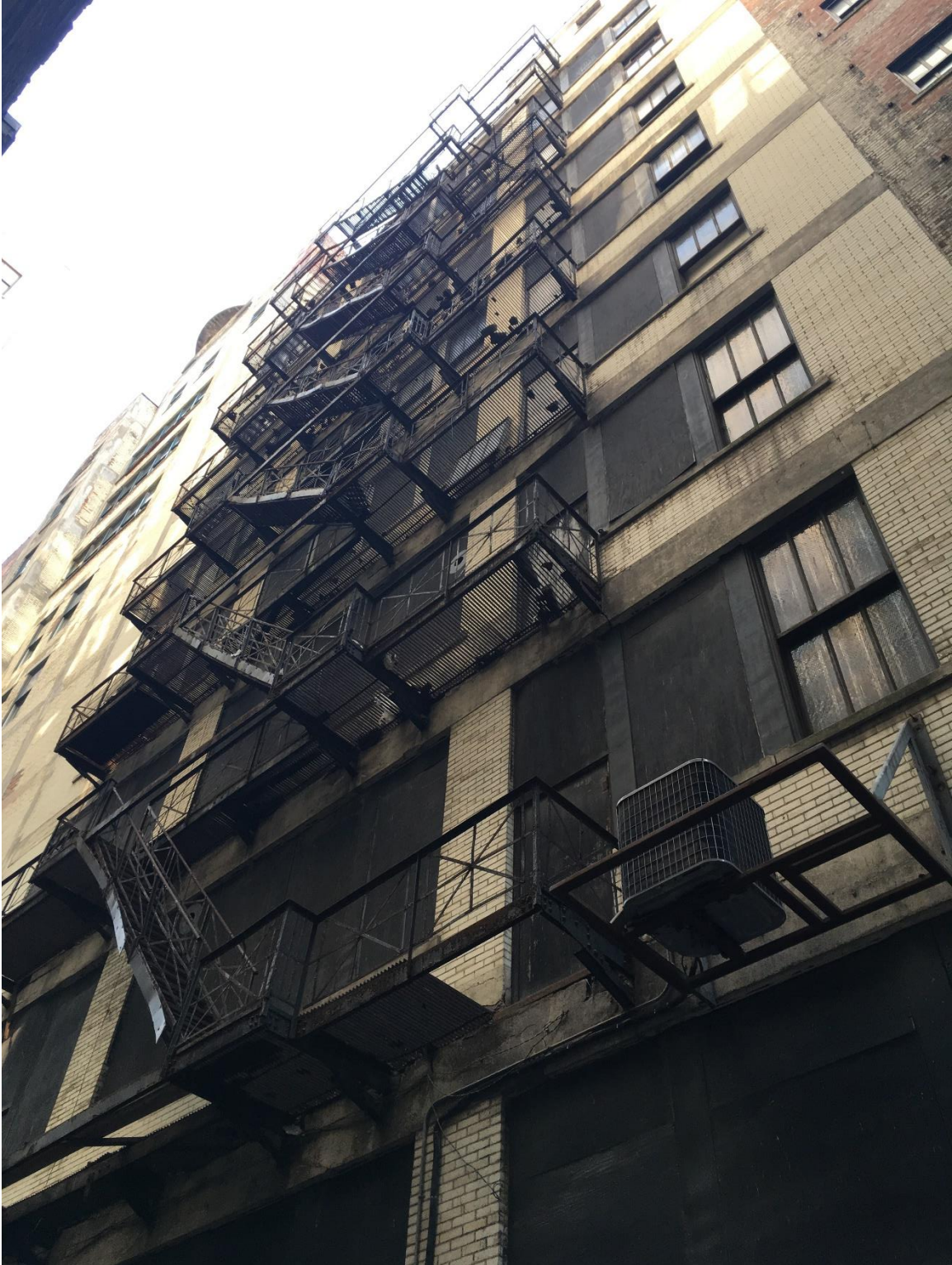
Figure #33: Exterior, Alley, Looking Up. 5/31/19
