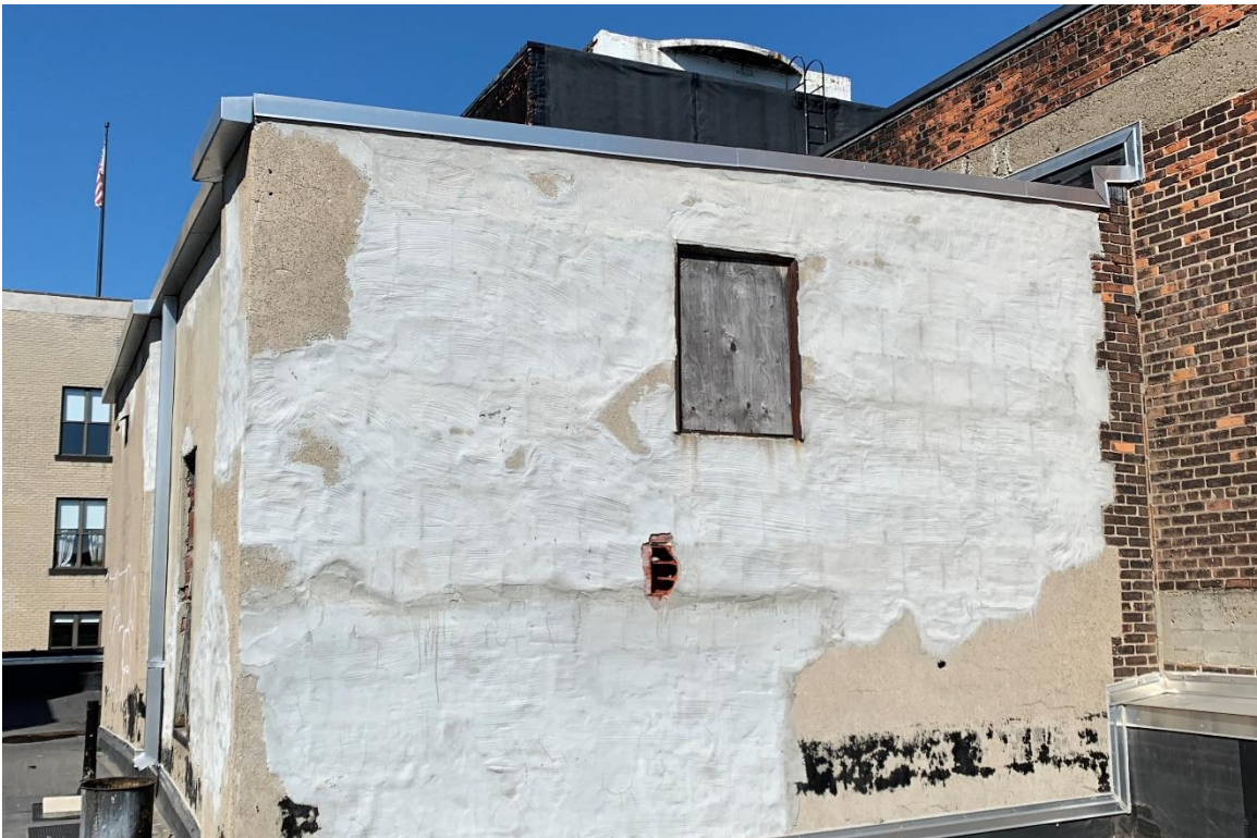
Figure #90: Exterior, Penthouse and Roof, Looking West. 6/12/20
