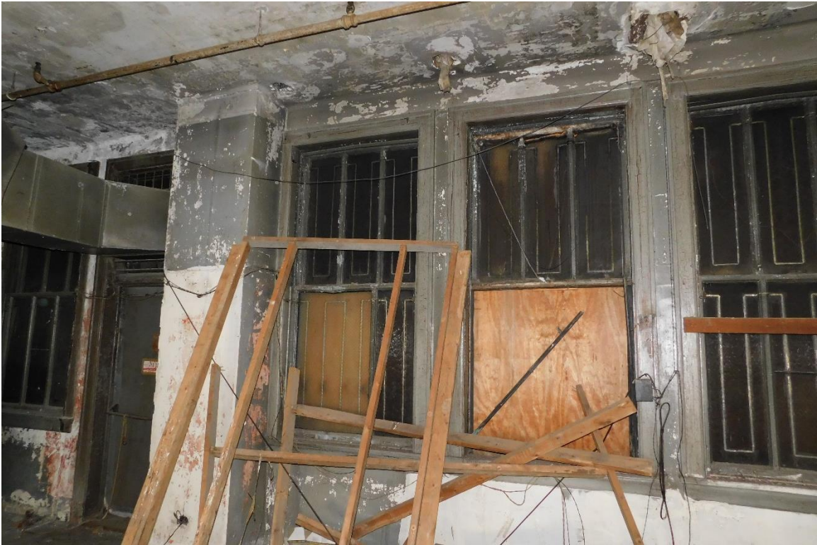
Figure #70: Interior, 4 th floor, Looking East. 10/15/19
