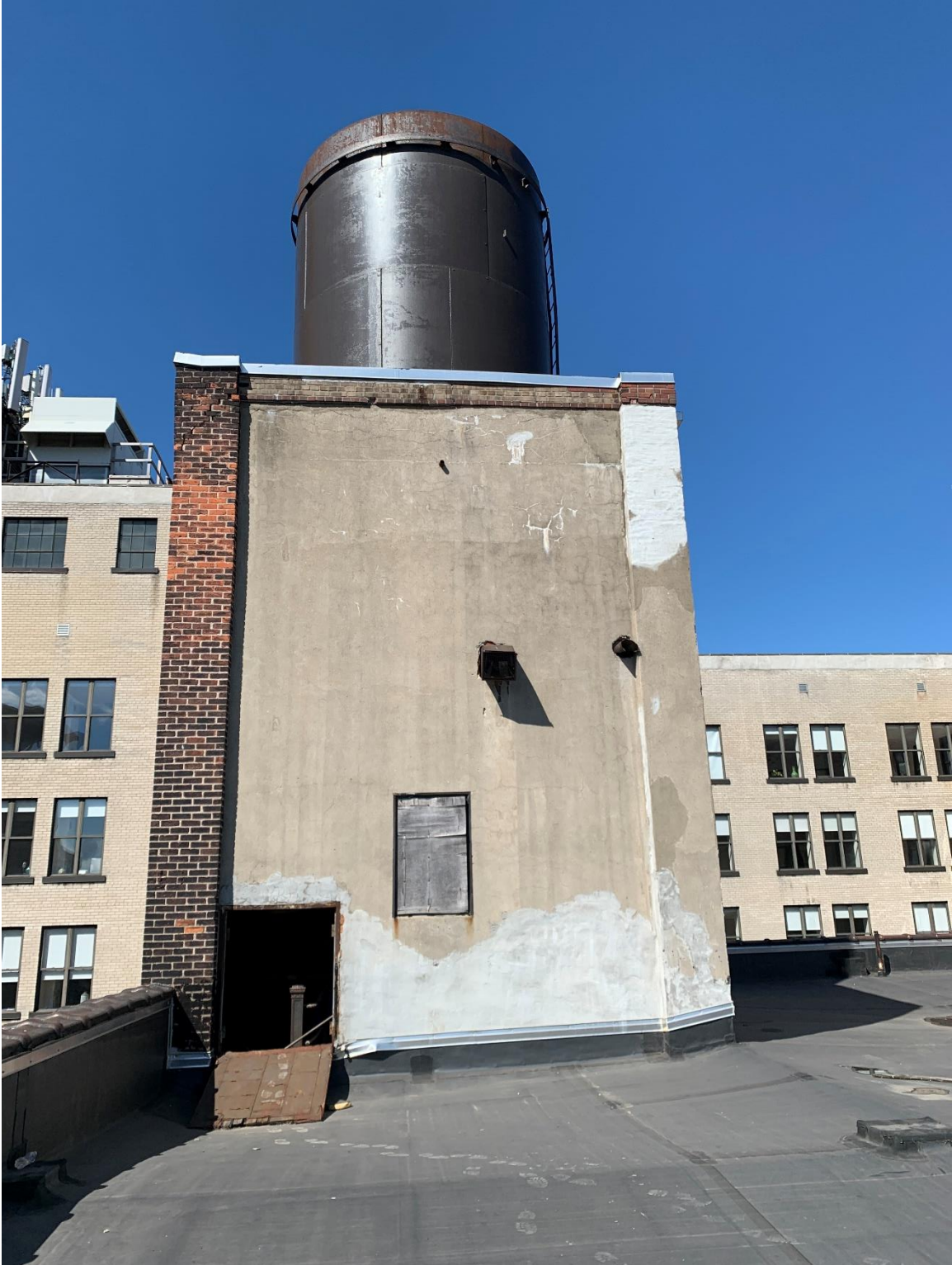
Figure #88: Exterior, Water tower, Looking up. 6/12/20
