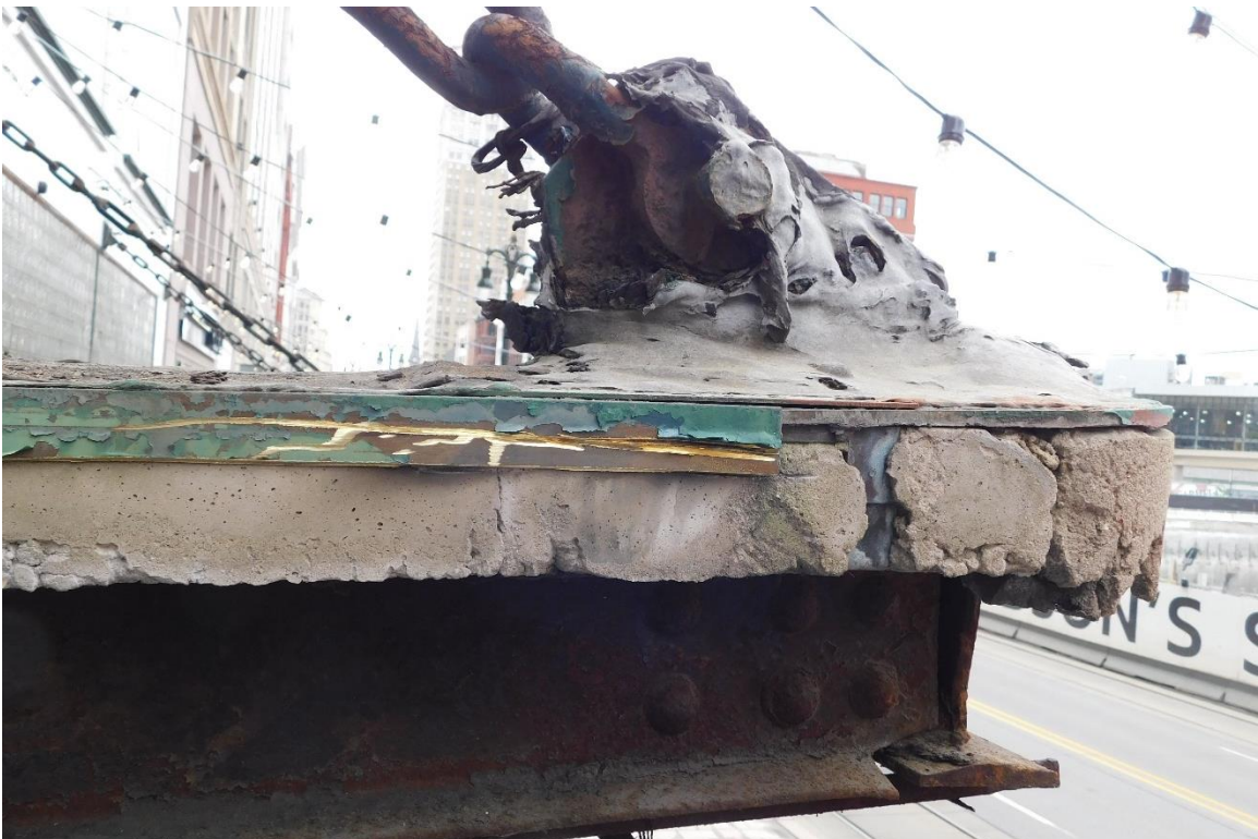
Figure #24: Exterior, Canopy Detail, Looking North. 10/15/19
