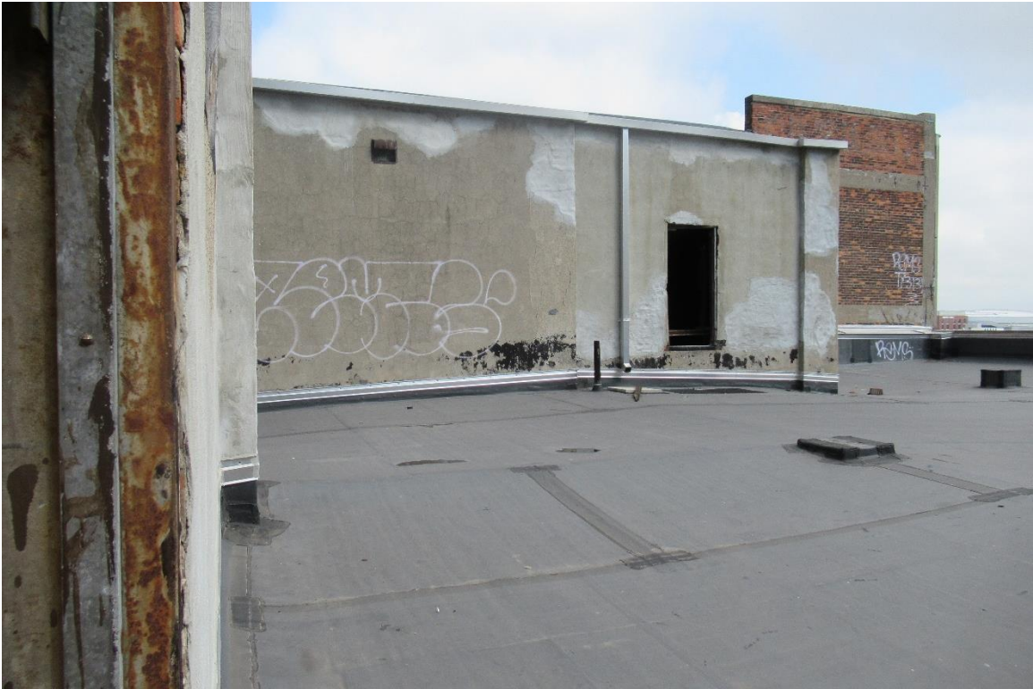
Figure #84: Exterior, Roof, Looking North. 7/17/19
