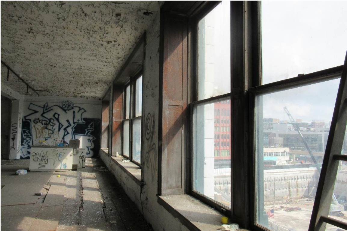
Figure #68: Interior, 4 th floor, Looking Northeast. 5/31/19
