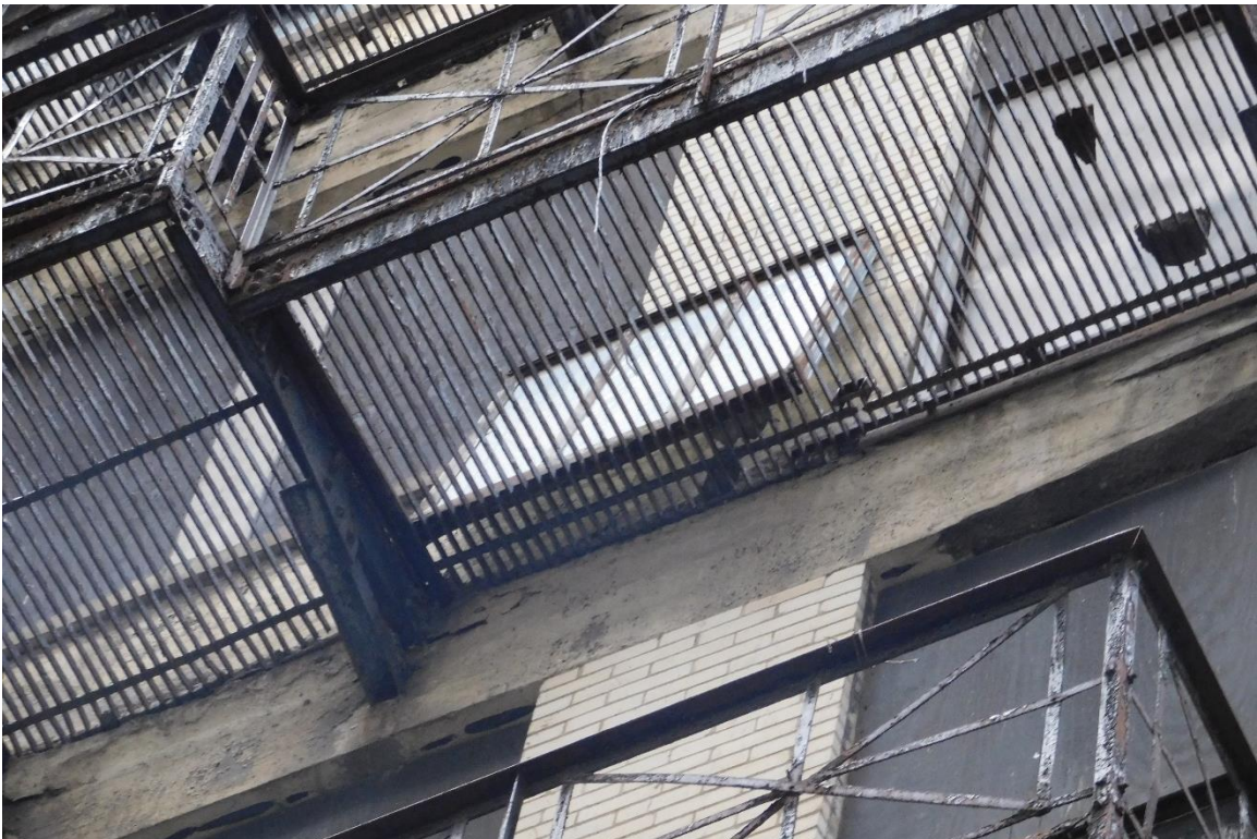
Figure #47: Exterior, Alley Façade and Fire Escape, Looking Up. 10/15/19
