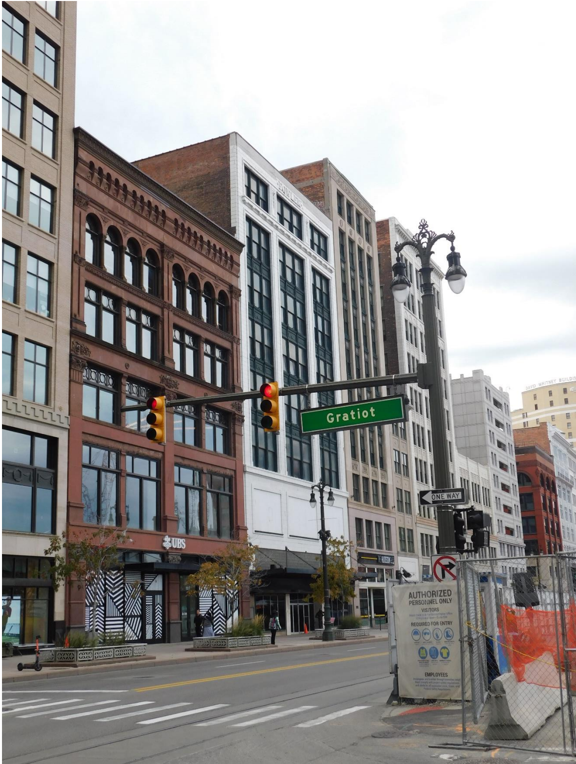
Figure #3: Exterior, Looking Northwest. 10/15/19
