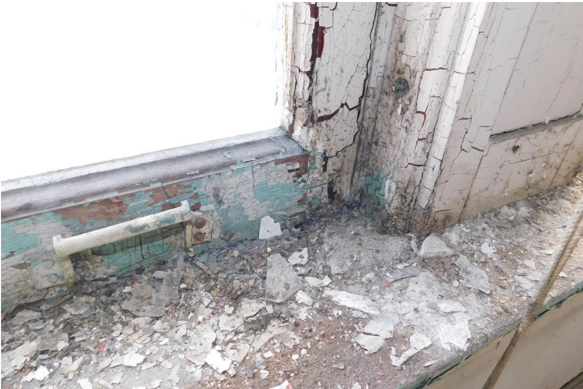
Figure #81: Interior, 8 th floor, Window Detail. 10/15/19
