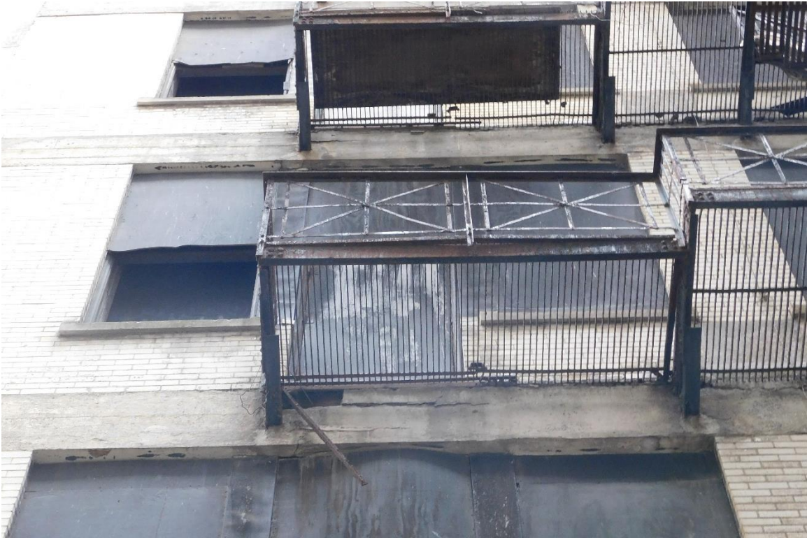
Figure #44: Exterior, Fire Escape, Looking Up. 10/15/19
