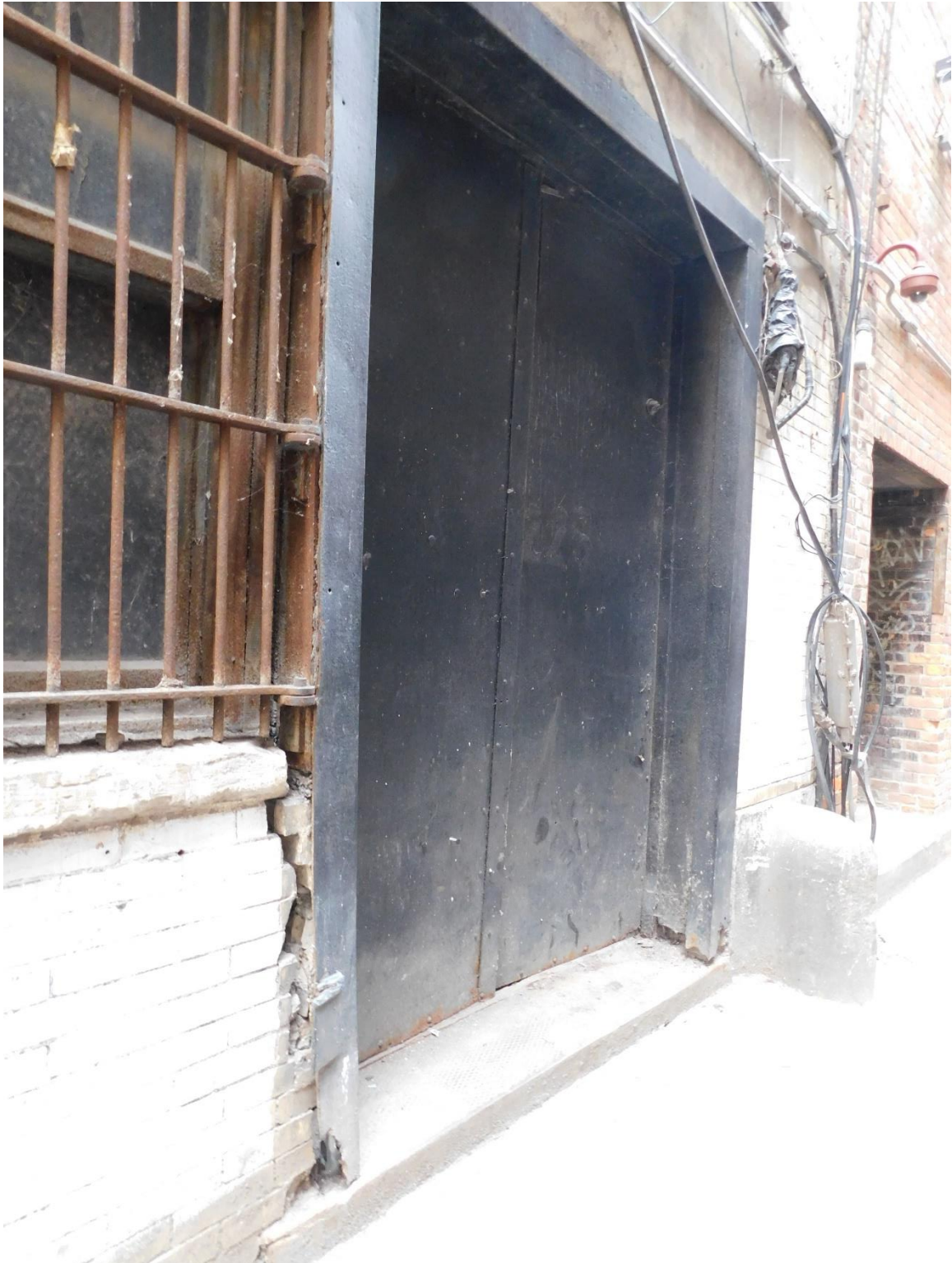
Figure #39: Exterior, Alley Façade Door. 10/15/19
