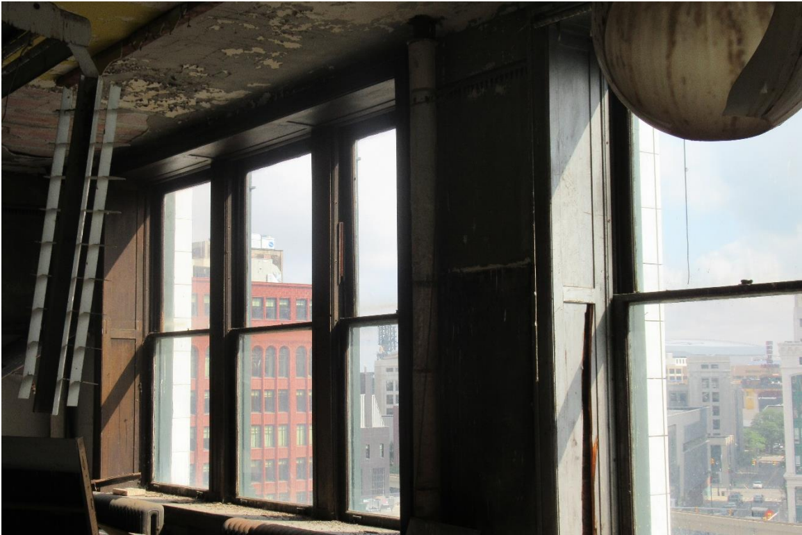
Figure #76: Interior, 6 th floor, Looking Northeast. 7/17/19
