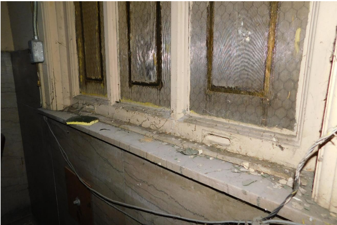
Figure #59: Interior, 2 nd floor, Window Detail. 10/15/19
