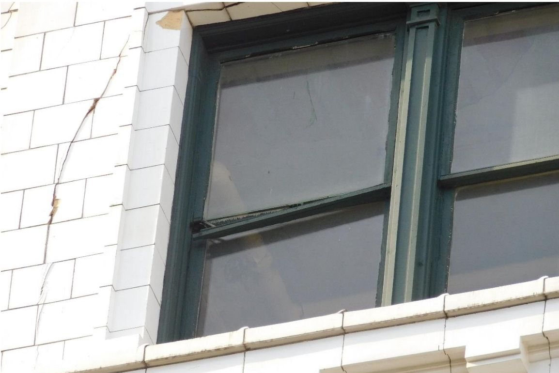
Figure #11: Exterior, Looking Up. 10/15/19
