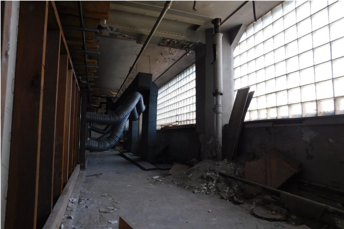
Figure #52: Interior, Mezzanine Glass Block, Looking Northeast. 10/15/19
