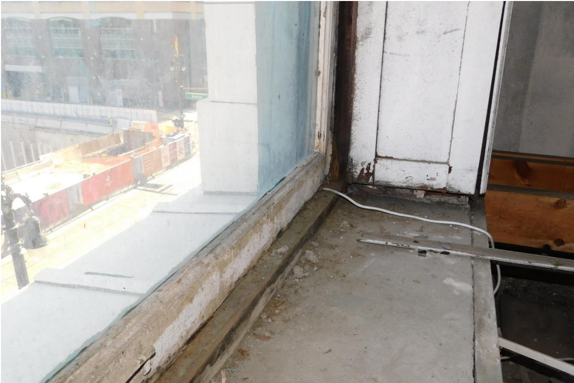
Figure #63: Interior, 3 rd Floor, Window Detail. 10/15/19
