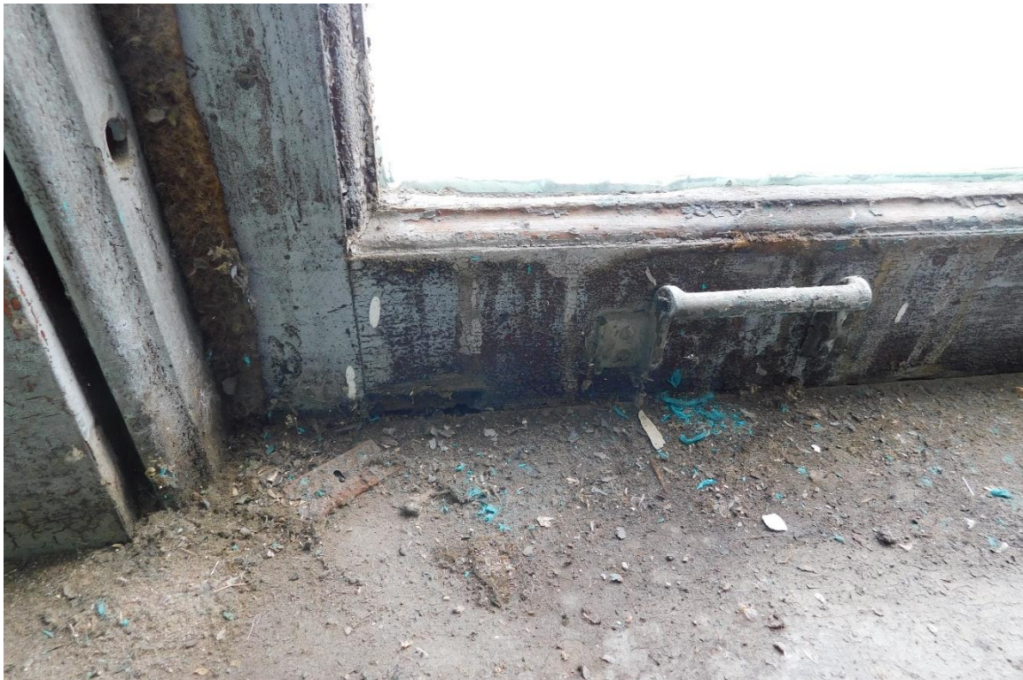
Figure #69: Interior, 4 th floor, Window Detail. 10/15/19
