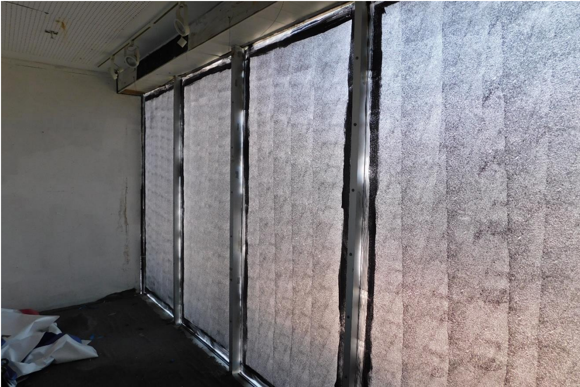
Figure #48: Interior, 1 st Floor Storefront, Looking Northeast. 10/15/19
