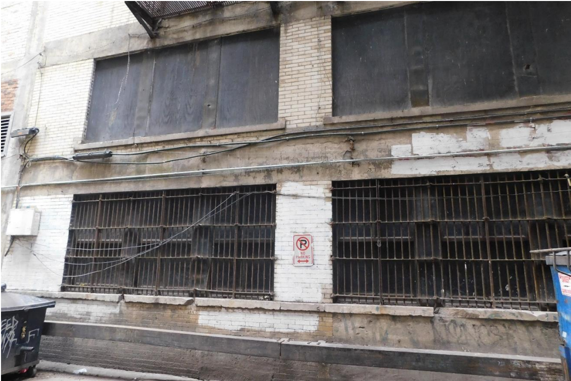
Figure #40: Exterior, Alley façade windows, Looking East. 10/15/19
