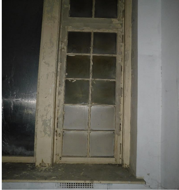
Figure #54: Interior, 2 nd floor, Looking East. 10/15/19
