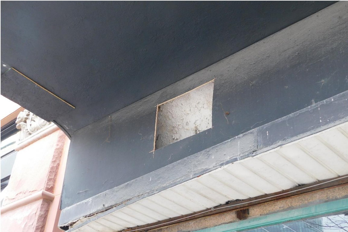
Figure #27: Exterior, Canopy Detail of Plaster Underside, Looking Up. 7/17/19
