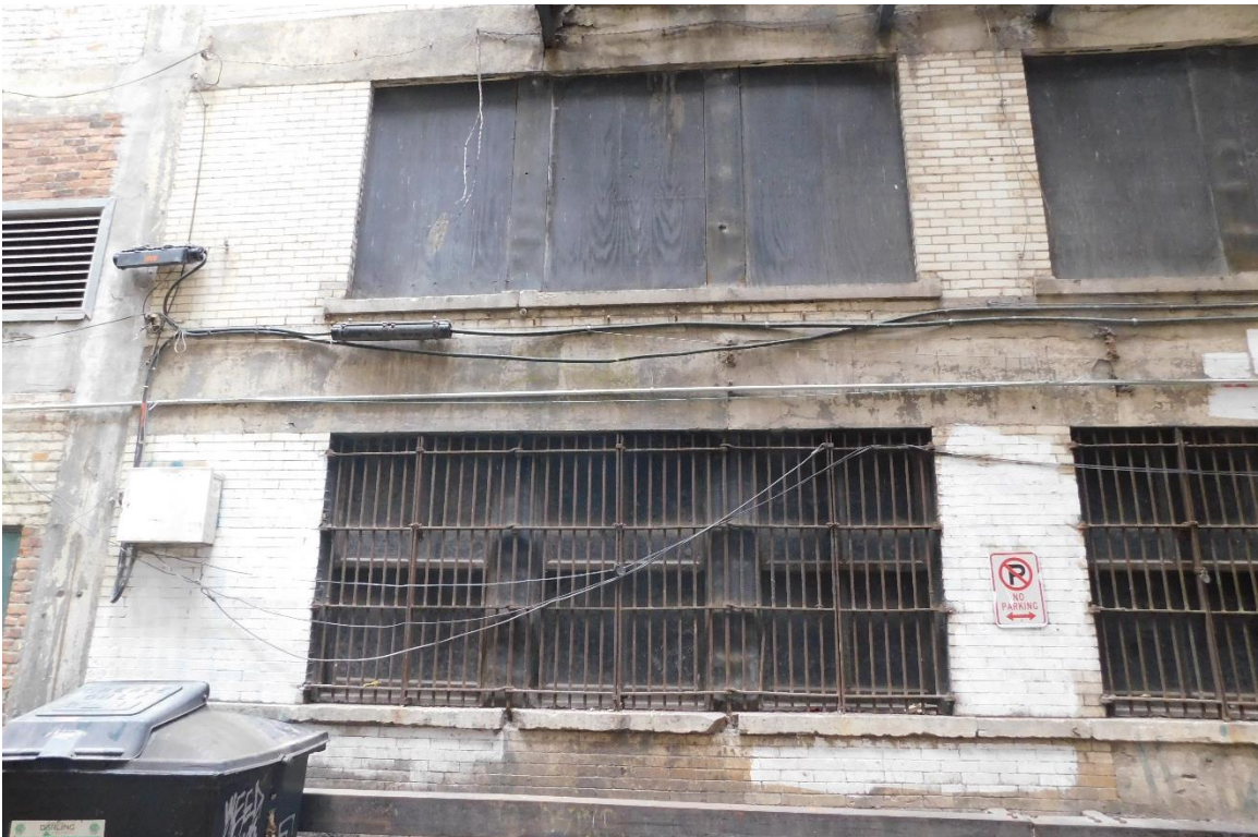
Figure #43: Exterior, Alley Façade, Looking East. 10/15/19
