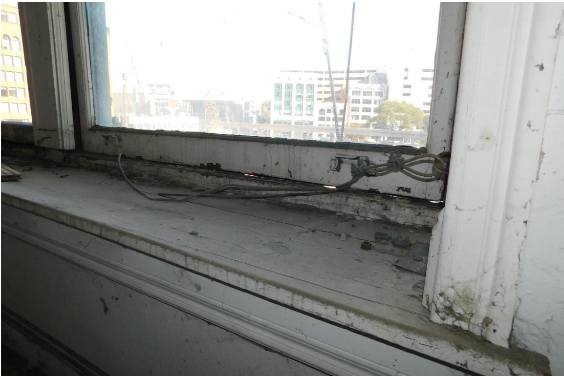
Figure #62: Interior, 3 rd Floor, Window Detail. 10/15/19
