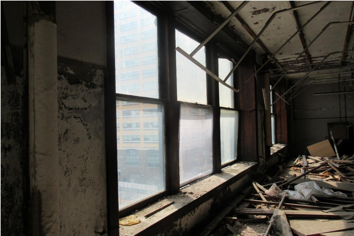
Figure #74: Interior, 5 th floor, Looking southeast. 7/17/19
