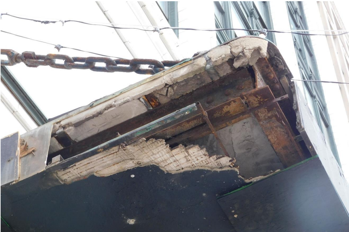
Figure #22: Exterior, Canopy, Looking Up. 10/15/19
