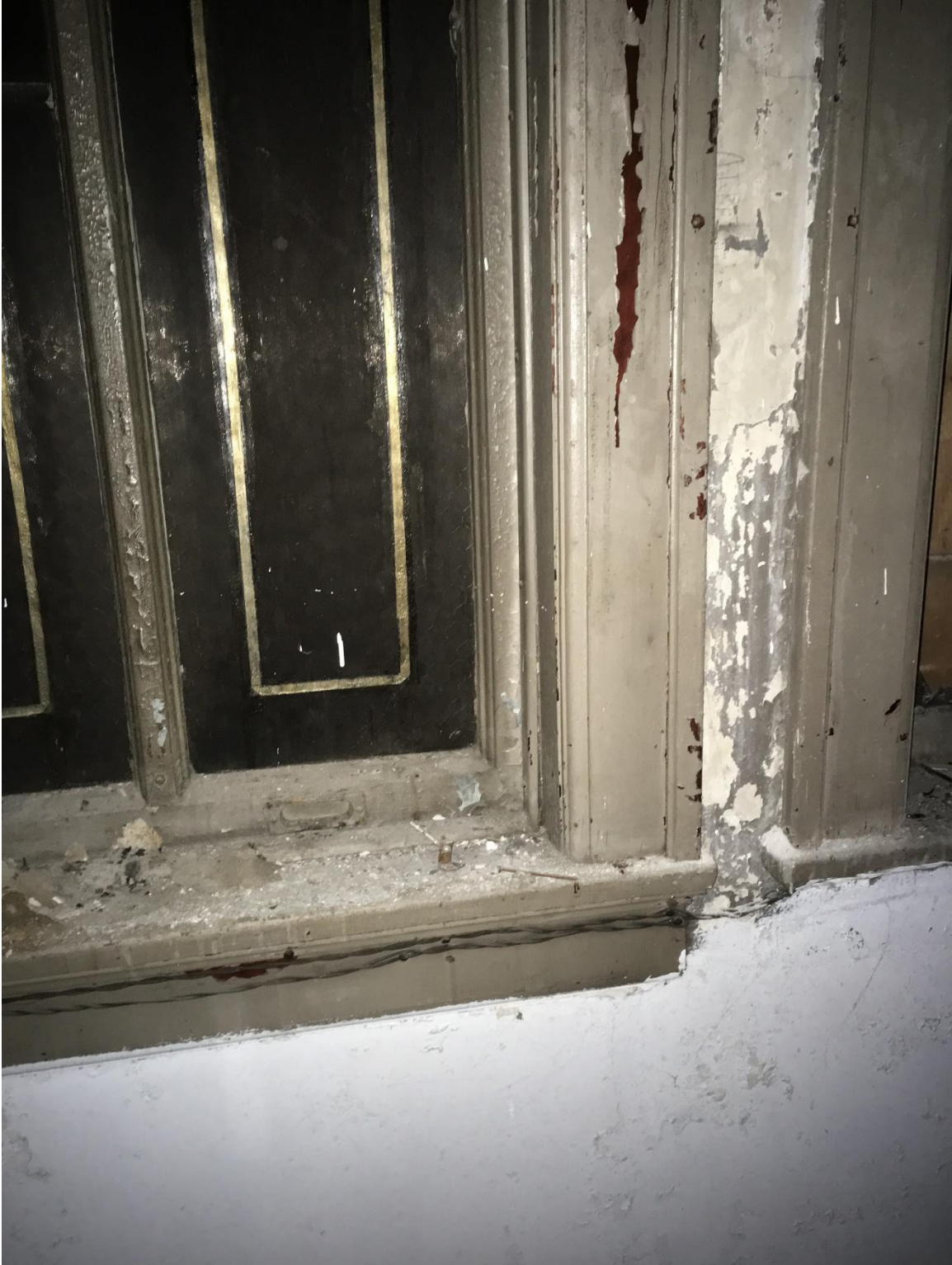
Figure #67: Interior, 3 rd floor, Window Detail. 5/31/19
