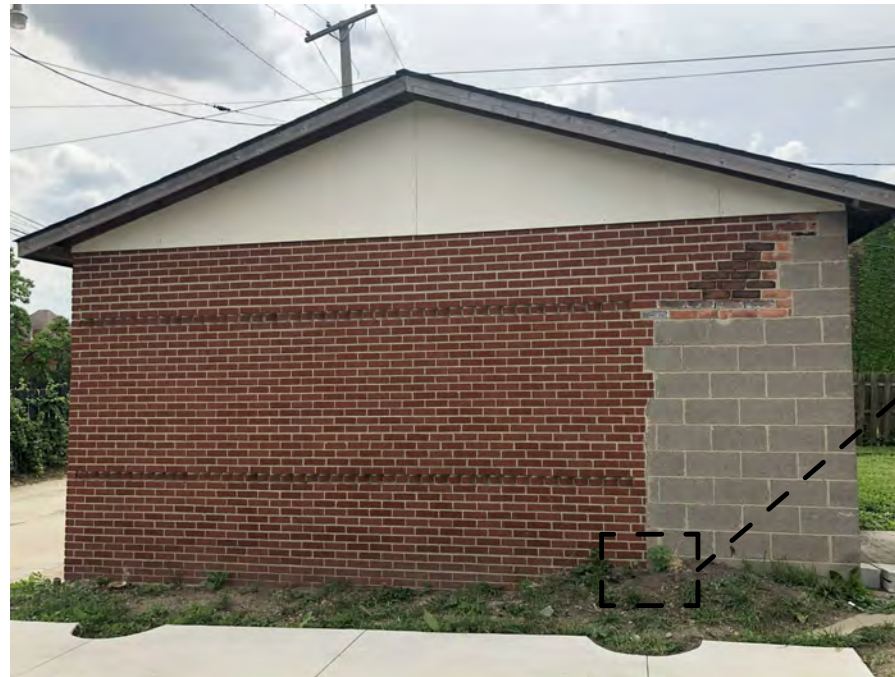
2. EXISTING CONDITIONS AT GARAGE (EAST FACADE)
