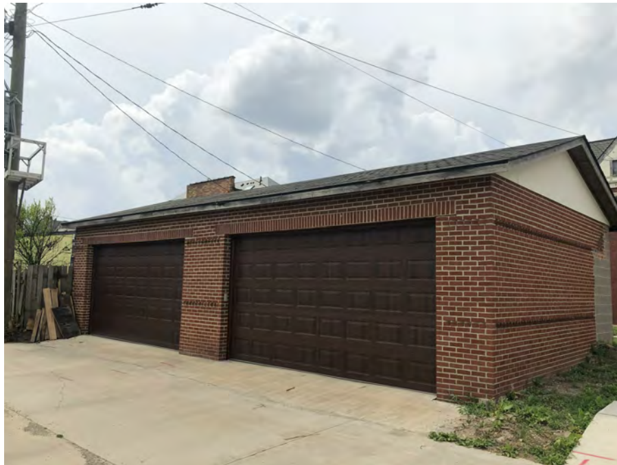
1. EXISTING CONDITIONS AT GARAGE (ALLEY FACADE)
