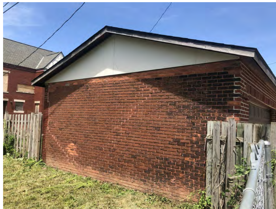
4. EXISTING CONDITIONS AT GARAGE (WEST FACADE)
