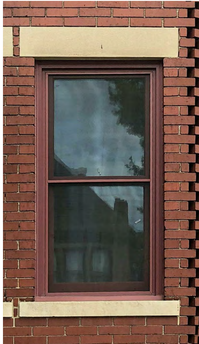
EXISTING CONDITIONS - REPLACEMENT WINDOW
