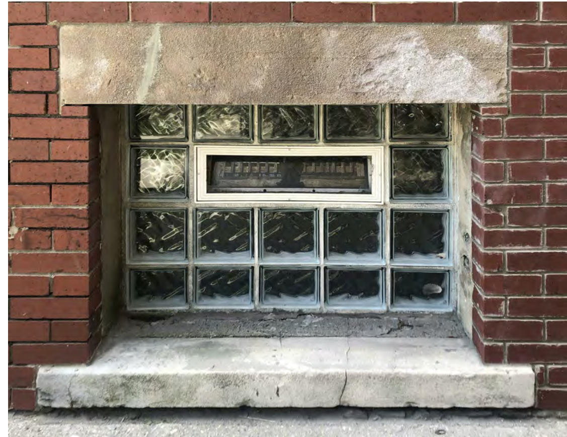
EXISTING CONDITION PHOTO - GLASS BLOCK W/ VENT
