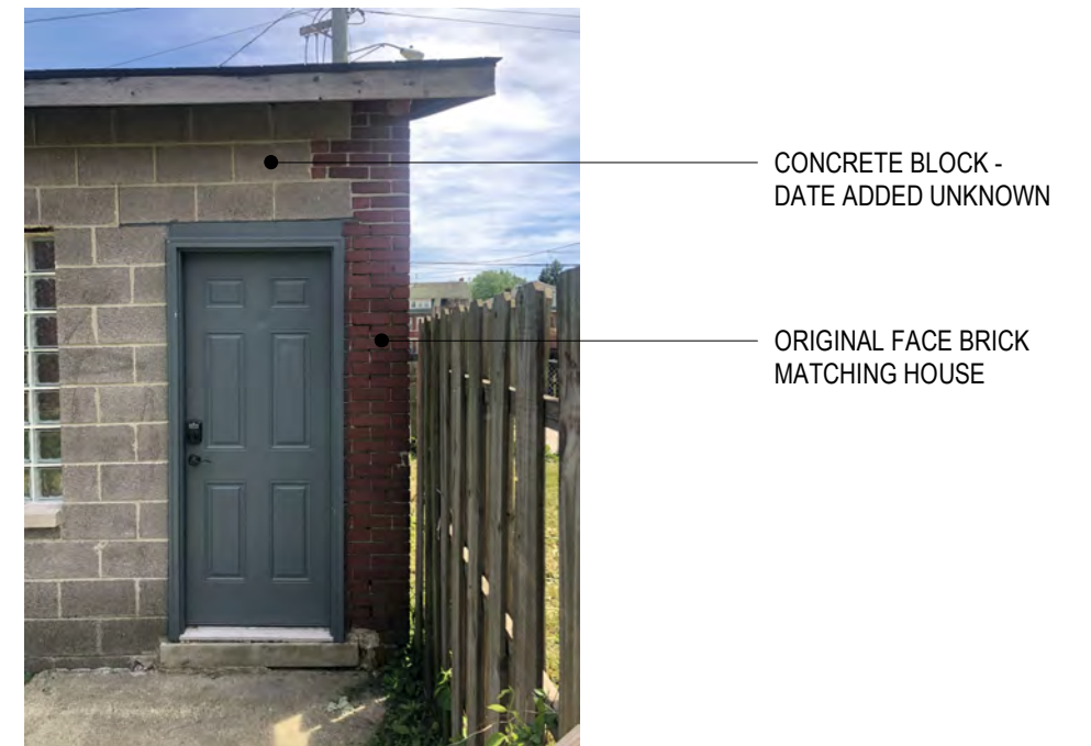
5. EXISTING CONDITIONS AT GARAGE (WEST FACADE)
