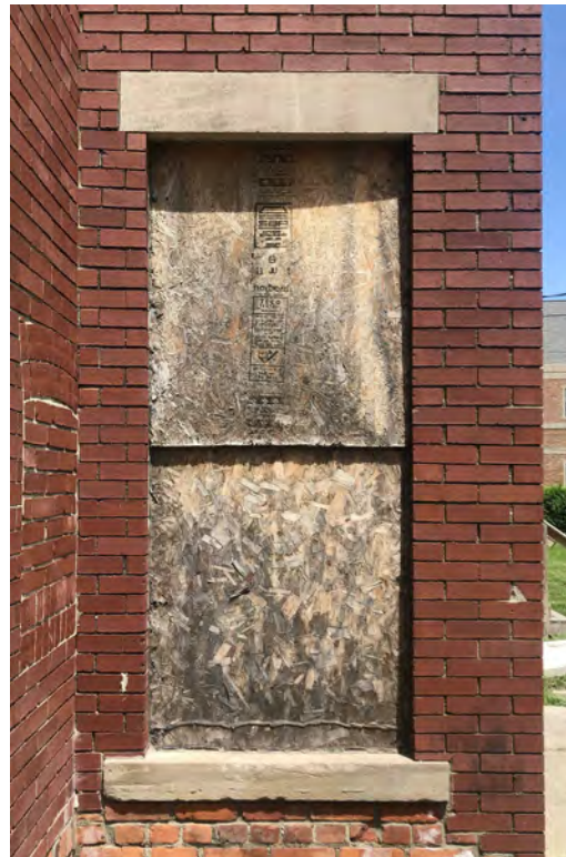
3. REAR DOOR - UNIT B (1ST FLOOR REAR)
