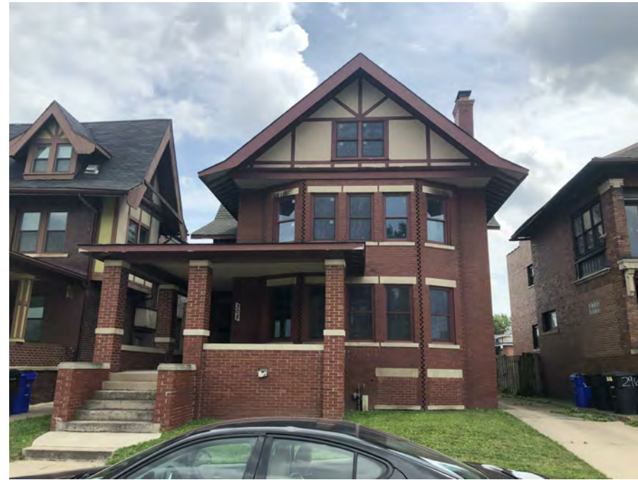
1. EXISTING CONDITIONS (NORTH ELEVATION)
