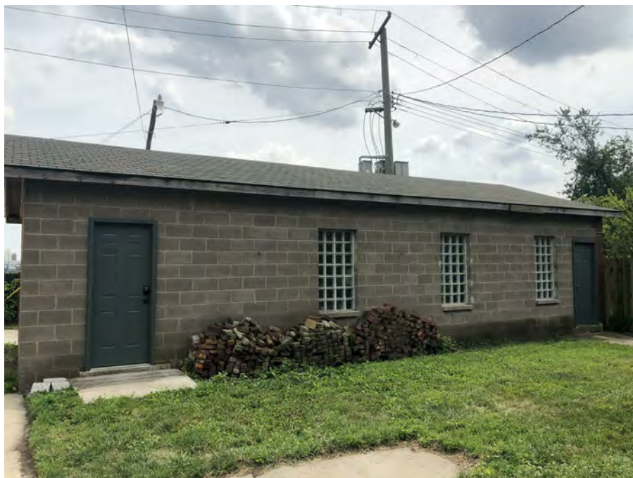
3. EXISTING CONDITIONS AT GARAGE (FACADE TOWARDS YARD)
