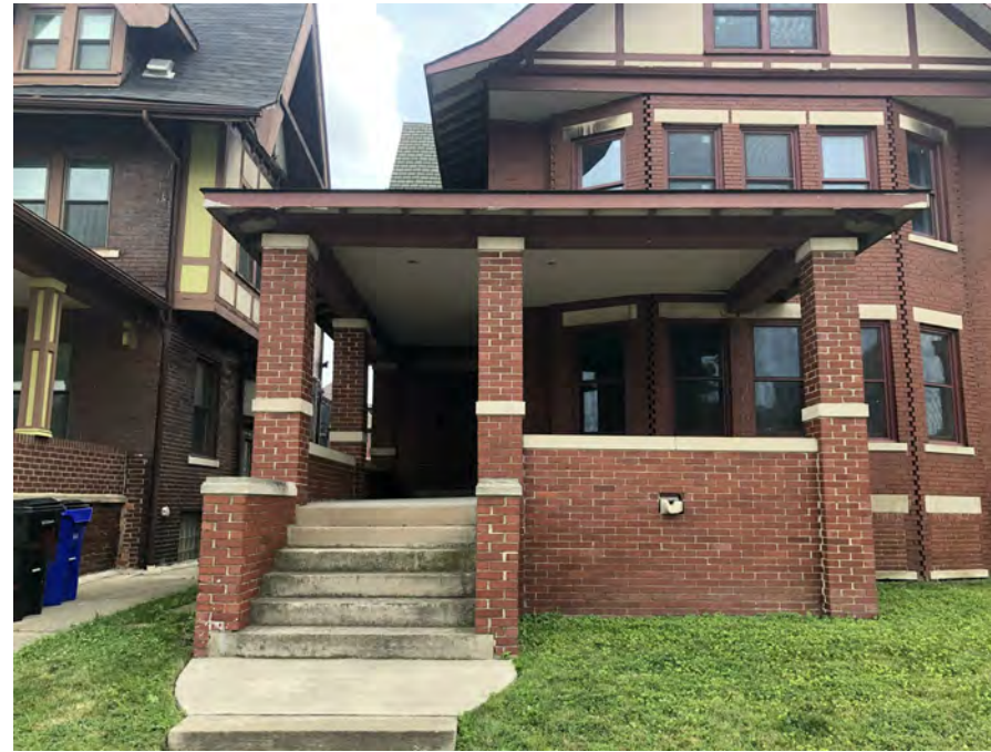
2. FRONT PORCH (NORTH ELEVATION)
