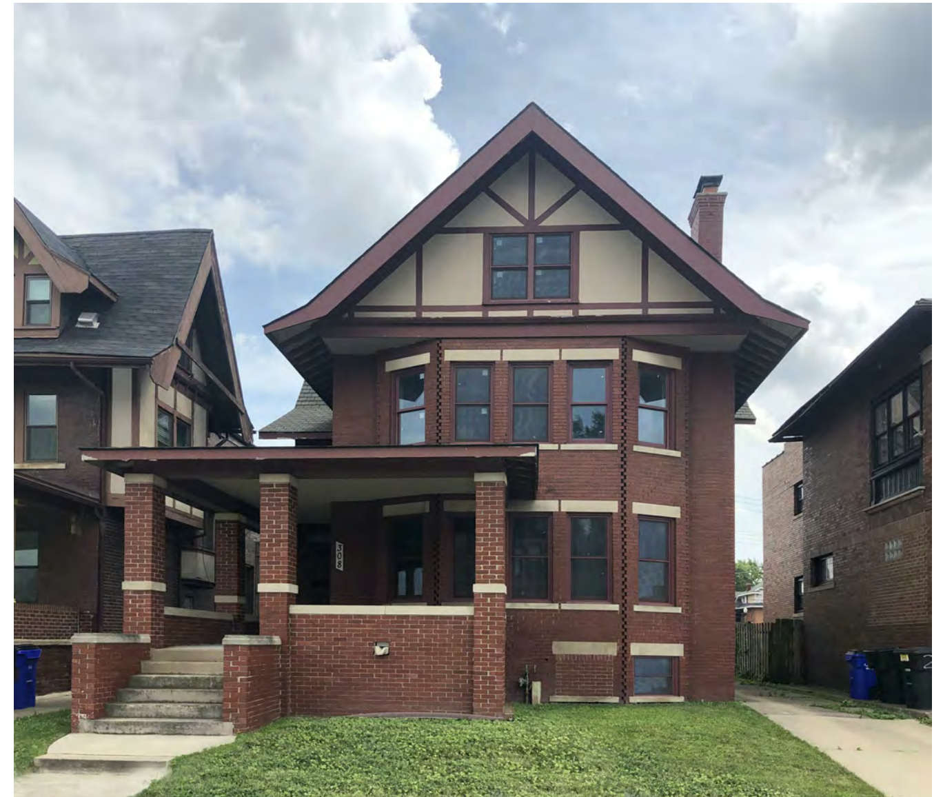
3. EXISTING CONDITIONS PHOTOGRAPH AT ELIOT STREET FACADE
