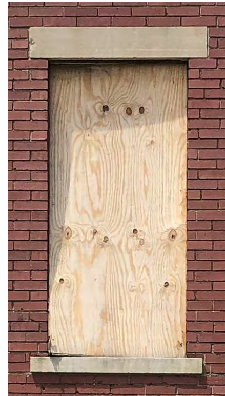
4. REAR DOOR - UNIT B (2ND FLOOR REAR)
