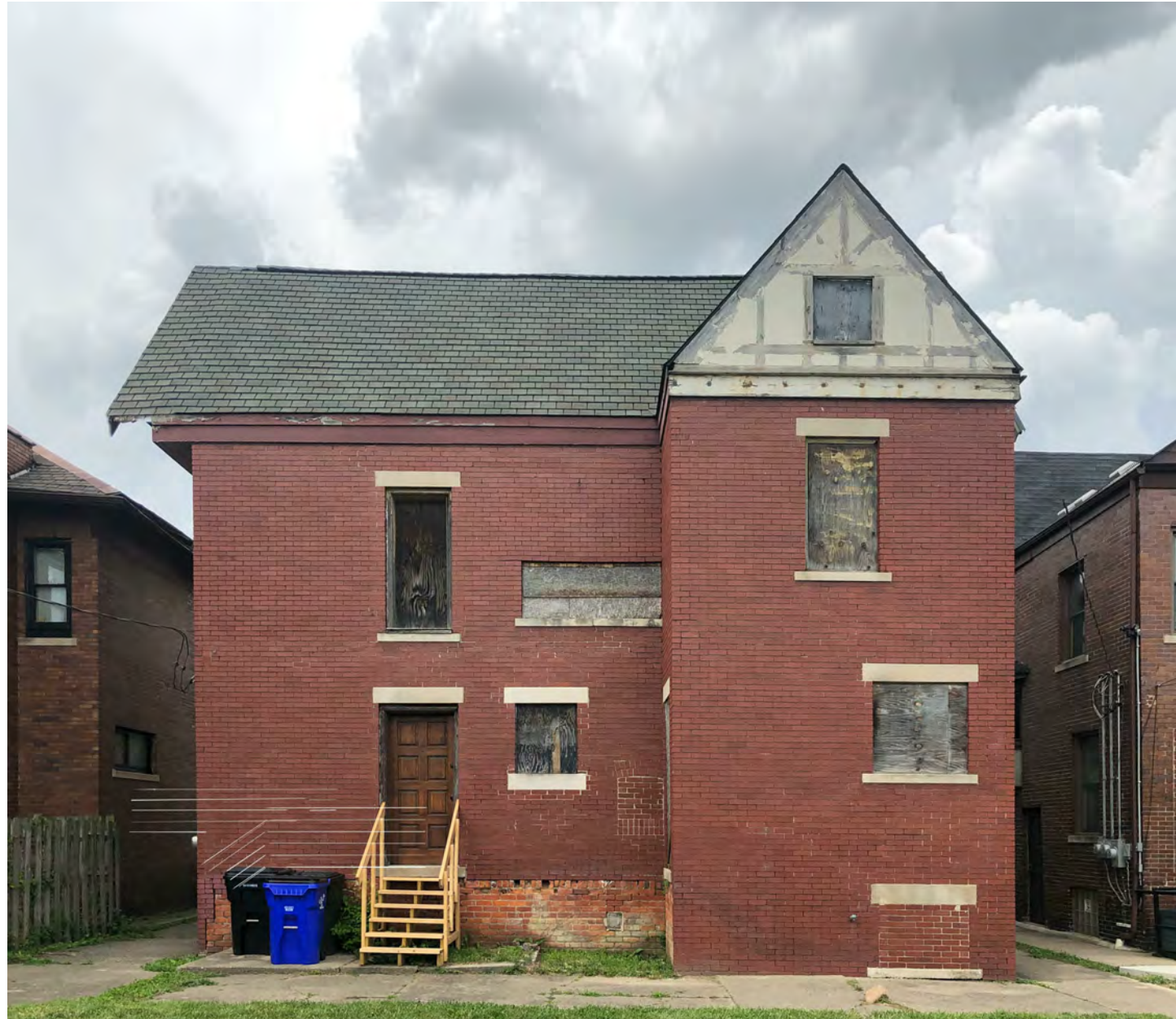
1. EXISTING PHOTOGRAPH AT REAR
