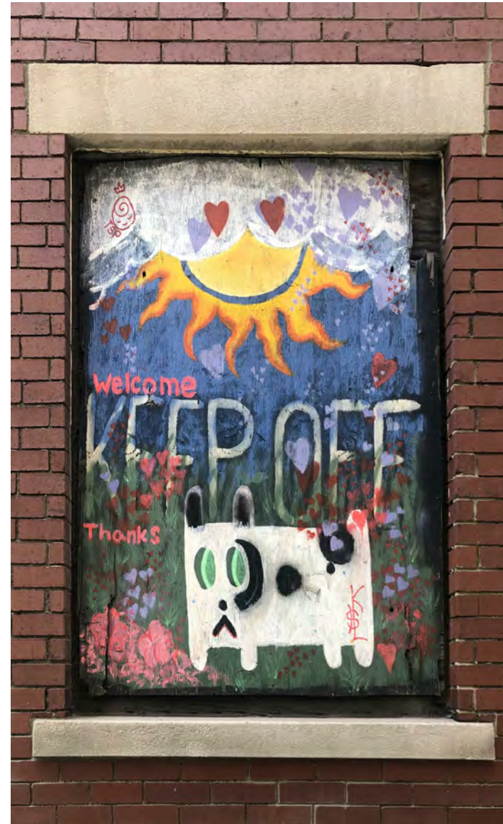
EXISTING CONDITIONS - PLYWOOD INFILL
