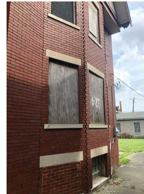
7. BAY WINDOWS (WEST ELEV.)
