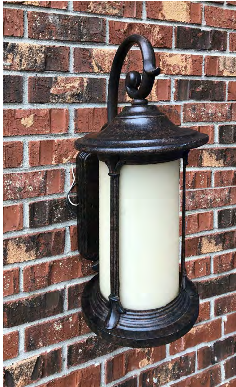
PORCH LIGHTS AT STREET FACADE (NORTH) DESCRIPTION: WALL-MOUNTED LAMP FINISH: OIL-RUBBED BRONZE
