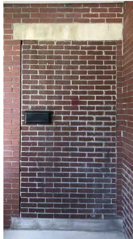
2. ENTRY DOOR - UNIT B (AT PORCH)
