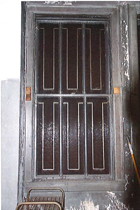
Interior of Steel Double Hung
