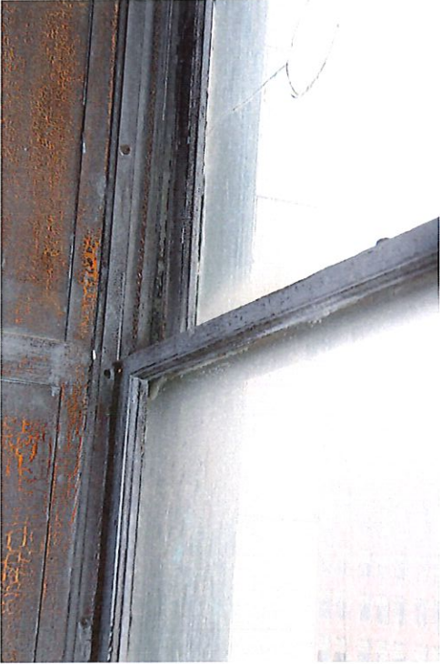
Interior Jamb Detail Wood Double Hung
